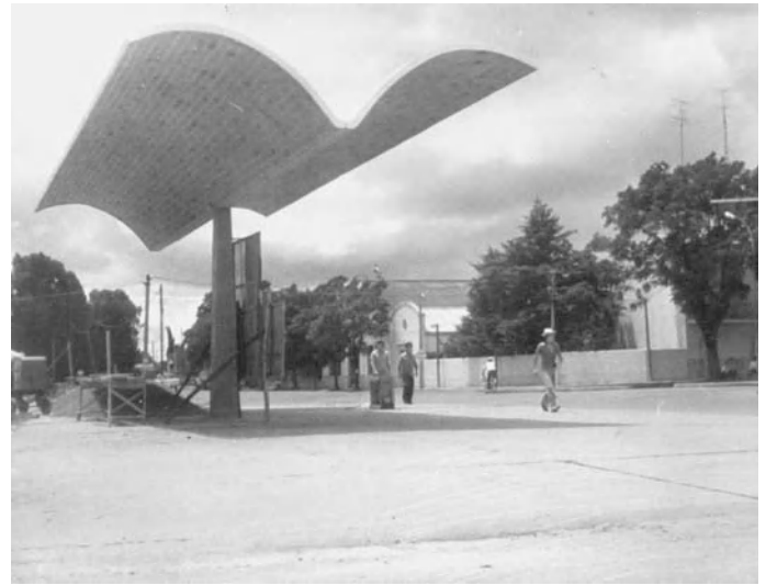
Reinforced Brick Self-Carrying Vaults of the Barbieri and Leggire Service Station Voûtes auto-porteuses en briques armées de la station service Barbieri et Leggire Estudio Dieste y Montañez Salto, Uruguay 1976
