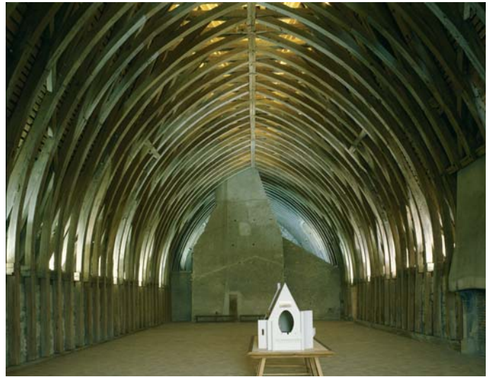
Roof Framing of the Sully-sur-Loire Château
