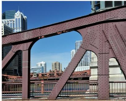
Figure 1.18 An old-fashioned riveted truss bridge ([pbase.com](http://pbase.com)).
