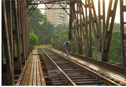
**Figure 1.7** An open-timber floor bridge ([123rf.com](http://123rf.com)).
