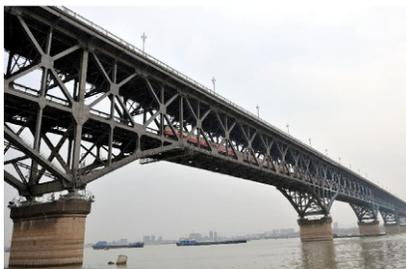
Figure 1.3 A combined highway-railway truss steel bridge ([chinatravelguide.com](http://chinatravelguide.com)).
