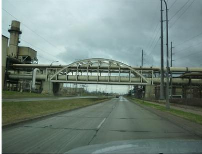
Figure 1.4 An arch steel bridge carrying pipelines ([civilinginphotos.blogspot.com](http://civilinginphotos.blogspot.com)).
