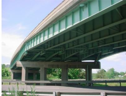
**Figure 1.10** A multiplate girder bridge ([haks.net](http://haks.net)).
