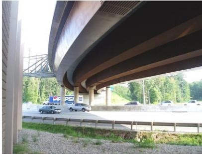
**Figure 1.11** A box girder bridge ([alviassociates.com](http://alviassociates.com)).
