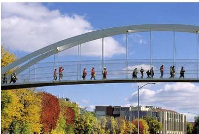
Figure 1.6 A pedestrian arch steel bridge ([photos.uc.wisc.edu](http://photos.uc.wisc.edu)).
