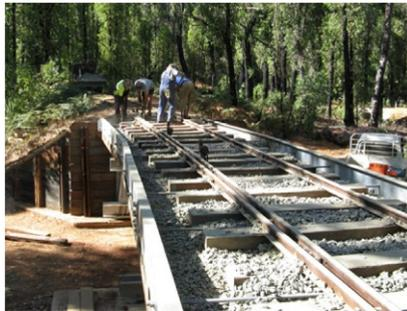
**Figure 1.8** A ballasted floor bridge ([hothamvalleyrailway.com](http://hothamvalleyrailway.com)).
