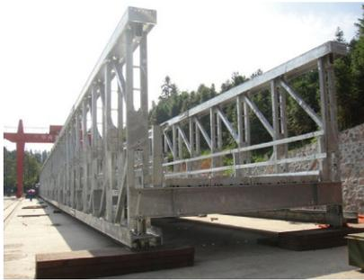
**Figure 1.16** A semi-through truss bridge under construction ([steel-trussbridge.com](http://steel-trussbridge.com)).
