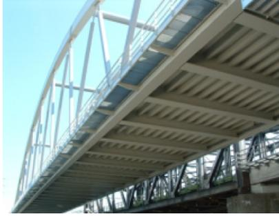
**Figure 1.15** An orthotropic steel floor truss bridge ([steelconstruction.info](http://steelconstruction.info)).
