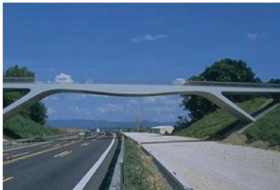
**Figure 1.12** A rigid-frame bridge ([en.structurae.de](http://en.structurae.de)).
