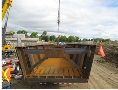
**Figure 1.9** A steel-concrete composite box girder bridge under construction ([mto.gov.on.ca](http://mto.gov.on.ca)).
