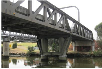
Figure 1.17 A pony truss bridge ([bphod.com](http://bphod.com)).
