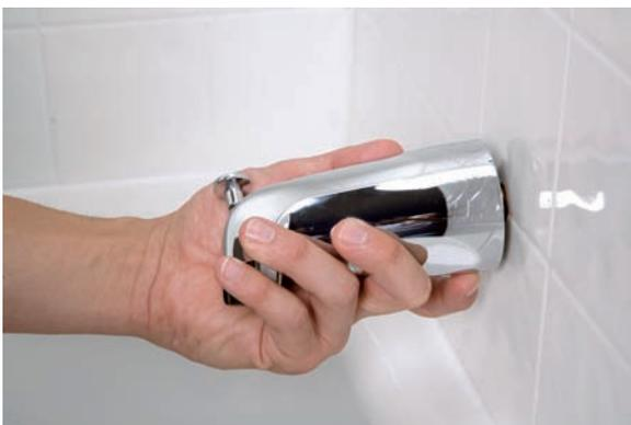
4. Screw the new spout onto the threaded supply pipe by hand until it's snug.
