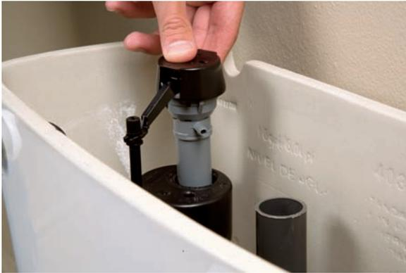
9. Insert the fill valve into the tank, placing the valve's threaded tail piece through the hole in the bottom of the tank.
