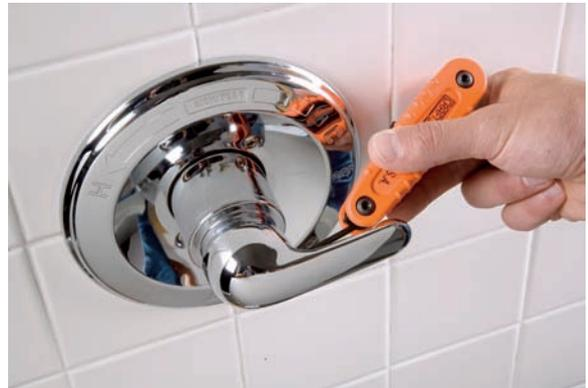
3. Loosen the escutcheon plate by unscrewing the three screws (the common configuration on most models).
