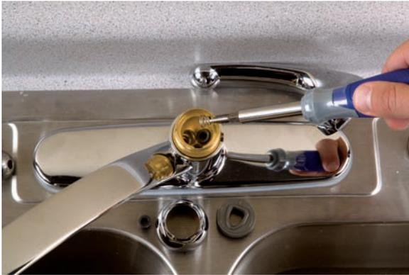
7. Insert the tip of the screwdriver into each spring in the faucet body to remove them. You may need to twist the springs back and forth slightly to break them loose.
