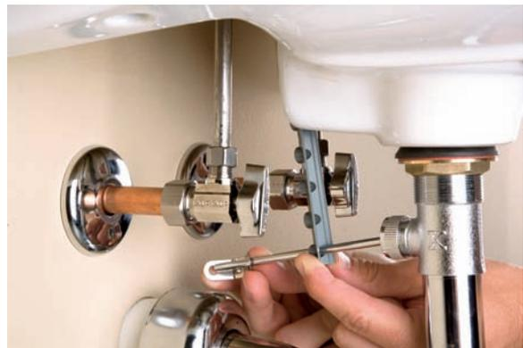
12. Test the plunger. The drain should be open when you push down (top photo) and closed when you pull up (bottom photo).
