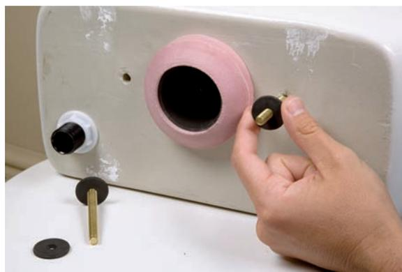
8. Replace the tank on the bowl. Alternating side to side, tighten the bolts and nuts (using the screwdriver and adjustable wrench, as in Step 2) until the gaskets look like they're seated. Then tighten each tank bolt nut another quarter turn.
