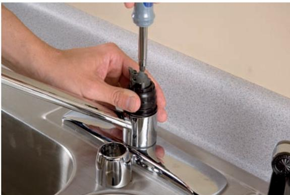
3. Use a screwdriver to remove the retaining nut under the handle.
