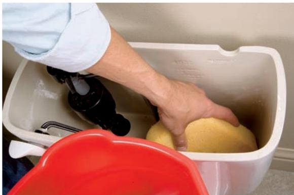
2. Drain the tank by flushing the toilet, and use a sponge to soak up any excess water in the tank.
