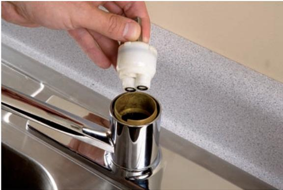
5. Lift off the cartridge. You can usually do this by hand. Use groove-joint pliers if the cartridge sticks.
