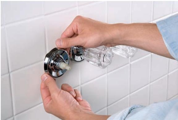
4. Remove the escutcheon plate behind the handle body. It should slide right off.
