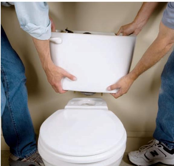
6. Lift the tank straight up off of the tail section of the bowl. Turn the tank over onto the towels on the floor.
