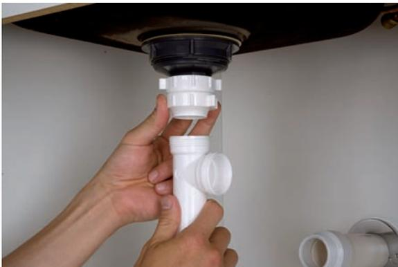
3. Connect the tail piece, whose length is determined by the position of the drain line coming out of the wall. The tail piece should come to the bottom edge of the wall drain line. You can eyeball this length and cut the tail piece later if it's too long.
