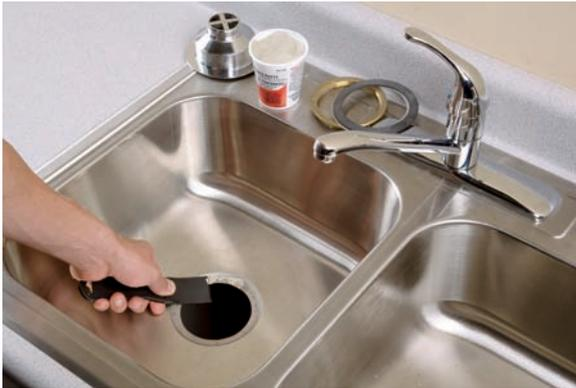
3. Scrape off any old plumber's putty on the upper side of the sink with a plastic putty knife. *Don't* use a metal putty knife or you'll damage the sink's finish! If you plan to reuse the old basket, scrape off any old putty under the basket flange.
