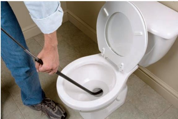
2. Crank the auger handle clockwise to snag or grab the obstruction. Continue cranking while pulling the auger cable (and the obstruction) out of the toilet.
