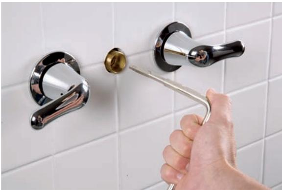
10. If a new washer doesn't stop the leak, then you need to replace the seat. Use a seat wrench to remove the old seat.
