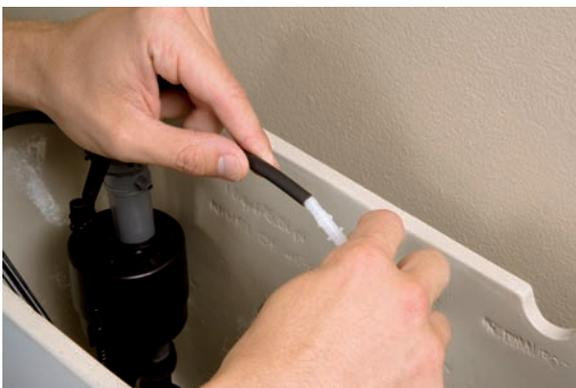
12. Attach the refill tube and adaptor to the overflow valve.
