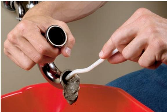
3. Check to see if the clog is in the trap itself. If so, force the clog out (using an old toothbrush if needed) and reassemble the trap.
