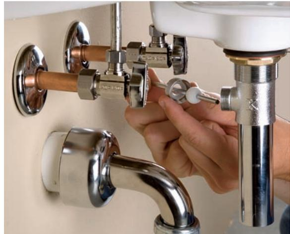
11. Secure the lift rod extension to the pivot ball rod by sliding the pivot ball rod into one of the holes in the lift rod extension and securing with the retaining clip. You may need to select a different hole if you can't fully open or close the plunger.
