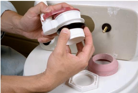
9. Install the beveled cone washer onto the tail piece of the new flush valve. The beveled side should face the end of the tail piece. Reinstall the flush valve in the tank.
