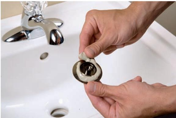
2. Craft a snake of plumber's putty that's about the same size in diameter as the width of the drain flange. (It's better to have too much putty than not enough; you can scrape away any excess when everything is tightened.) Press the putty snake around the underside of the drain flange and set aside.
