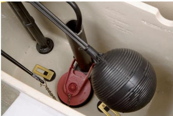
6. Adjust the chain length as needed so that there's about  $\frac{1}{2}$  inch of slack in the chain.
