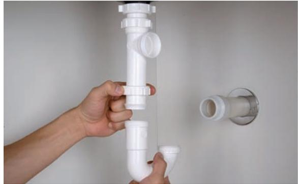
5. Position the trap arm on the P-trap, and mark where to cut the arm so that it fits in the wall drain line. Remove the arm and cut it to length using a PVC tube cutter or hacksaw.
