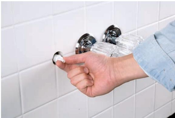
7. Remove the cartridge. It should come out by hand.
