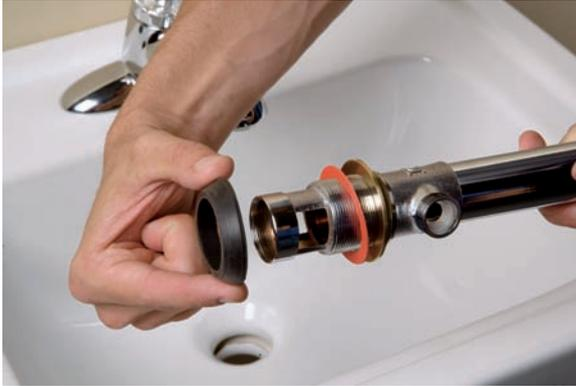
4. Slide the beveled or cone-shaped gasket onto the drain tail piece and thread the lock-nut onto the drain body.
