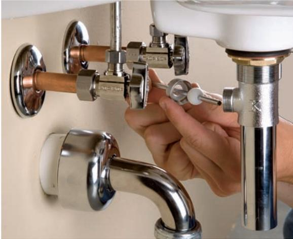
**If water leaks from the pivot ball connection:** Unscrew the pivot ball retaining nut with groove-joint pliers, and remove the rod, ball, and gasket. Replace the gasket, and reassemble the connection.
