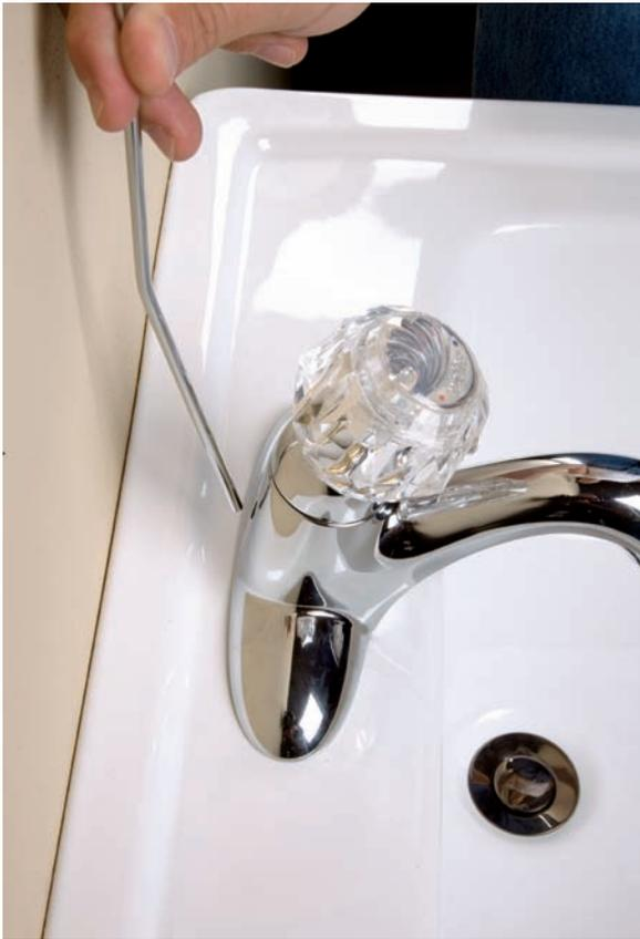
7. Insert the drain plunger lift rod completely through the hole in the top of the faucet. You can adjust the lift height of the rod later.
