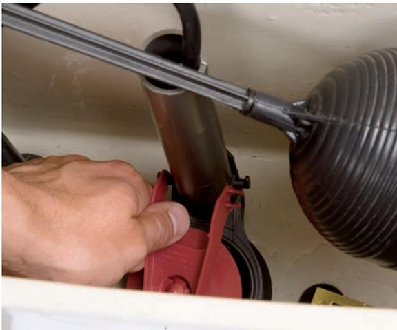
4. Line up the new flapper with the flush valve opening, and slip the flapper tabs over the flush valve ears. The new flapper lift point should be aligned with the flush lift arm.
