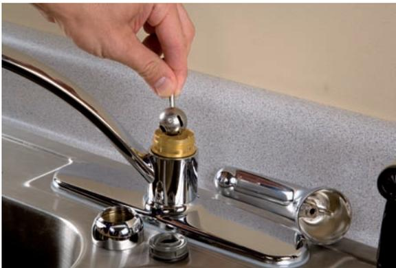
5. Lift out the ball. Inspect each part for damage and replace them with parts from the kit as needed.
