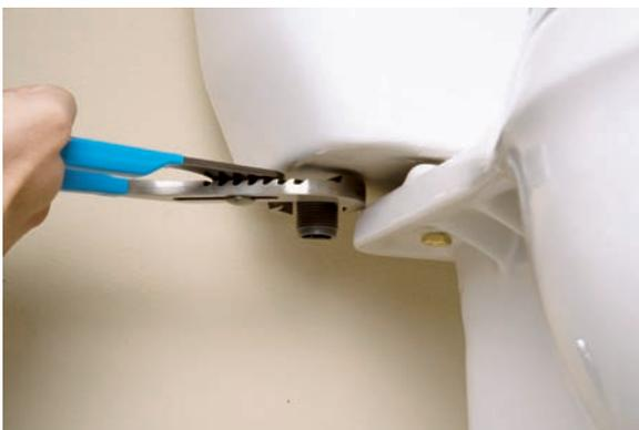
5. Loosen and remove the nut on the bottom of the fill valve; it's located on the bottom of the outside of the tank where you find the water supply feed. Leave the bucket under the fill valve to catch any water that may run out when you loosen the nut.
