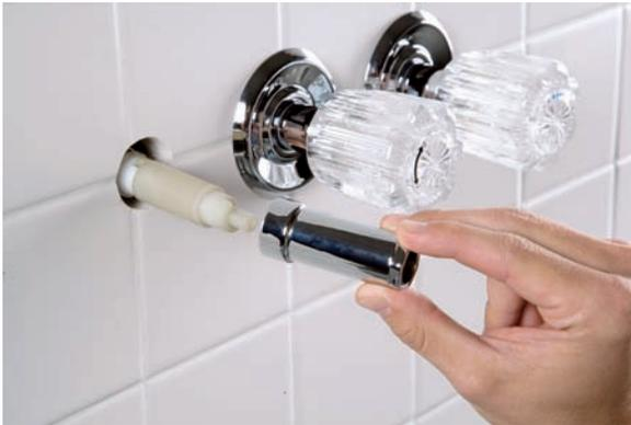
**16.** Slide the metal cover back onto the faucet body and hand-tighten it. Place the escutcheon plate over the metal faucet body.
