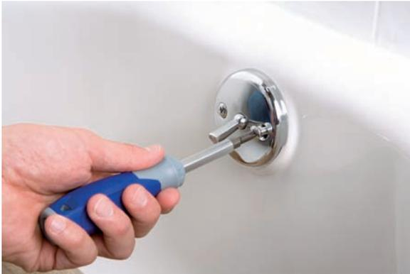
**Clearing a tub drain with an auger through the drain assembly:**
