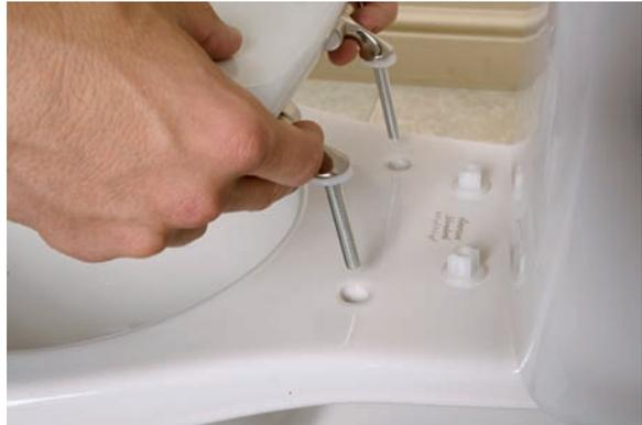
4. Center the seat over the bowl opening and tighten the nuts using an adjustable wrench. Don't overtighten the nuts — just beyond snug is good enough.
