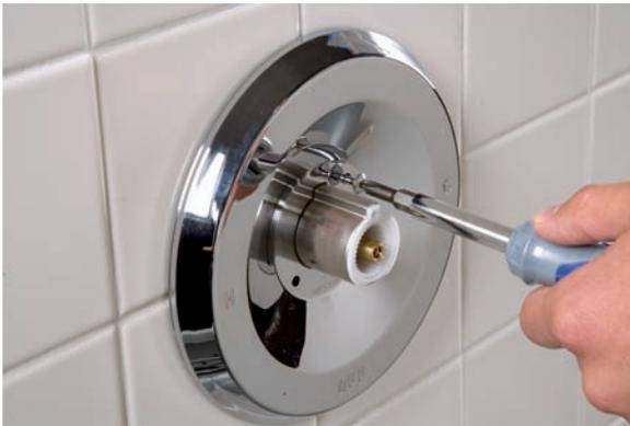
4. Remove the screws holding the escutcheon.
