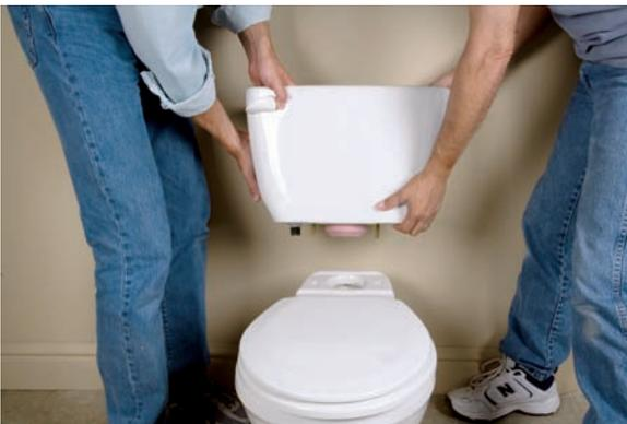
**13.** Reinstall the toilet tank with your helper and reconnect all of the parts by reversing Steps 1 through 5.
