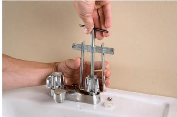
3. Remove the retaining nut using groove-joint pliers.
