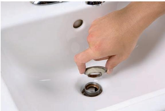
6. Thread the flange ring from Step 2 onto the drain body from above. Scrape off any excess plumber's putty using a plastic putty knife.
