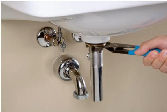
9. Use groove-joint pliers to tighten the locknut until it feels snug.
