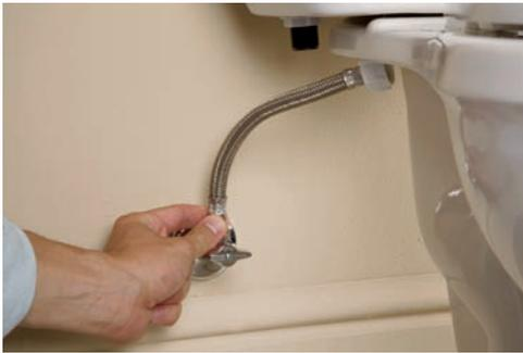
4. Drain the tank by flushing the toilet, and use a sponge to soak up any standing water in the tank. Place a bucket under the toilet tank and remove the supply tube, which is connected to the shutoff valve and fill valve.
