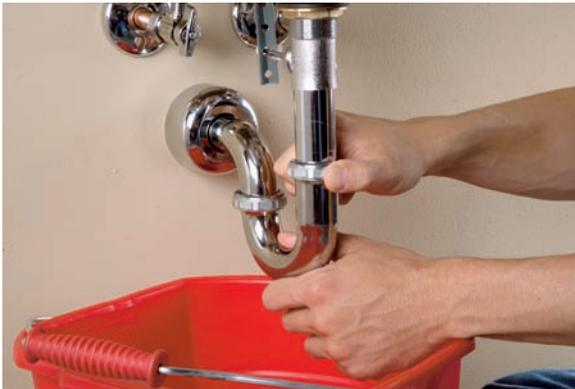
5. Secure the new trap to the drain lines with the slip nuts. Hand-tighten the nuts.
