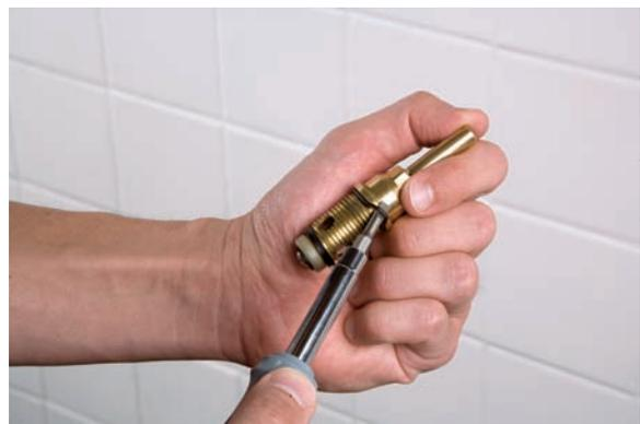
9. With your fingertip, rub silicone grease on the new O-ring and insert it on the stem.
