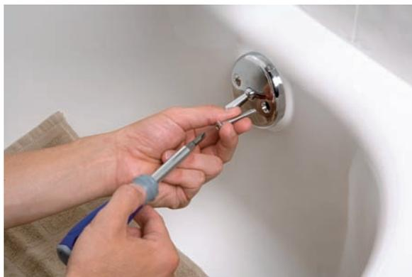
6. Tighten the screws on the coverplate. If the drain still won't hold water, repeat the process starting at Step 1.
