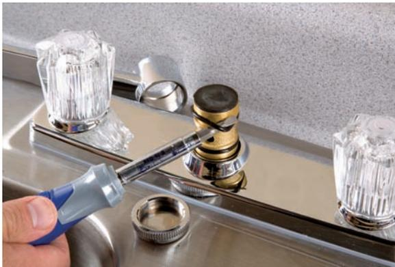
3. Use a screwdriver to pry the O-rings from the groove in the faucet body.
