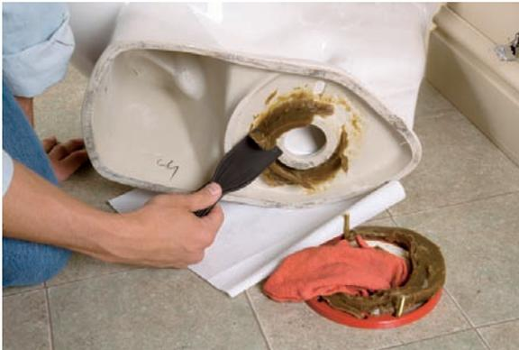
5. Place the bowl on its side on an old towel (to catch any water that may be in the trap). Don't remove the flange bolts unless they're damaged and need to be replaced. If they need replacing, do it now.
