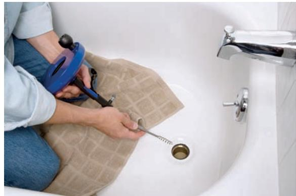
4. Keep pushing the auger cable into the drain until you can't move the cable in any farther. Leave about 6 inches of excess cable coming out of the shower drain.
