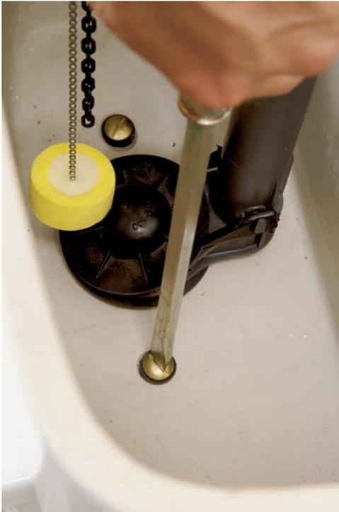
2. Unscrew the tank bolts with an adjustable wrench and screwdriver. You have to use the adjustable wrench to hold the nut located on the underside of the tank bolt, and then use the screwdriver to loosen the tank bolt inside the tank.
