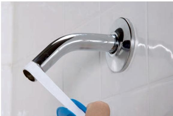
2. Clean the threads of the shower arm with an old toothbrush and then wrap the pipe threads with two or three turns of pipe-thread (Teflon) tape. Wrap the tape in a clockwise direction to keep it from unwrapping when you attach the new showerhead.
