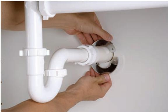
11. Install an escutcheon plate to cover the gap between the wall drain line and the wall. This not only adds a finished look but also seals drafts and keeps out insects. There are two types of plates: A split-ring plate fits around the pipe that's already installed, and a solid-ring plate slips over the pipe before you connect the trap arm to the wall drain line. (In this project, you'd put a solid-ring plate on before Step 7.)
