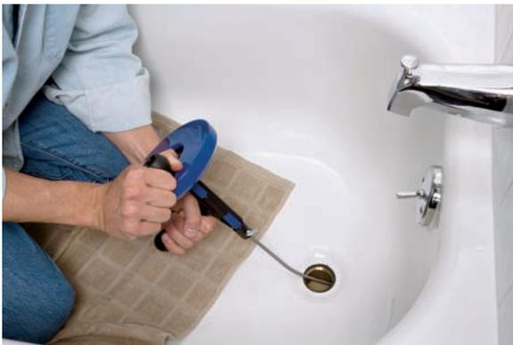
5. Tighten the auger screw and then turn the auger handle clockwise. Put pressure on the cable as you turn the handle in order to snag or loosen the clog to send it down the drain.
