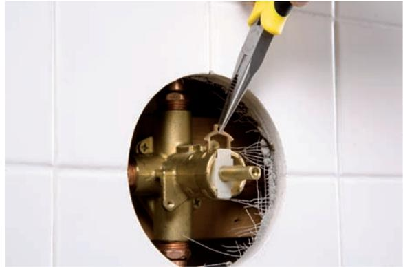
7. Pull the old cartridge out; try pulling it out by hand first, especially if you plan to reuse it (you don't want to damage the stem by pulling it out with pliers).
