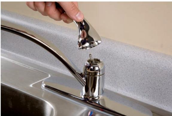
3. Lift off the handle and unscrew the cap located under the handle.
