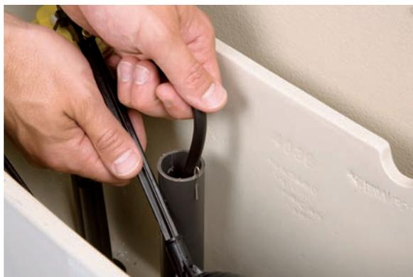
4. Disconnect the rubber fill tube from the fill valve that's connected to the flush valve's overflow tube.
