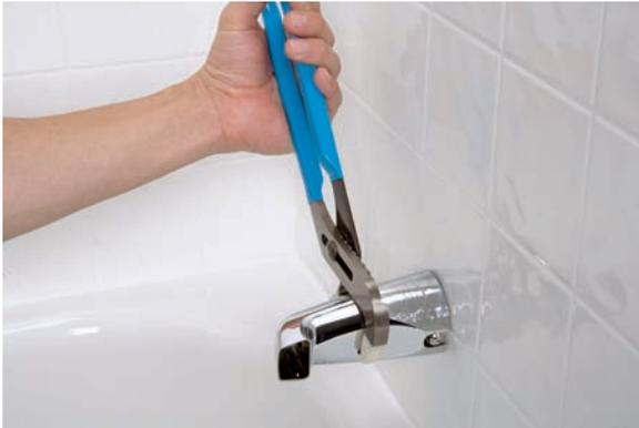
2. Use groove-joint pliers to turn the old spout counterclockwise to unscrew it from the threaded supply pipe. (Don't worry about wrapping the old spout to prevent damage before using the pliers — you're throwing the old spout away.)
