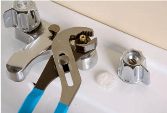
4. Grab the stem with the pliers, and pull it straight up and out of the faucet housing.
