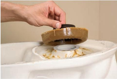
7. Turn the bowl upside down on the towel. Place the new wax ring (with flange) over the drain horn of the toilet.
