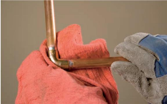
10. Wipe away the excess solder using a rag. The pipe will be hot, so be careful when touching the rag to it!
