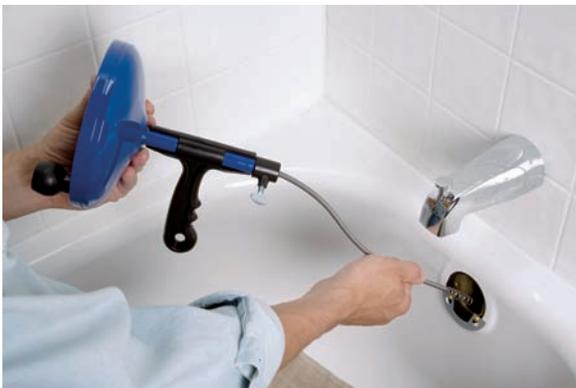
3. Push the auger cable into the opening until you feel resistance. Leave about 6 inches of extra cable out of the opening and tighten the auger screw.
