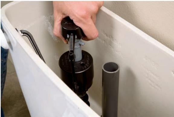
7. Determine the height of the replacement fill valve so that the markings near the valve's top assembly are at least 1 inch above the top of the overflow tube.
