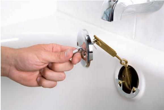
2. Carefully pull the coverplate, linkage, and plunger from the overflow drain opening.
