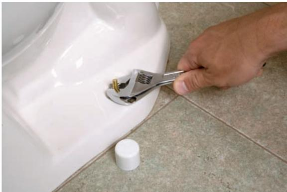
3. Loosen the toilet bowl nuts (which connect the toilet base to the floor) with an adjustable wrench, and remove the nuts.
