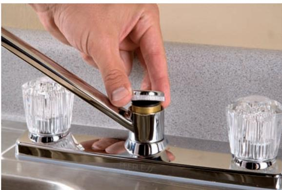
7. Reinstall the spout cap. First tighten it by hand and then use pliers or a strap wrench to complete the job.
