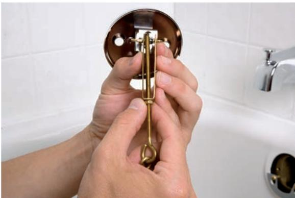
4. Screw the rod down about  $\frac{1}{8}$  inch and tighten the locknut.
