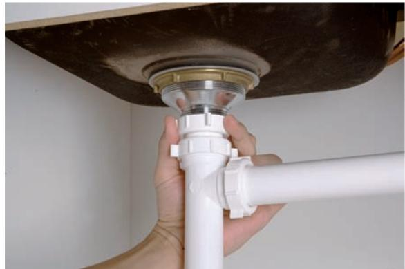
8. Test the drain with running water. If you spot leaks, tighten the nut slightly, but no more than one-quarter turn.
