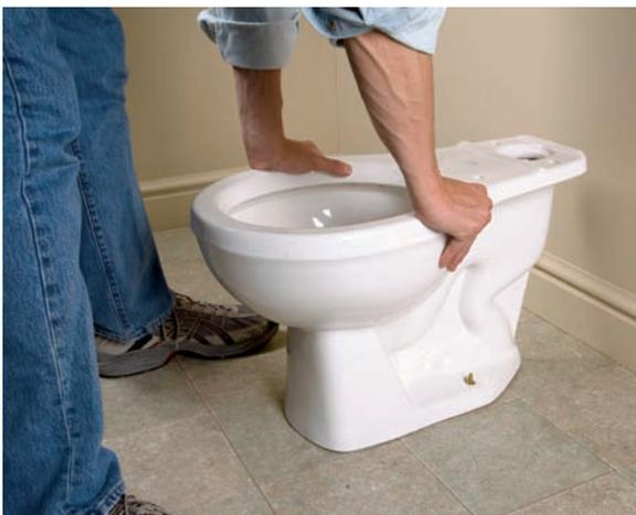
9. Lift the toilet base, and slowly set it down over the flange bolts. Press down evenly on the base to compress the wax ring and properly seat the base.
