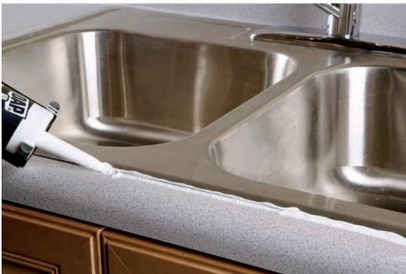
3. Apply steady pressure to the trigger on the caulk gun to apply a bead of caulk along the joint between the sink and the countertop. Take your time when working along the back edge of the sink and around the faucet.
