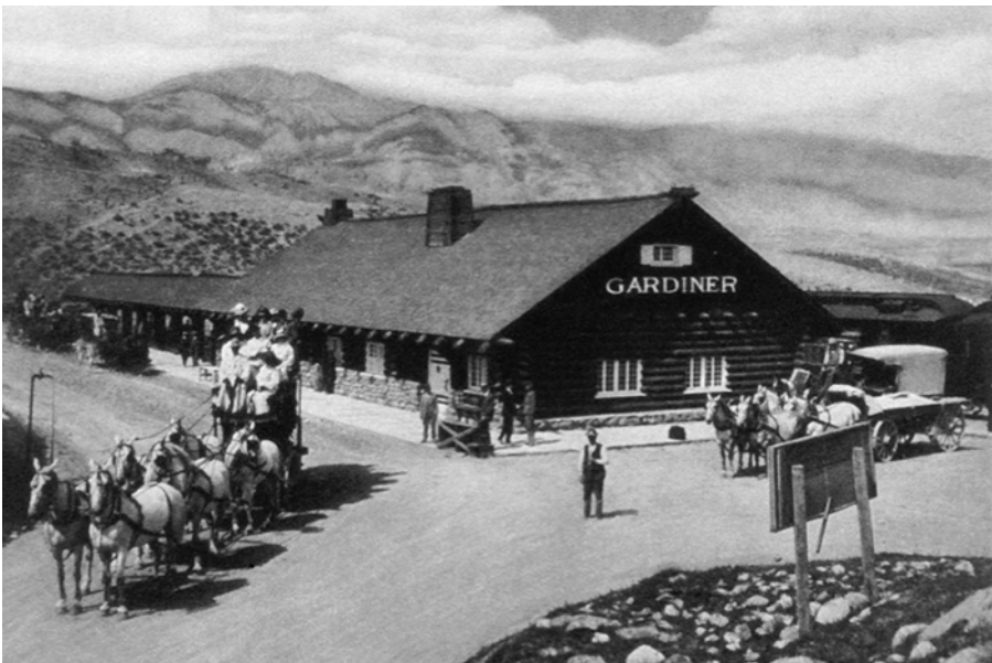
2.20 Disembararking at the Gardiner train station at the north entrance to the Park.
