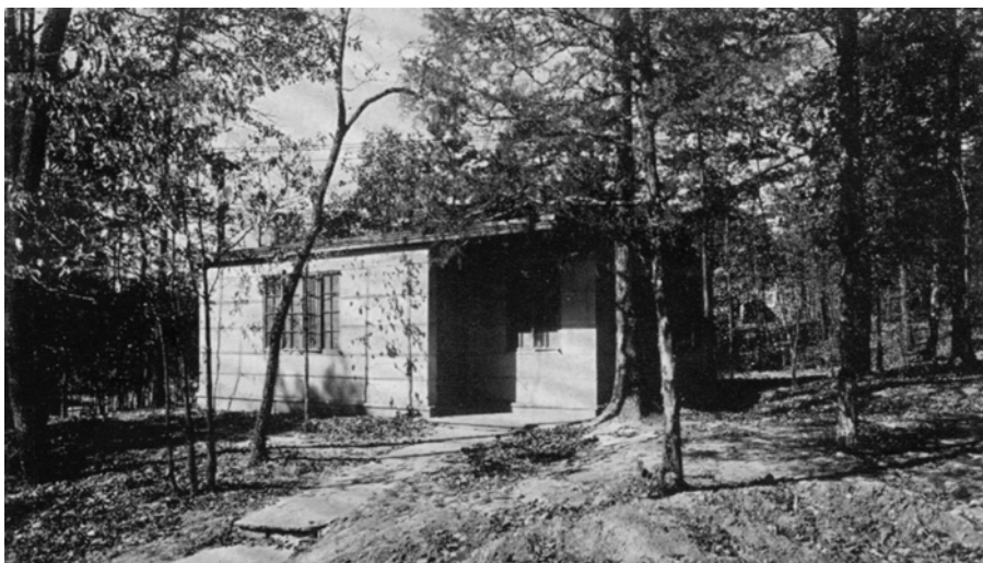
3.40 Steel frame house, Norris.
