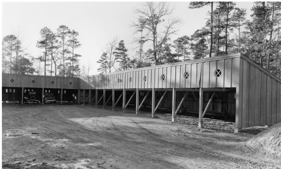
3.37 Collective parking garages in Norris, 1934.
