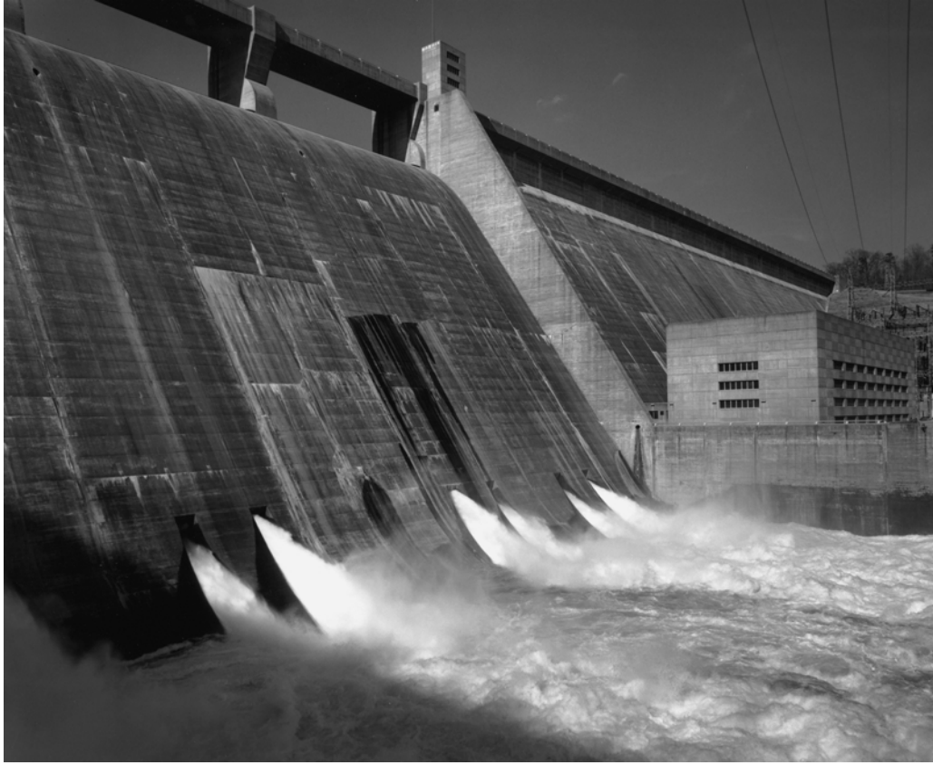
3.18 View of Norris from below.
