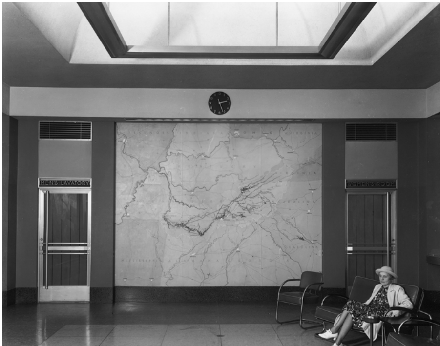
3.16 Visitors' lobby in the Norris Dam powerhouse.
