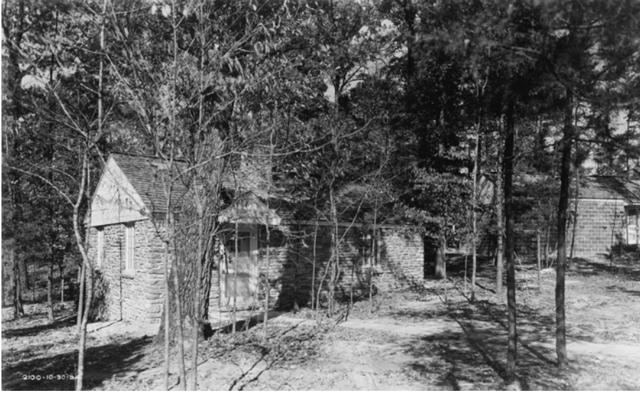
3.36 Stone house in Norris, 1934.
