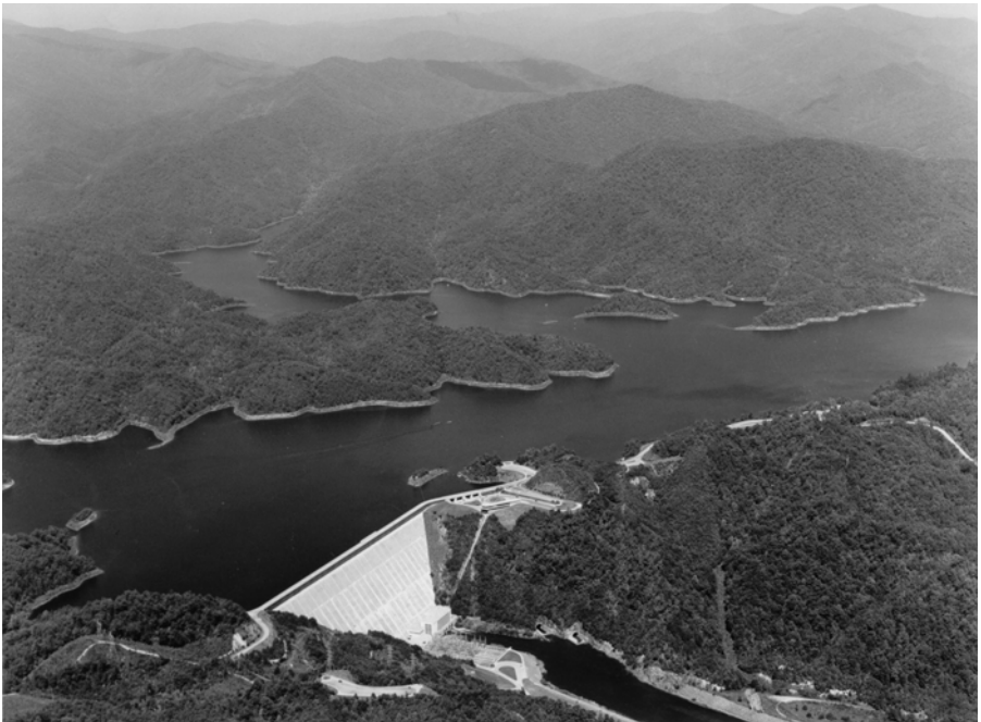
3.48 Aerial view of Fontana Dam.
