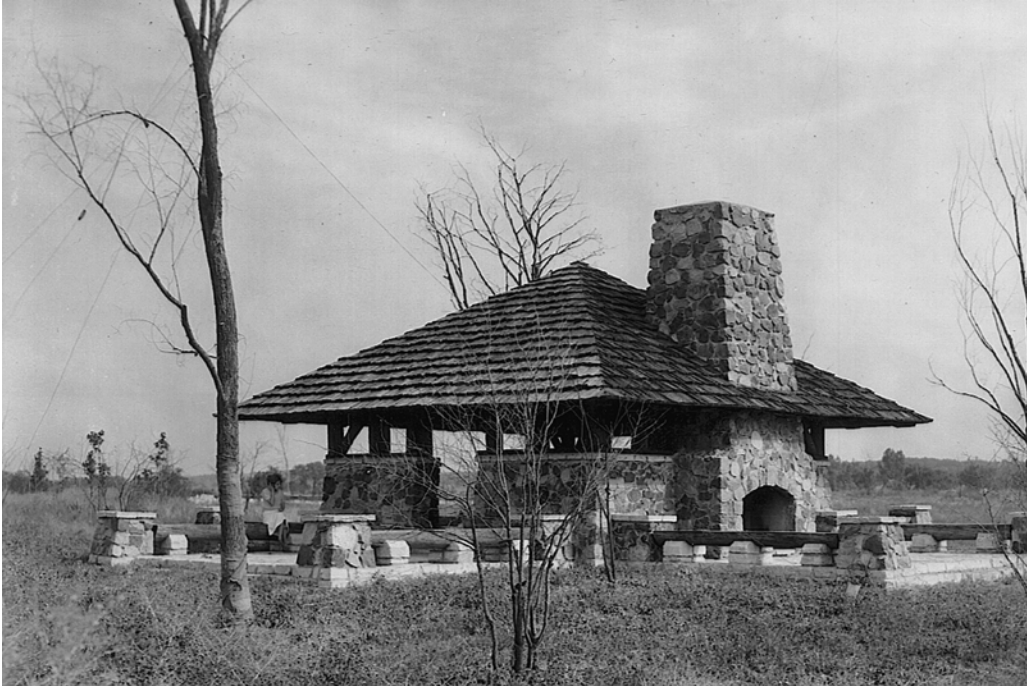
2.28 Picnic shelter in I&M Canal State Park, Marseilles, Illinois.
