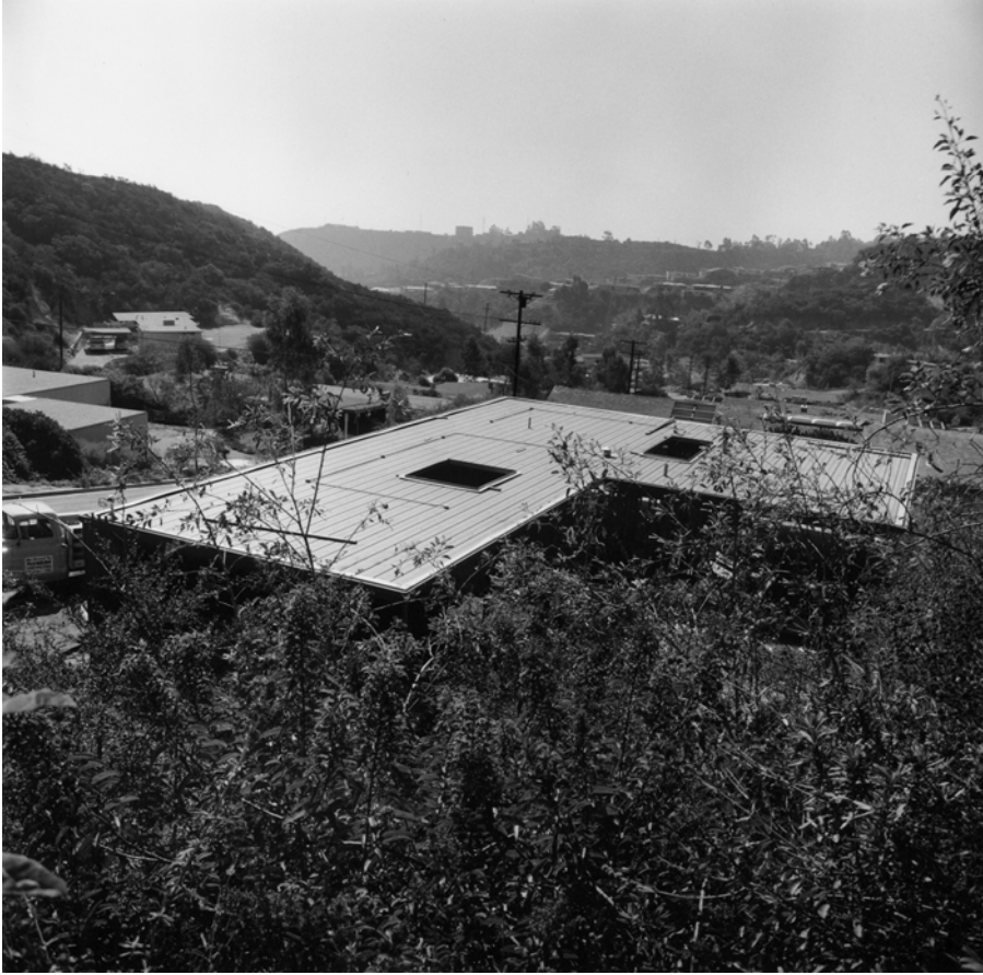
4.29 View of CSH 21 from neighbor uphill.
