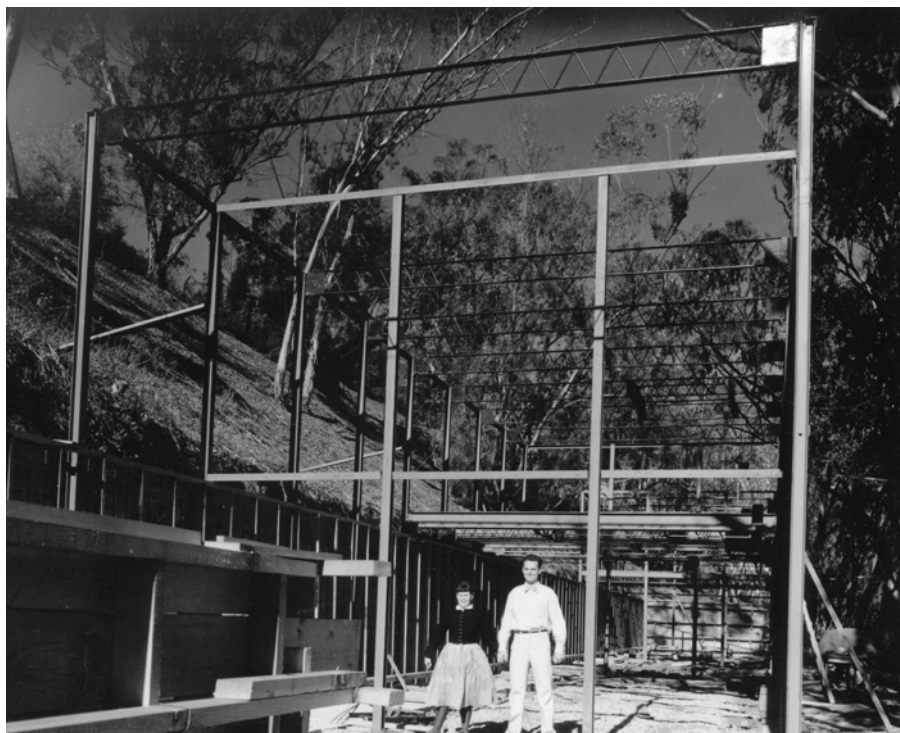
4.25 Charles and Ray Eames during construction of their house, 1949.
