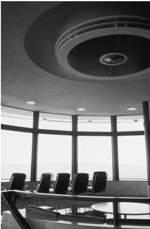
3.46 Ceiling of visitor center, Watts Bar Dam.
