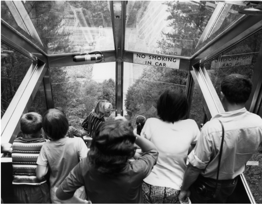
3.50 View from inside Fontana incline car.
