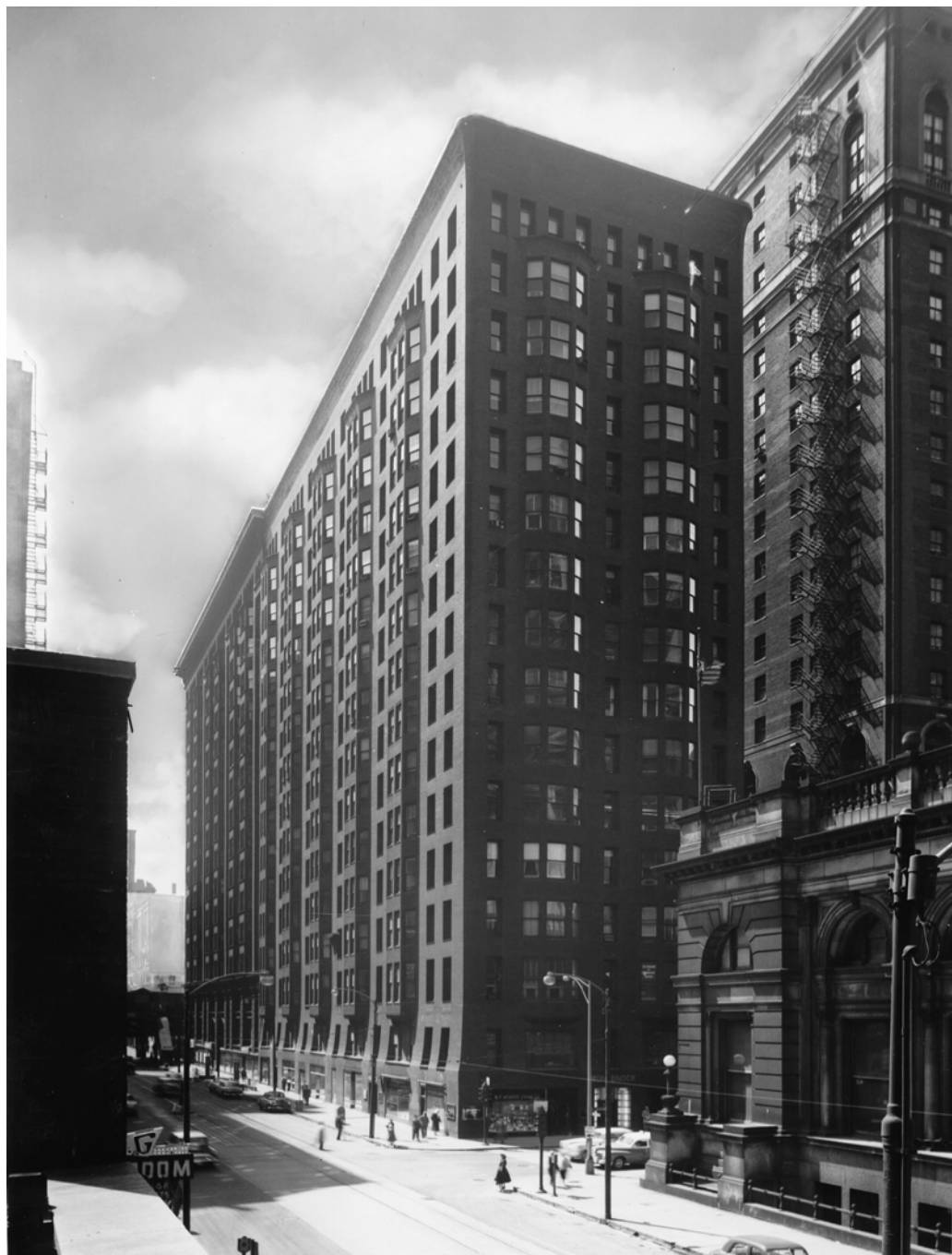
1.2 The "Monadnock" block, Chicago, 1891. Architects Burnham & Root.
