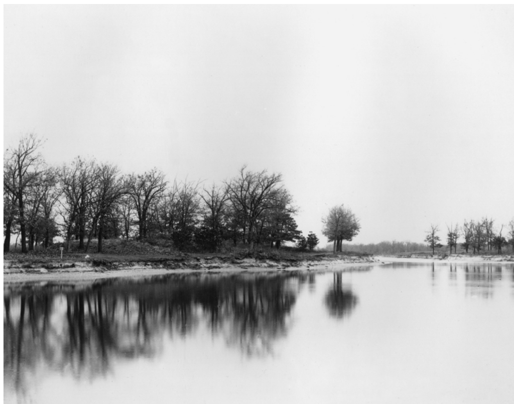
1.9 Jackson Park before construction. Photograph by Laban Deardorff.
