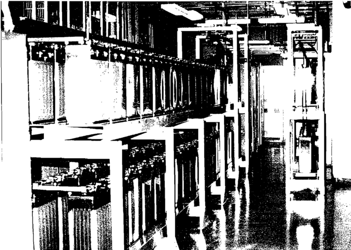
FIGURE 9.18. Room-size battery installation. (Photo courtesy of GNB Batteries Inc.)
