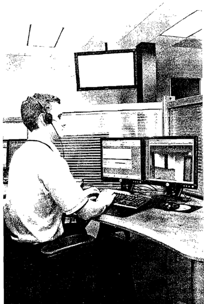
FIGURE 11.6. Central security system monitoring station. (Photo courtesy of GE Security.)
