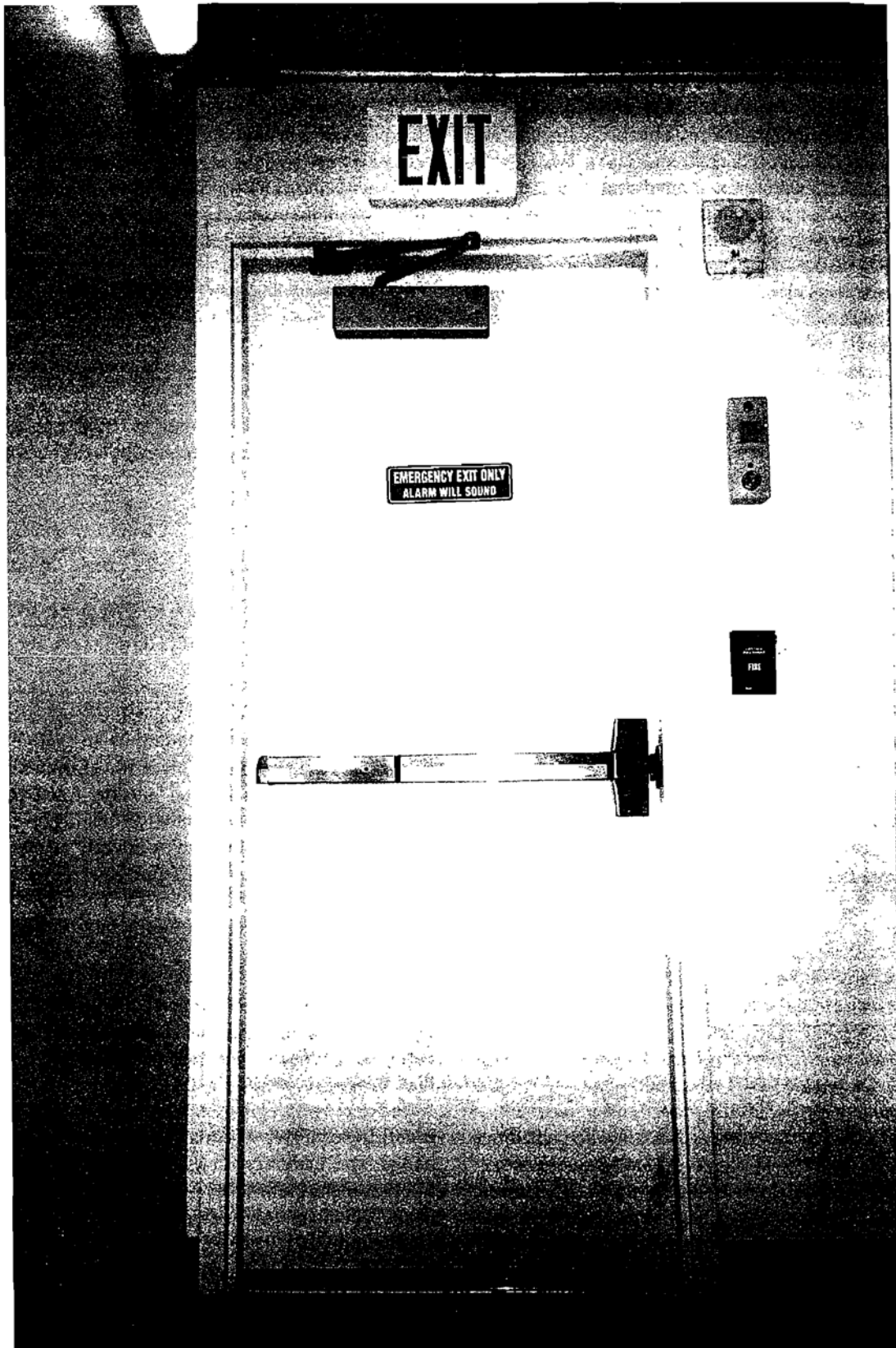
FIGURE 13.5. Panic hardware alarm. (Photo by Vaughn Bradshaw.)
