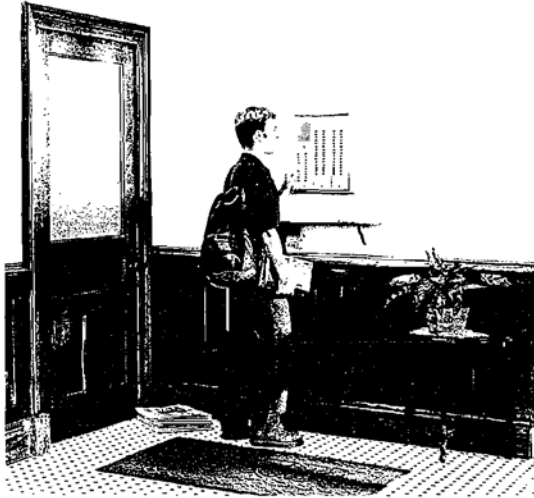
FIGURE 11.7. Apartment building lobby access control intercom. (Photo courtesy of Nutone Inc.).
