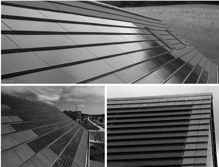
**FIGURE 6.13** Integrated PV roof tiles on the roof. (From <http://www.horizonrenewables.co.uk/>; <http://www.flickr.com/>; <http://www.archiexpo.com/>.)
