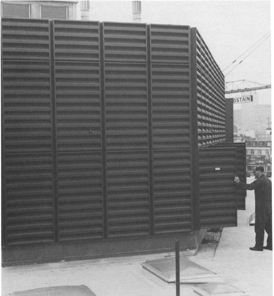
*Figure 14.11* Acoustic Louvres (courtesy Sound Attenuators Ltd)
