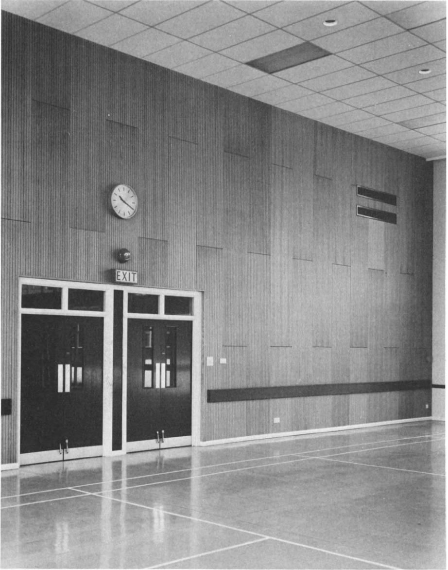
*Figure 3.17a* Absorbent Timber Wall Panel and Detail Courtesy of Sound Acoustics Ltd.
