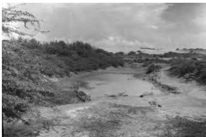
FIGURE 3.6 A percolation tank about to get dry towards beginning of summer. Location: Village: Ralegan Siddhi, District: Nagar, Maharashtra State.
