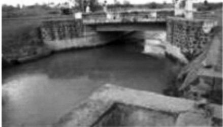
Standing wave flume along the Ghataprabha left bank canal. GLBC-standing wave flume and road bridge
