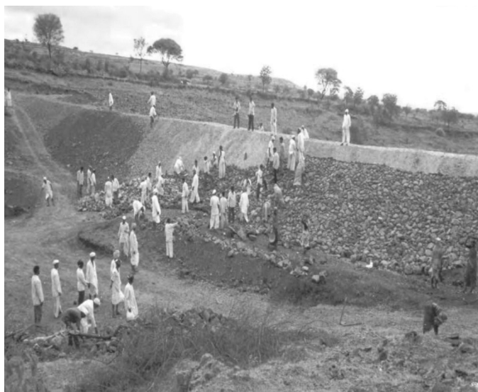
FIGURE 3.5 Stone Pitching on the face of the earthen bund of a percolation tank under construction. Photo from village Hivre Bazar, District: Nagar, Maharashtra state.
