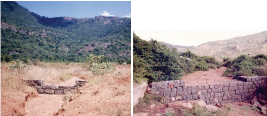
FIGURE A2.8 Temporary check dam: water harvesting.
