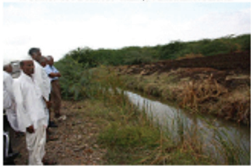
Drained off water from syb surface drainage system flowing in open channel, Jamkhandi Tahala
