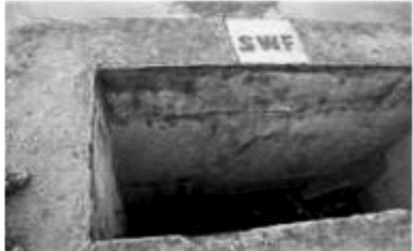
GLBC -guage well for standing wave flume
