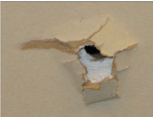
FIGURE 7.6 The lack of bullet wipe and regular smooth edges, as well as the "blasted-out" nature of frangible gypsum, characterize exits from this material.
