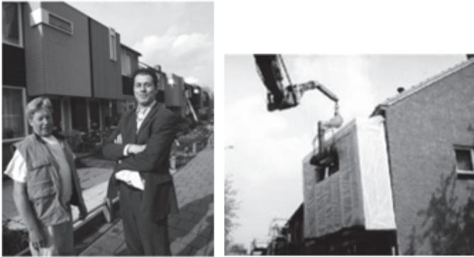
Figure 1 The practical backpack bathroom. Source Heijmans Services and [www.PZC.nl](http://www.PZC.nl)
