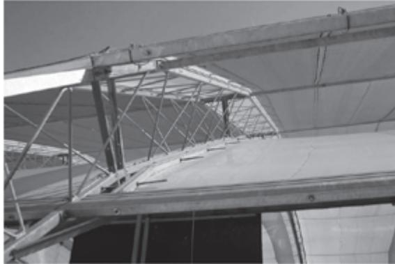
*Figure 2 Detail of the roof: truss structure, upper and lower membrane and ventilation openings*
