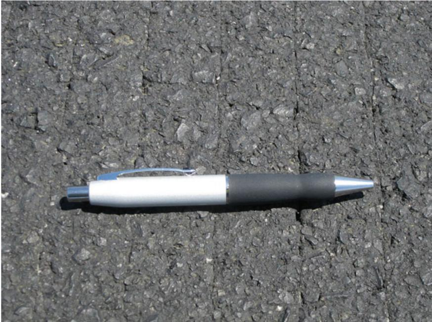
**Fig. 3.** Runway surface groove closure
