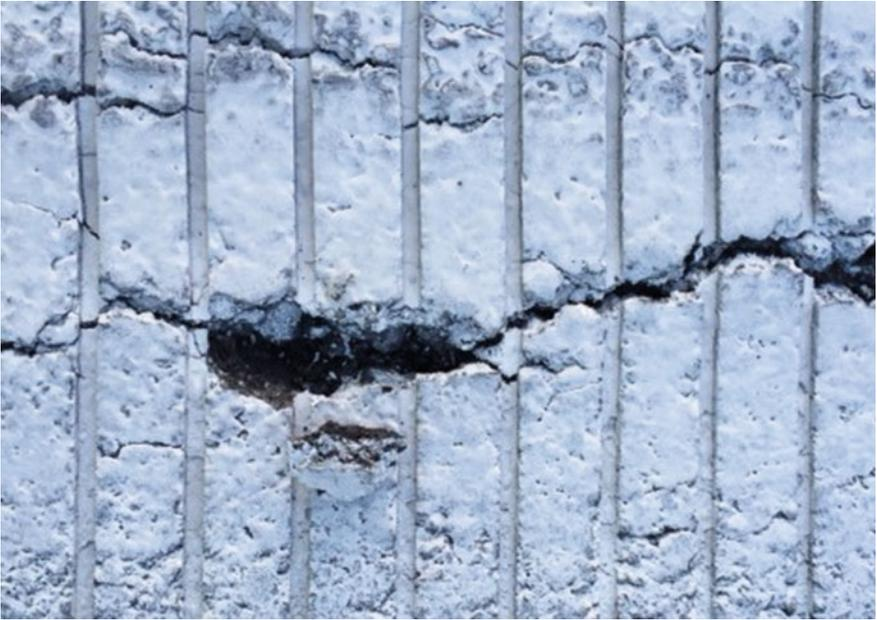
**Fig. 1.** Runway surface top-down cracking
