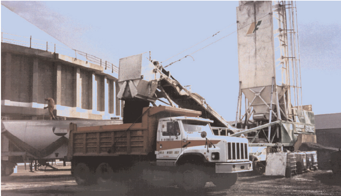
Figure 1.7. Dump trucks for transportation. (IMG15514)
