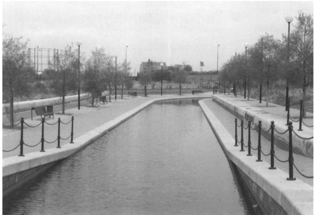
Albion Channel in Surrey Docks. This canal, formed as a connection between Canada Water and Surrey Water, was restored and landscaped by the LDDC prior to development taking place (photo: Brian Edwards)
