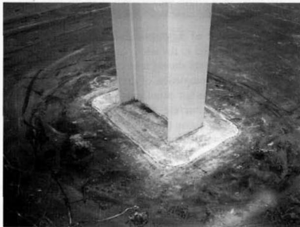
Figure 8.6: Isolation details around column.
