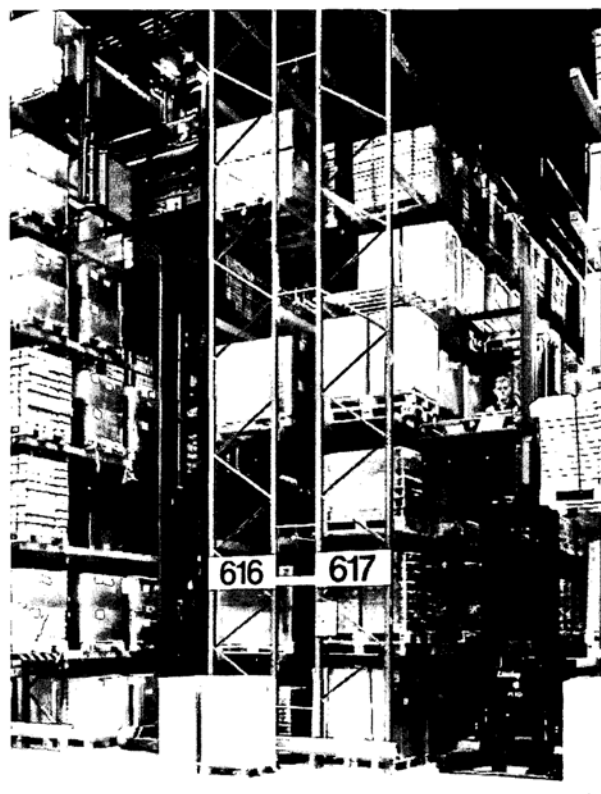
Figure 3.3: Back-to-back storage racking with 'man-up' stacker trucks operating in narrow aisles. Pallets are deposited at the ends of the racking for collection.
