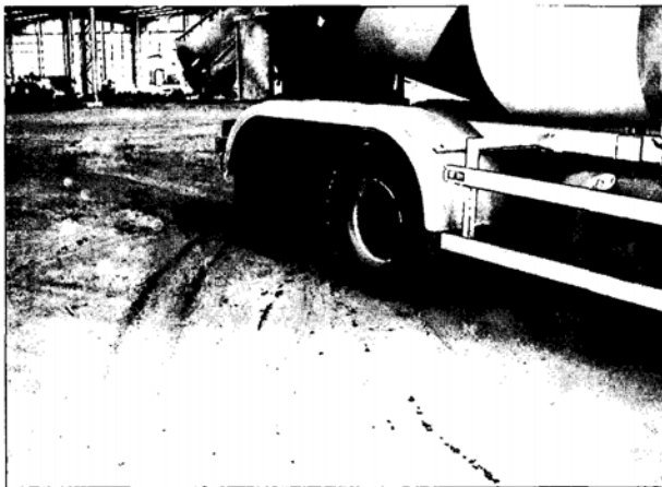
Figure 6.3: Proof loading of sub-base for construction traffic with concrete truck.
