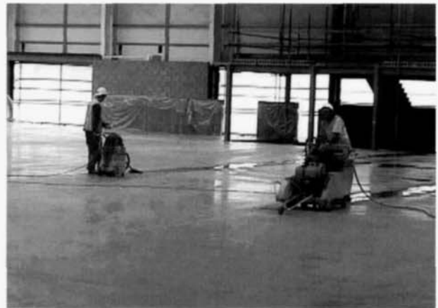
Figure 8.8: Joint sawing.
