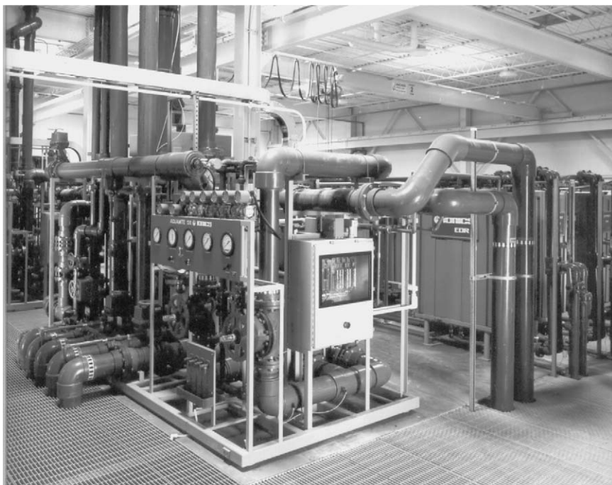
Figure 19 Industrial-size electrodesalination reversal desalination plant. Photograph, courtesy of Ionics Incorporated.
