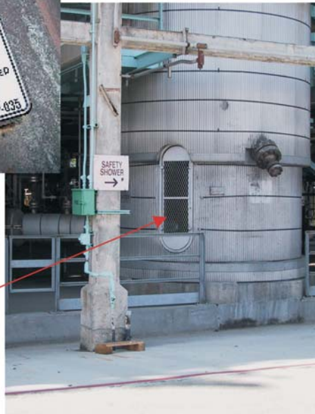
Vessel skirt manhole is closed by a locked door
