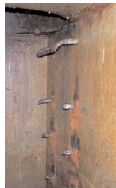
Corroded ladder rungs
