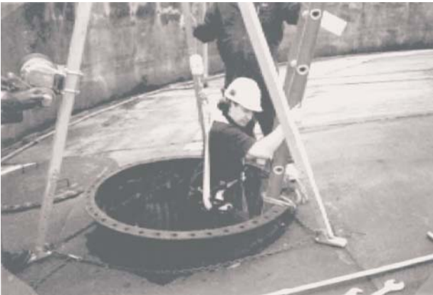
Entrant in full body harness making a correct entry into a confined space.
