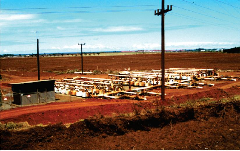
Figure 1.9. Large complex of sand media filters used to filter sugarcane mill wastewater for microirrigation, Maui, Hawaii, USA. Photo courtesy of Freddie Lamm, Kansas State University.
