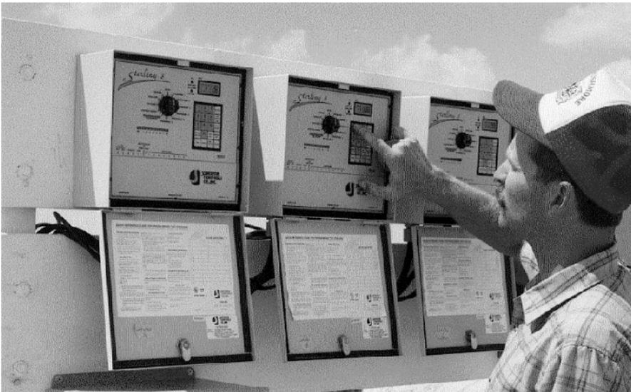
Figure 1.8. Programming an automated microirrigation system. Photo courtesy of Freddie Lamm, Kansas State University.
