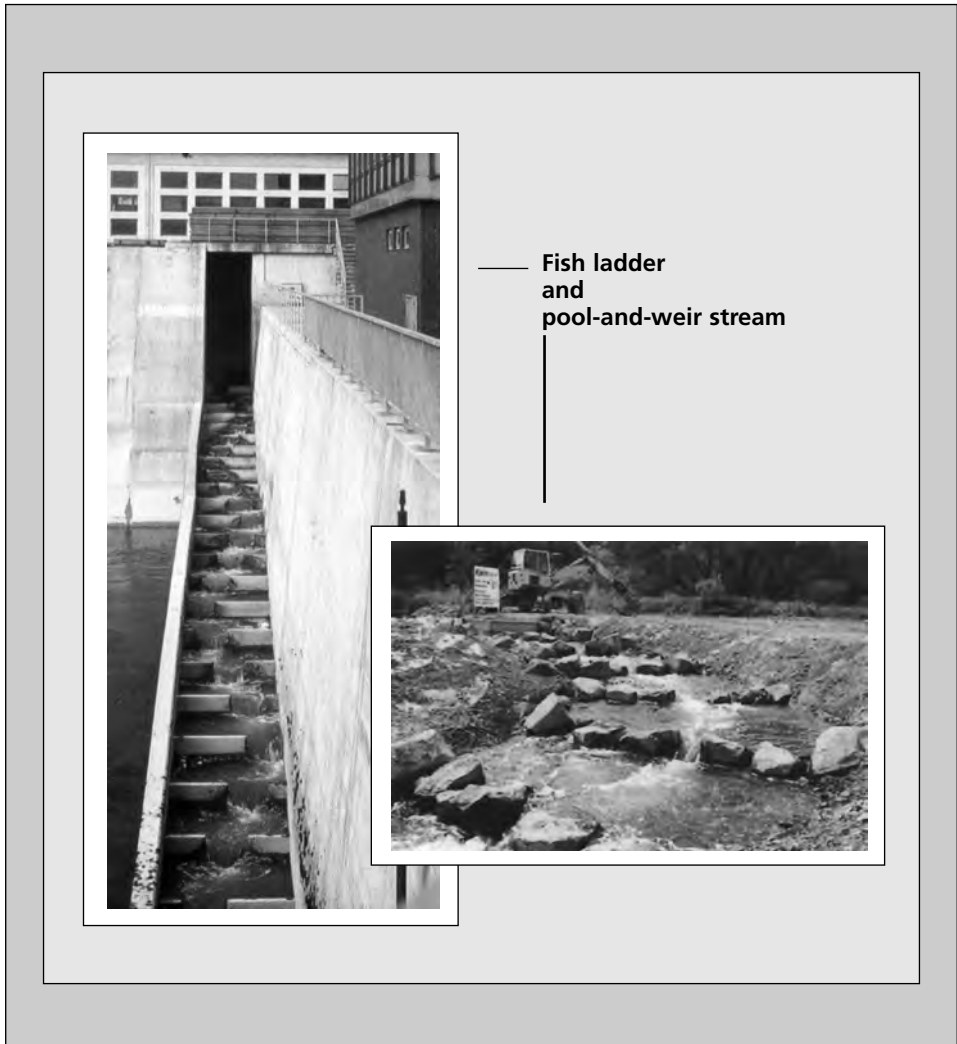
Figure 7.3 Hydropower and nature conservation: Fish bypasses
