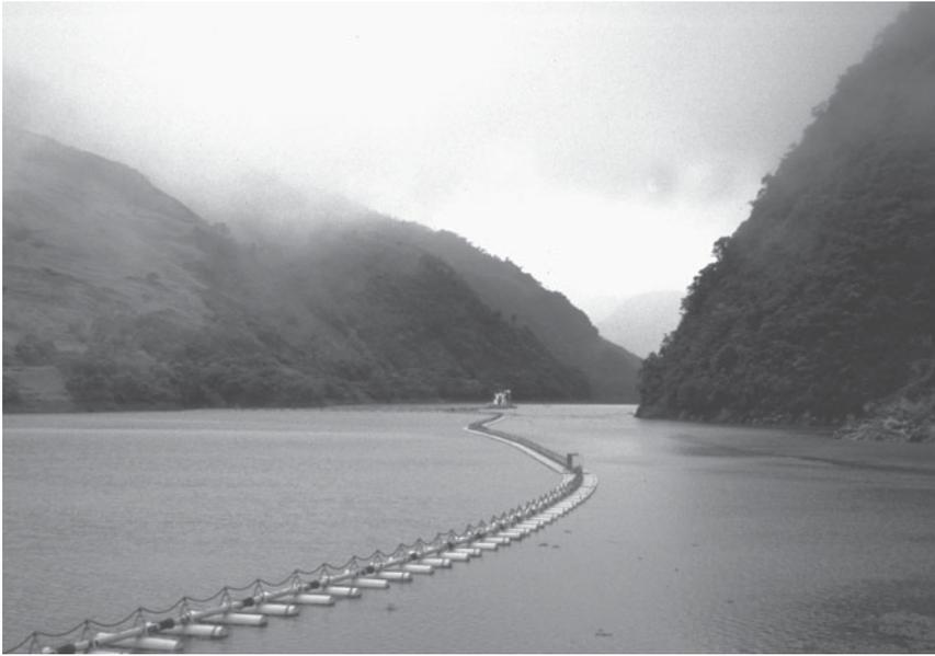
Figure 18.9 A dredge pumps sediment from the reservoir of the Paute River (Ecuador) and sends it through a floated tube to be discharged downstream of the dam (photo: C. Harden, 2002).
