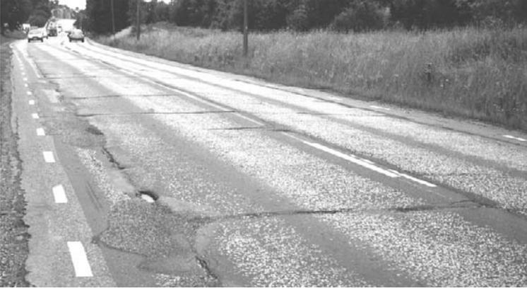
**Fig. 13.38** An asphalt overlay over a concrete pavement showing severe reflection cracking. Reproduced by permission of MacPave Corporation
