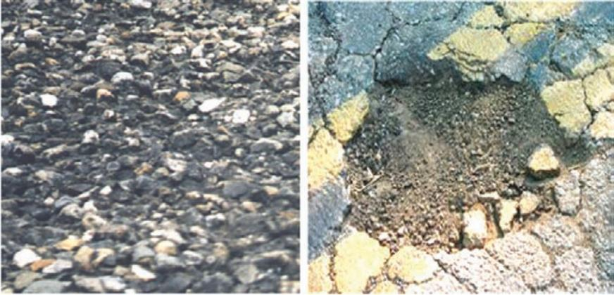
**Fig. 5.4** Water-induced damage in asphaltic material (a) ravelling (b) potholing (de Bondt, 2005). Reproduced by permission of N. Kringos
