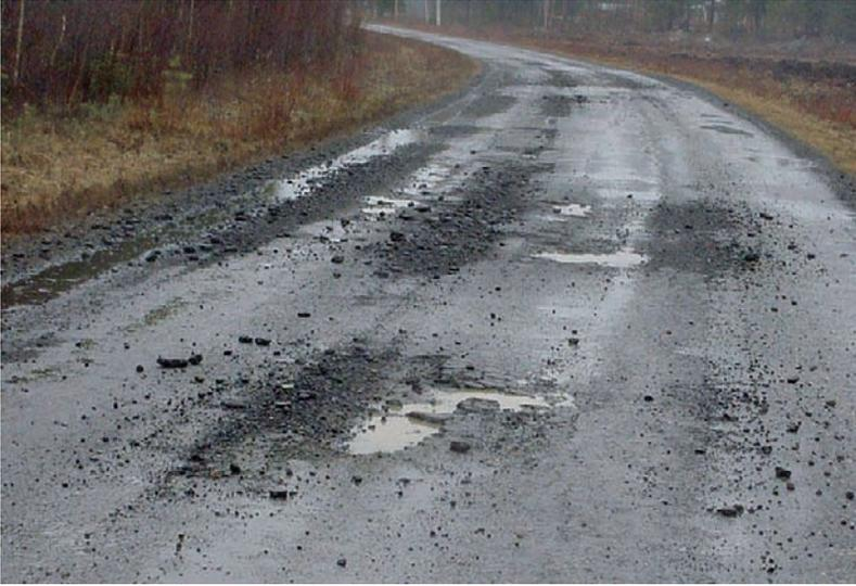
**Fig. 1.9** Thin asphaltic surfacing of a road lifted by traffic-induced water pressure during spring-thaw in Northern-Karelia, Finland. Reproduced by permission of M. Leppänen
