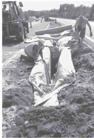
**Fig. 13.15** Trench drain (a) without pipe, (b) with pipe, (c) in central reserve<sup>2</sup>. (Credit: B. Gajewska)
