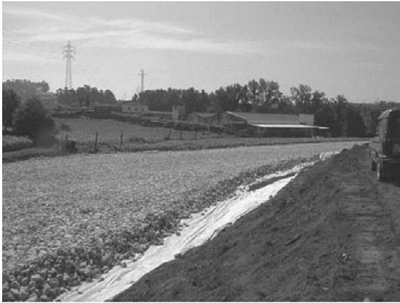
**Fig. 13.19** Drainage layers
