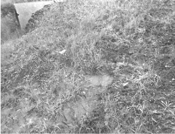
**Fig. 13.45** Water exiting from an embankment slope where it has collected due to a culvert (in the background) acting as a barrier
