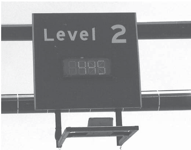
Figure D.6a. By-floor space counter linked to by-space detector system at Baltimore/Washington International Airport.
