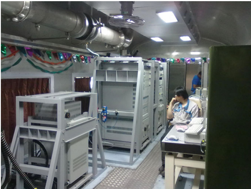
Fig. 3 Inside layout view of the exhaust sampling pipe
