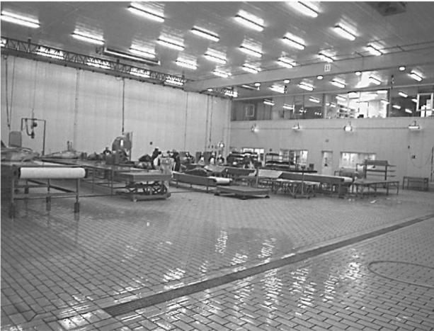
**Figure 9.10** Enclosure constructed of sandwich panels in a tuna processing room.
