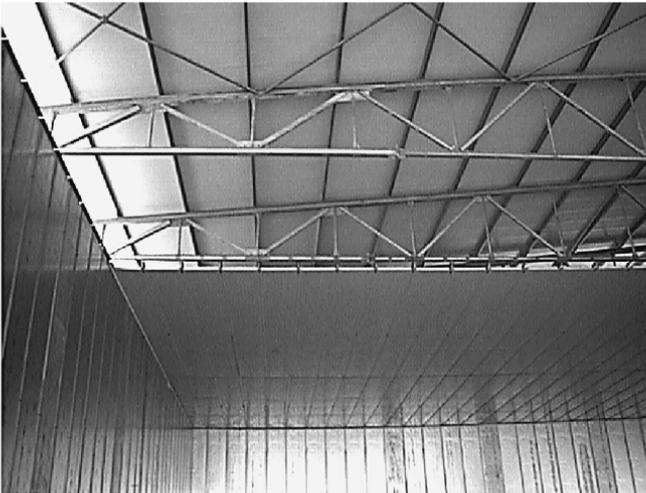
**Figure 9.12** Cold storage construction with ceiling made of polyurethane sandwich panels.
