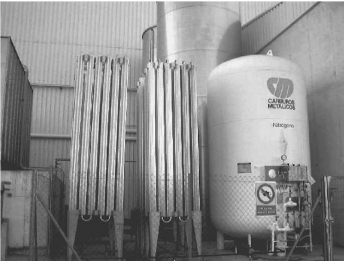
**Figure 1.10** Installation for supply of nitrogen during juice bulk storage.
