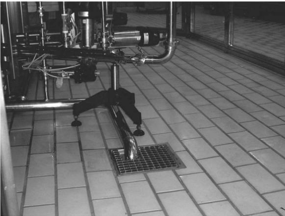
**Figure 9.18** Floor drains made of stainless steel.
