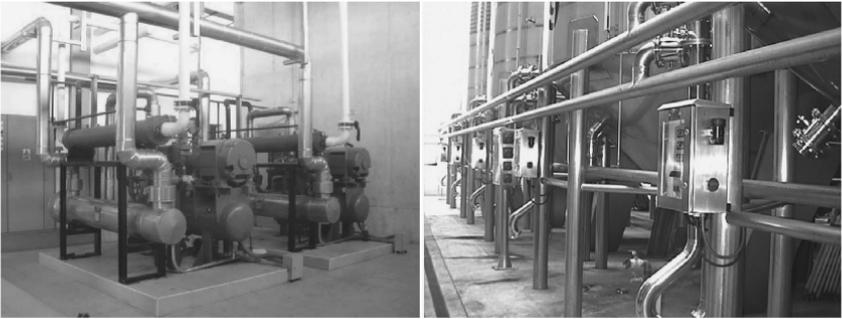
**Figure 1.1** Compressors in a mechanical refrigeration system for water cooling in a juice factory (left), and controlled temperature fermentation tanks using cool water in a winery (right).
