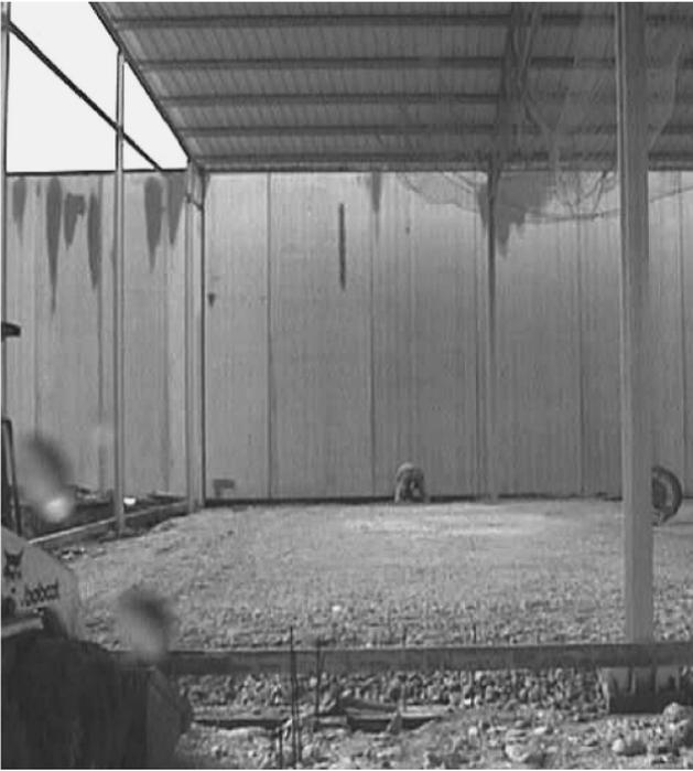
**Figure 9.13** Cold storage construction with metallic structure and stone layer floors over 20 cm thick.
