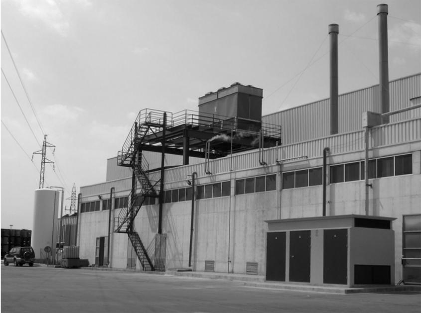
**Figure 9.7** Centralized refrigeration and boiler rooms building in a food factory. It is relatively near the processing rooms.
