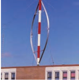
Figure 4.2 Twin-blade DAF-Indal Darrieus integrated into Canadian school circa 1980 (NRCan)
