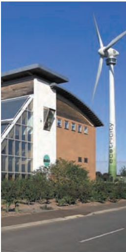
Figure 4.11 Turbine at the Ecotech Centre, Swaffham, UK (Ecotricity)
