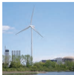
Figure 1.3 Wind energy existing alongside a nuclear power station at Pickering on Lake Ontario, Canada. A Vestas 1.8MW turbine with a blade diameter of 78m which is 150m from the nearest occupied buildings and reported to meet the electricity demands for 600 homes. (Harold L. Potts)
