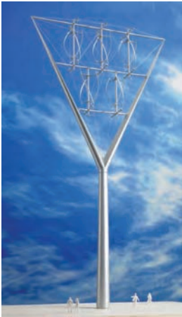
Figure 2.27 The Beacon designed by Marks Barfield Architects which consist of five 'QR5' 5kW VAWT by UK Manufacturers Quiet Revolution
