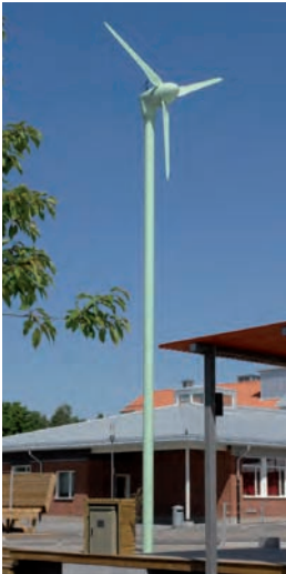
Figure 2.5 Tulipo turbine at Knivsta High School in Sweden with a 5m blade diameter, rated at 2.5kW (WES – Wind Energy Solutions)
