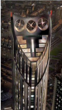
Figure 2.22 The top of the iconic Castle House residential tower, with three integrated 9m diameter HAWTs, in Elephant and Castle. The client/developer is Brookfield Europe and the architects are Hamiltons (Hayes Davidson)
