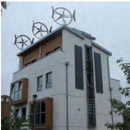
Figure 2.2 Swift (UK) turbines rated at 1.5kW with a 2m blade diameter, mounted on a Sigma Home (Renewable Devices)
