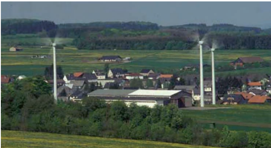
Figure 3.6 Large turbines located within fallow distance of buildings in Hoethe, Westerwald, Germany (Paul Gipe)
