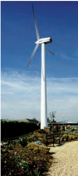
Figure 2.13 26m diameter turbine at the Wood Green Animal Shelter, Cambridgeshire, UK (Wood Green Animal Shelter)
