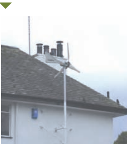
Figure 2.1 Small home-mounted turbine in Scotland from UK manufacturer Windsave, rated at 1kW and with a 1.9m blade diameter (Stewart Russell)
