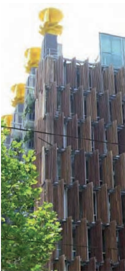
▲ Figure 5.2 CH2 building in Melbourne, Australia by DesignInc Architects
