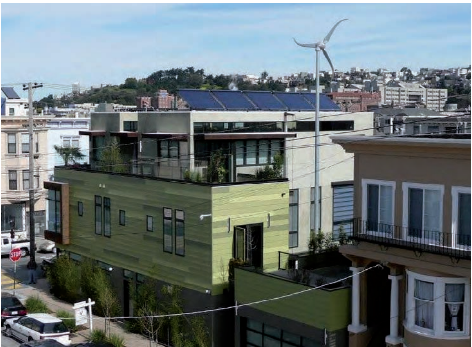
Figure 2.7 Skystream 3.7 from US manufacturer Southwest Windpower as part of La Case Verde, a sustainable residence made from recycled materials in San Francisco, California. The full installation, including permits, was around US$20,000. (Robin Wilson)
