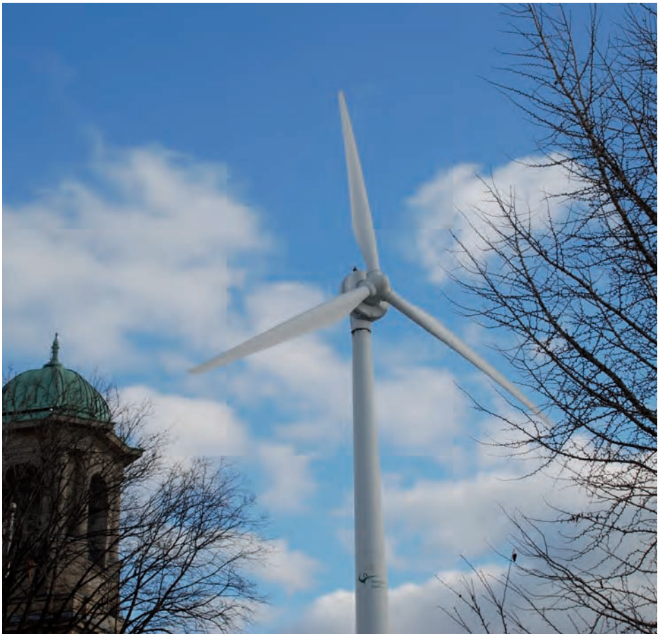
Figure 3.14 Toronto turbine manufactured by Lagerwey (now Emergya Wind Technologies manufacturing mid-range turbines available with either 750kW or 900kW) (Harold L. Potts)
