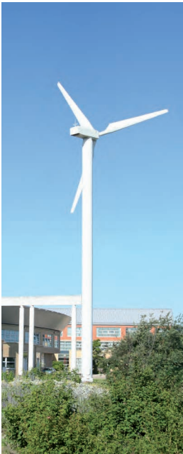
Figure 2.10 Leonardo Da Vinci School in Calais, France with a 20m diameter (hub height 35m) turbine rated at 130kW, from Dutch manufacturer Vestas (Frédéric Allard)
