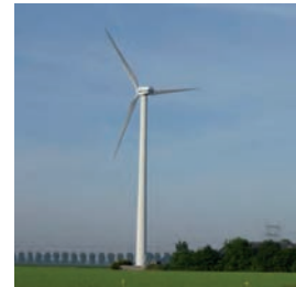
Figure 4.15 Vestas V47, 47m blade diameter, which may be available as a re-engineered turbine
