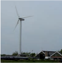
Figure 4.14 A Re-engineered Micon M350 (250kW 26m blade diameter)
