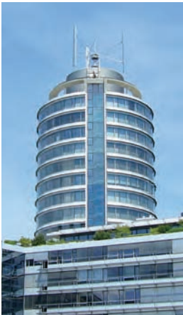
Figure 2.25 'H-Darrieus type' of VAWT integrated into the design of the Technisches Rathaus, Munich, Germany
