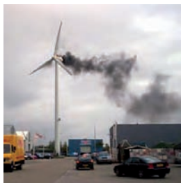
Figure 3.7 Turbine malfunction in Herenveen in Holland
