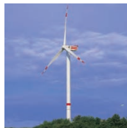
Figure 1.6 The largest production turbine from German manufacturer RePower rated, at 5MW and with a 126m blade diameter (Jan Oelker & RePower)
