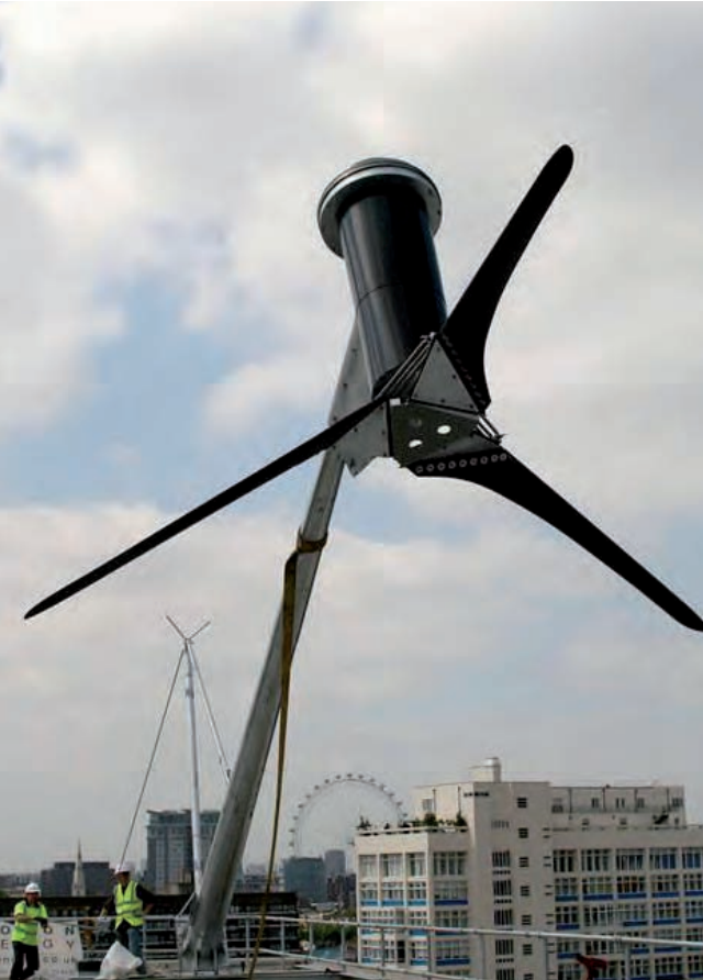
Figure 4.12 6kW Proven turbine being erected on the roof of Ashenden House, London (2007) (Photon Energy)
