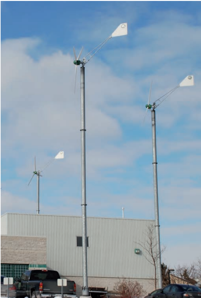
◀ Figure 4.13 Ontario Electrical Construction Company visibly supporting wind energy (Harold L. Potts)
