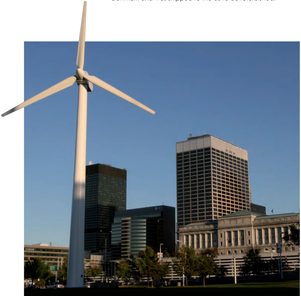
Figure 2.14 Great Lakes Science Center 27m diameter turbine in Cleveland USA, rated at 225kW, from Dutch manufacturer Vestas (V27) (Jim Kolmus)
