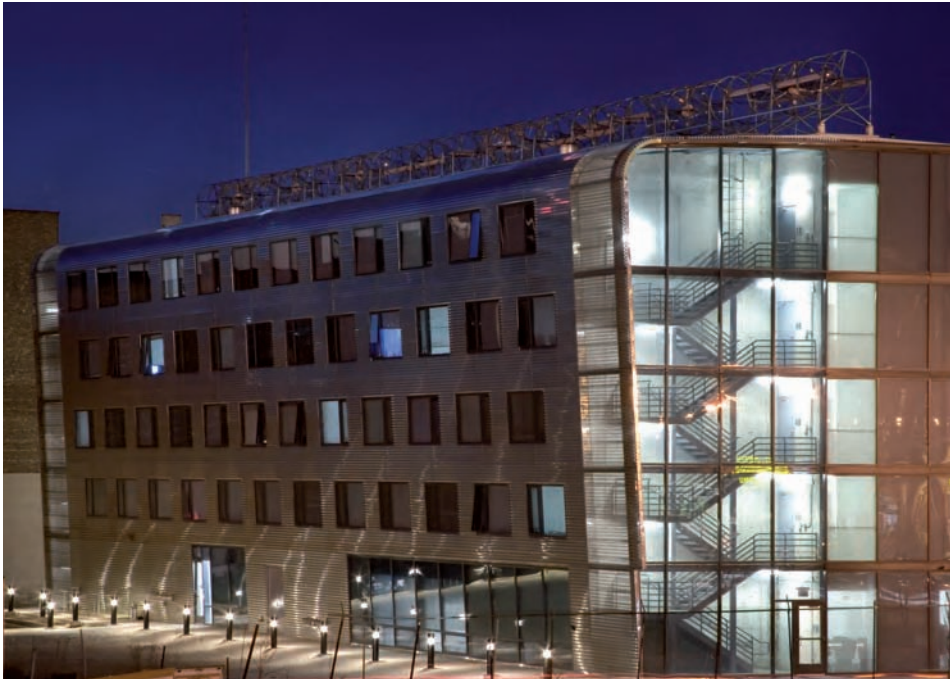
▲ Figure 5.18 Building-integrated turbines on the Margot and Harold Schiff Residences project by Murphy Jahn Architects using Aerotecture ( www.aerotecture.com ) horizontal VAWT to feed 96 apartments (with other green features such as solar thermal and rainwater collectors) in North Clybourn Avenue, Chicago (2007) (Doug Snower Photography, Chicago)
