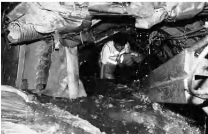
*Figure 7.11* River of water out of pilot tunnel TBM, Ping Lin, Taiwan.
