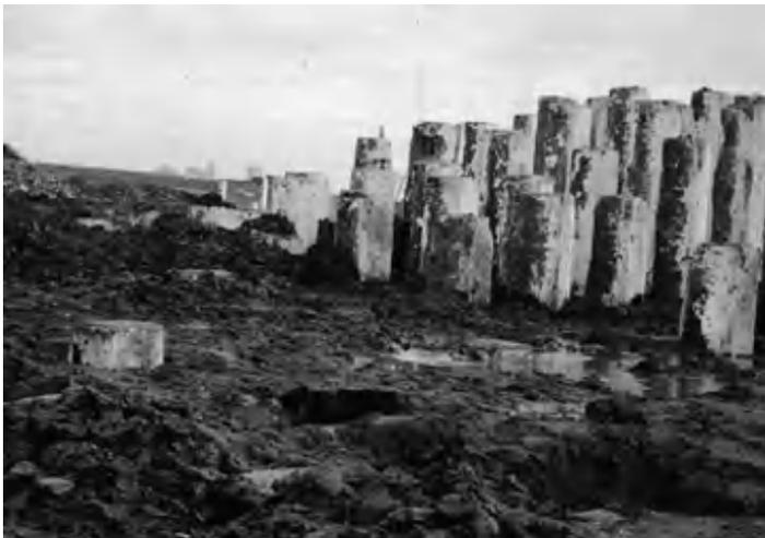
*Figure 7.19* Driven piles at Drax Power Station completion. Dark holes in foreground are where pile heads have been driven below carpet level without achieving an adequate set and need re-driving.
