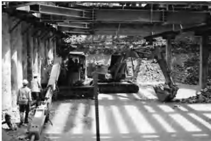
*Figure 6.2* Temporary works for an underground station construction in Singapore. Piles to the left were excavated by a large-diameter drilling rig and then concreted. As excavation has proceeded, the piles have been anchored back into the ground and strutted using systems of waling beams (horizontal, along the face of the piles) and struts, supported where necessary by additional king posts.
