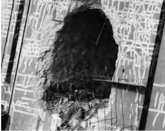
*Figure 7.4* Cracks in face of the Pracana Dam, Portugal, due to alkali-silica reactivity from use of reactive aggregates in concrete (reproduced with kind permission from Ilidio Ferreira, Head of Dam Safety Department at EDP, Portugal).
