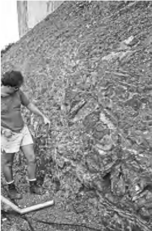
*Figure 5.16* Cut slope through weathered volcanic tuff.
