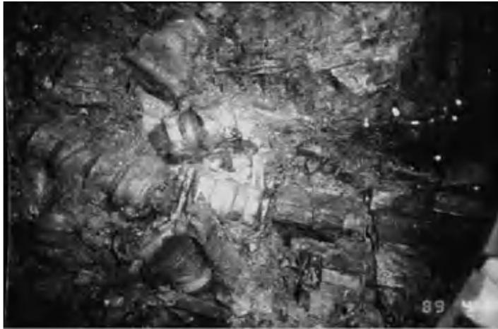
Figure 7.9 Collapse of fault zone around TBM – exacerbated by attempt to move TBM backwards, which necessitated emergency backfill and grouting above the tunnel.
