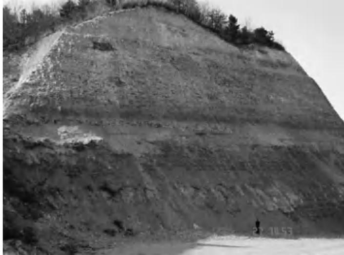
Figure B6-5.1 View of large cut slope in Eocene mudstone near Po Chang Korea.
