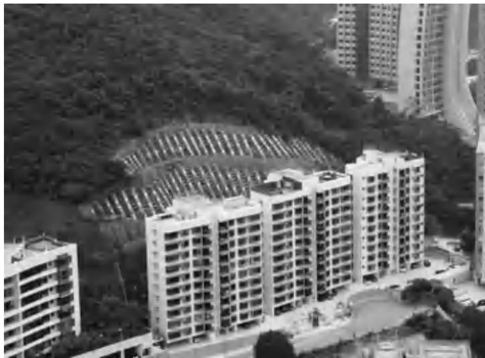
Figure B1-2.4 Slope in 2010 showing anchored concrete beams installed to prevent further failure in the trimmed-back slope above the apartment blocks.
