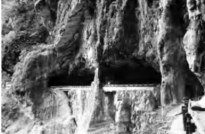
*Figure B6-4.3* Road cut through limestone with very little engineering support or protective measures, Tailuko Gorge, Taiwan.
