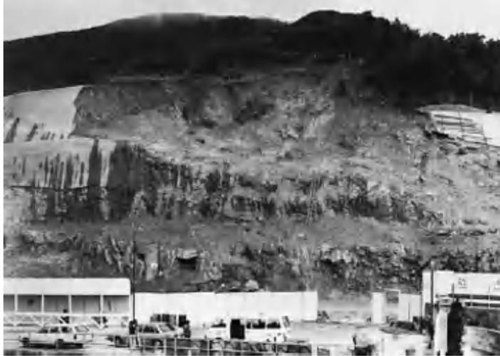
Figure B1-2.1 View of large rock slope failure in 1982, South Bay Close, Hong Kong.
