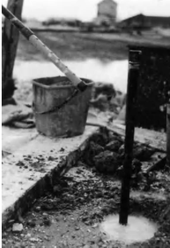
*Figure 4.40* Standpipe piezometer tip about to be placed in borehole. Another has already been installed at a deeper level. It is not very good practice to install more than one piezometer in a borehole, because of potential leakage between the different horizons being monitored, but can work providing great care is taken in installation. Portsmouth dry dock, UK.
