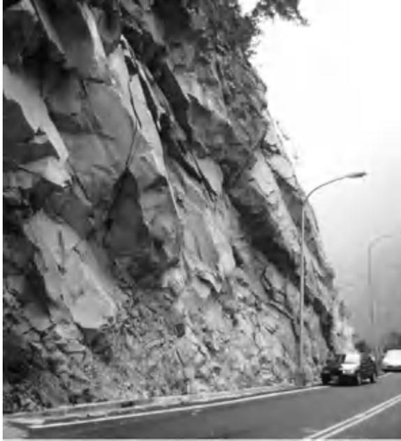
*Figure 5.19* Well-defined daylighting discontinuities, clearly only stable due to imperistence (cohesion), Taiwan.
