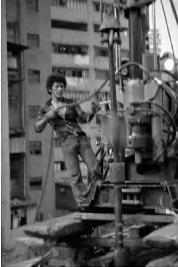
*Figure 4.31* SPT test underway in Hong Kong (1980s). Nowadays, a helmet would be worn.
