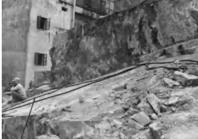
Figure B5-2.1 Failure plane with debris cleared off.
