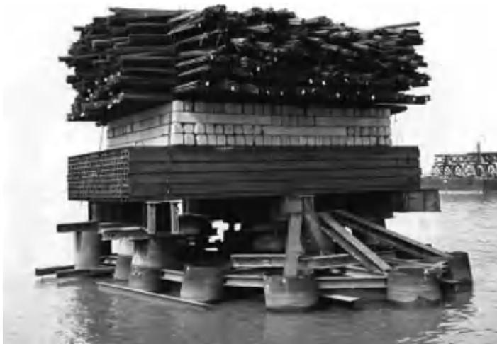
*Figure 6.9* Pile test set up with kentledge. Donghai Bridge, China. Figure courtesy of Leonard Tang, Halcrow.
