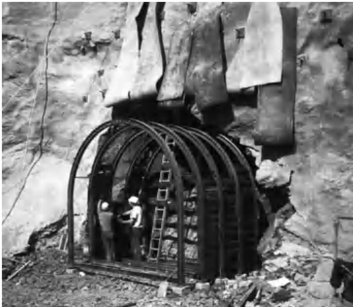
*Figure 6.15* After first blast and mucking out, construction of temporary steel arches to protect tunnel portal, Queens Valley Reservoir, Jersey, UK.
