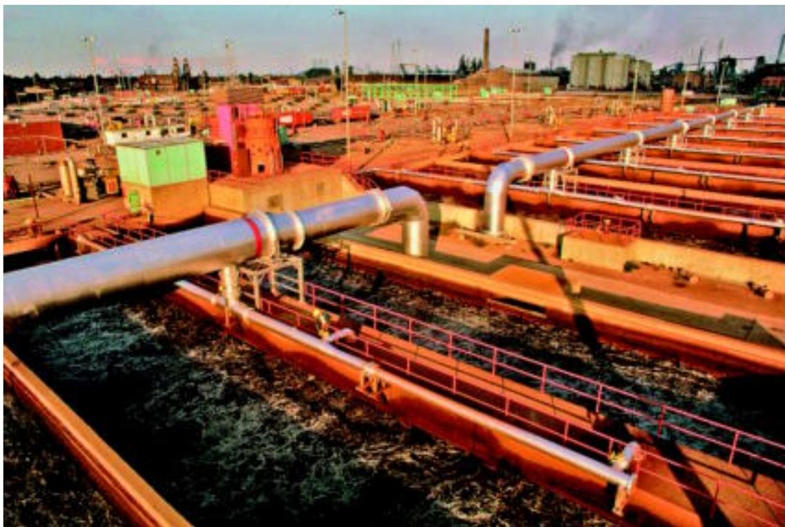
Equipment at the Detroit Municipal Sewage Water Treatment Plant. Solid wastes are removed from sewage and treated separately. © Ted Spiegel/Corbis.
