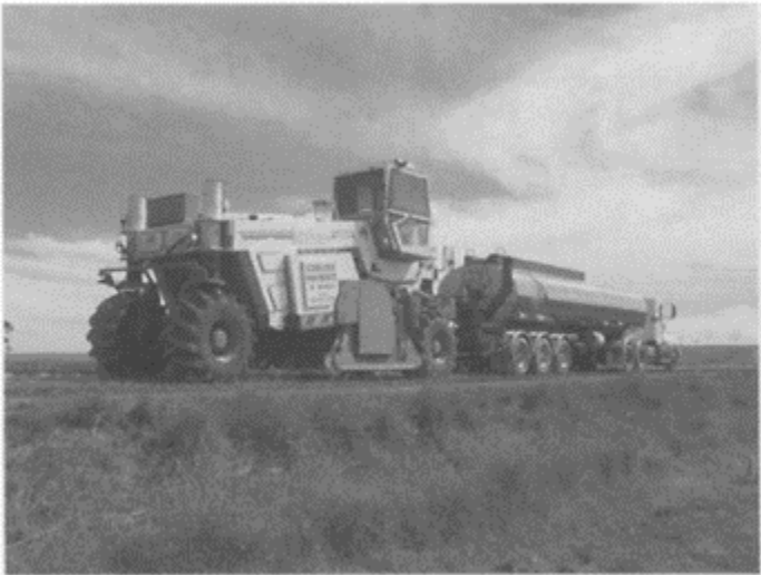
Figure 1. Foamed bitumen stabilisation using a Wirtgen 2500 reclaimer/stabiliser.
