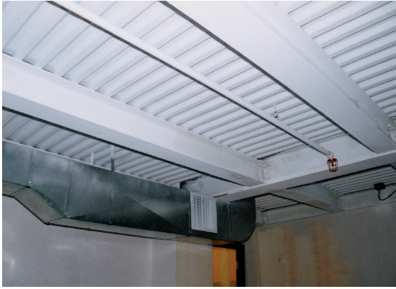
Figure 5.5 Steel floor deck and steel beams
