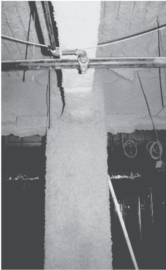
Figure 18.15 Column with spray-on fire protection
