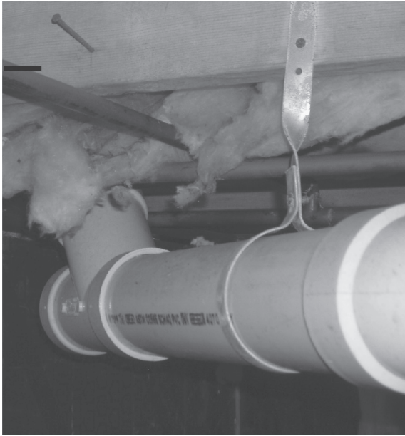
Figure 10.4 Plastic waste pipe
