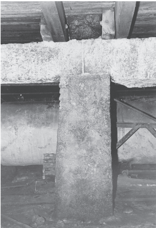
Figure 4.6 Stone beams and column, Pemberton Mill, Lawrence, Massachusetts, 1967
