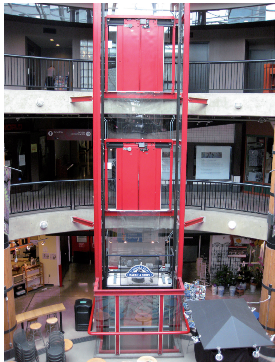
Figure 19.11 Glass-enclosed elevator
