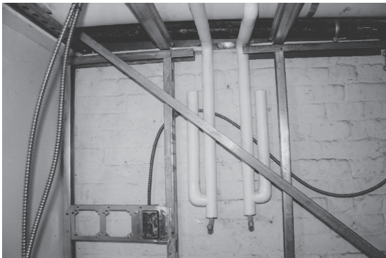
Figure 9.11 Masonry wall with furring for plumbing
