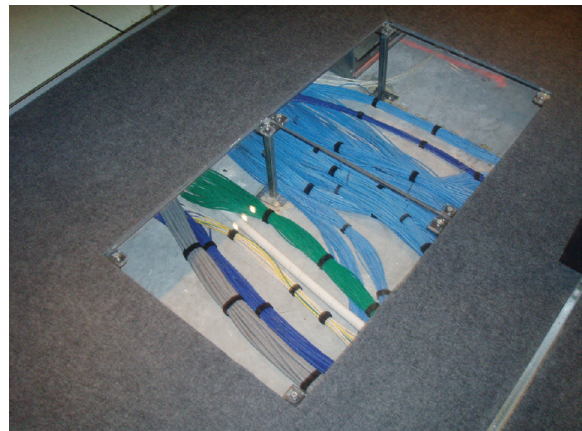
Figure 20.6 Access floor data cables
