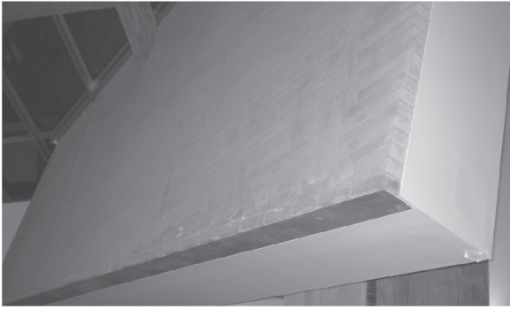
Figure 8.24 Interior brick and concrete wall, Stata Center, Massachusetts Institute of Technology
