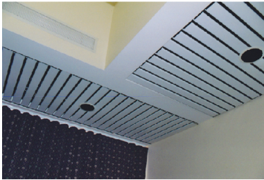
Figure 8.30 Linear metal ceiling
