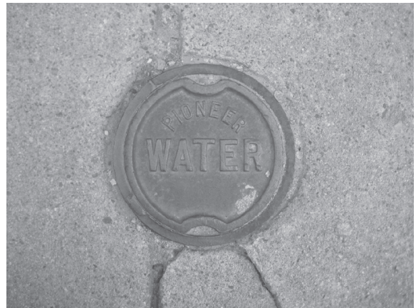
Figure 9.9 Water shutoff cover
