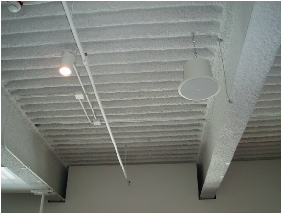
Figure 8.39 Sound masking equipment
