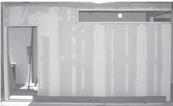
Figure 8.25 Gypsum wallboard partition with openings Source: Courtesy of Herb Fremin
