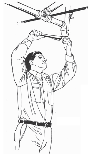
Figure 9.15 Plumber opening trap
