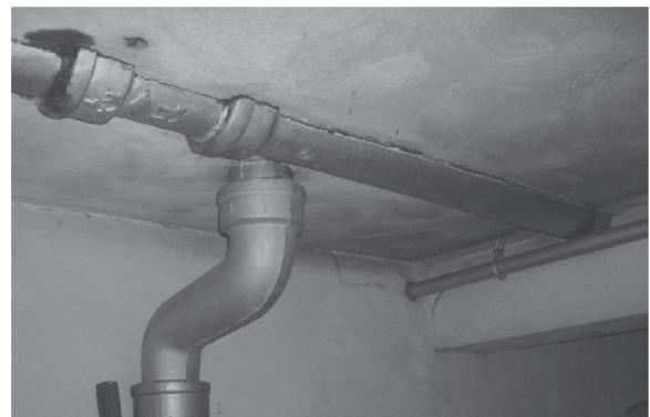
Figure 10.3 Cast iron pipe
