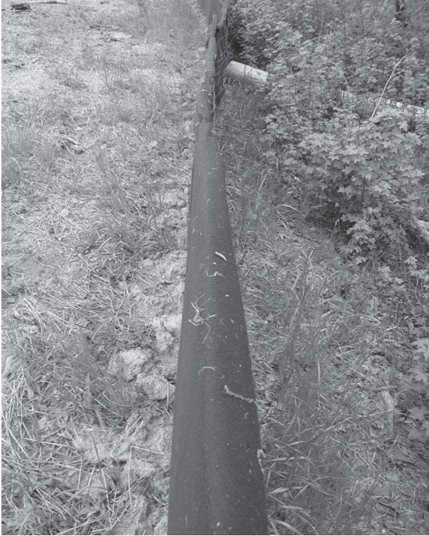
Filter fence along edge of property line (front side to left).
