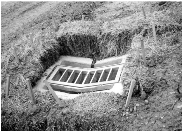
Typical straw bale barrier surrounding inlet (notice tight bales and large amount of sediment collected around outside of bales, needing removal).
