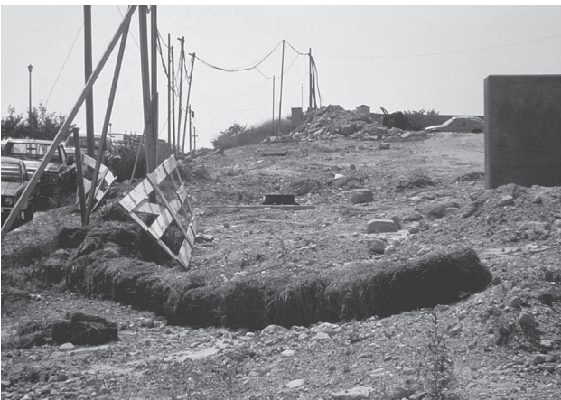
Hay bale barrier along edge of pavement.
