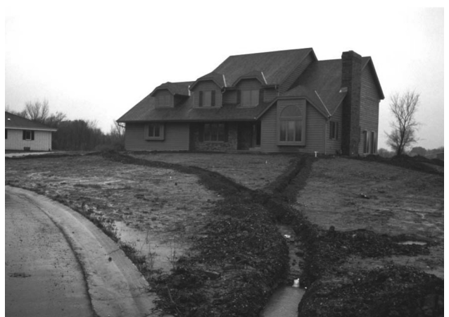
A small utility trench can cause high turbidities in downstream runoff.
