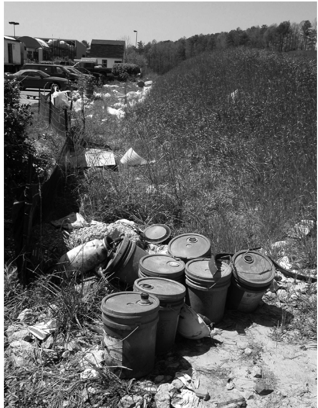
Unsafe storage disposal of empty oil containers at construction site.
