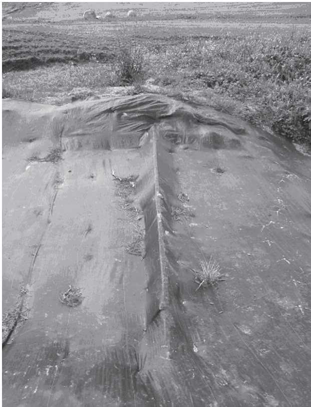
Temporary outlet made from level timber placed at correct elevation and covered with plastic to protect spillway (Auckland Regional Council).
