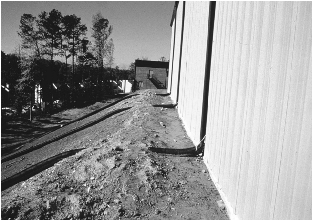
Small-scale slope diversion to safely carry roof runoff away from building and down sensitive adjacent slope.
