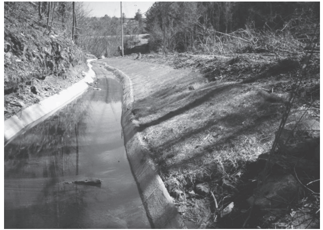
Concrete lined channel, with reinforced matting along overflow area.
