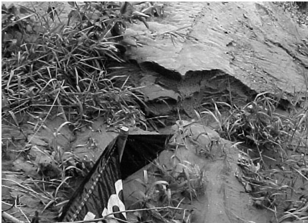
Inspections must require replacement of damaged erosion controls (J. Voorhees photo).
