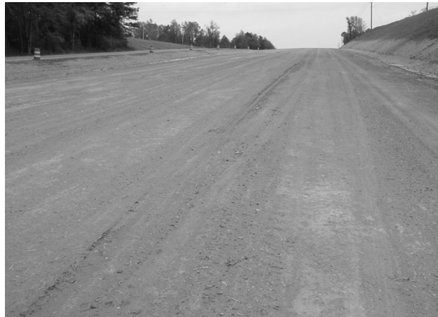
Unprotected newly graded area at highway expansion project.
