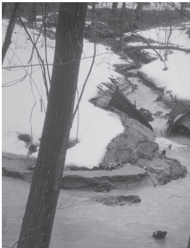
Filter fabrics rarely made adequate check dams (Photograph by D. Lake).
