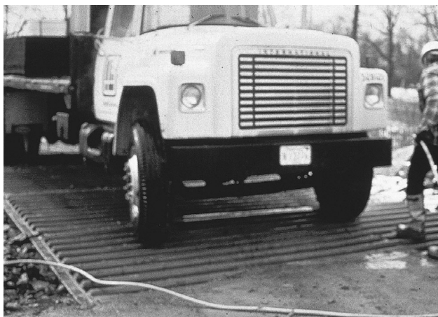
Truck being cleaned as it leaves construction site for public right-of-way.
