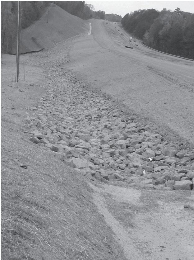
Large rocks for channel reinforcement.
