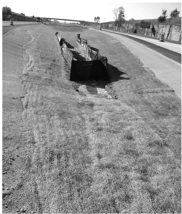
Inlet protected by filter fabric, thick matting to protect new grass, and chemically stabilized soil (Illinois).
