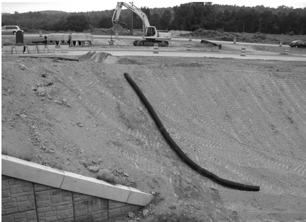
Highway slope diversion during initial construction.
