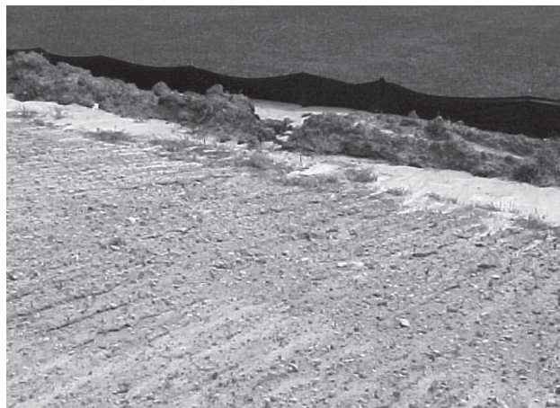
Sheet and rill erosion on hillside.
