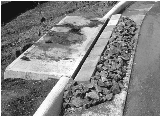
Older concrete block and stone inlet barrier (historical SCS photo).
