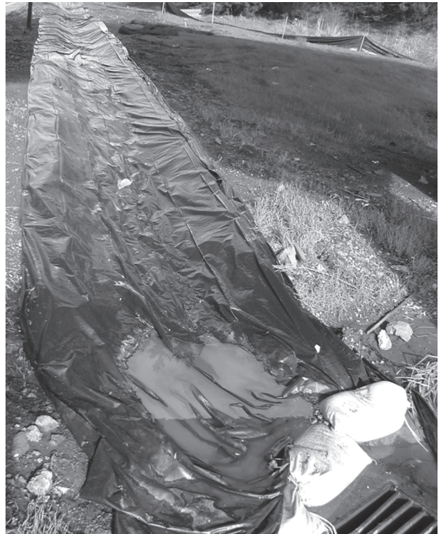
Plastic tarp used as a temporary liner.
