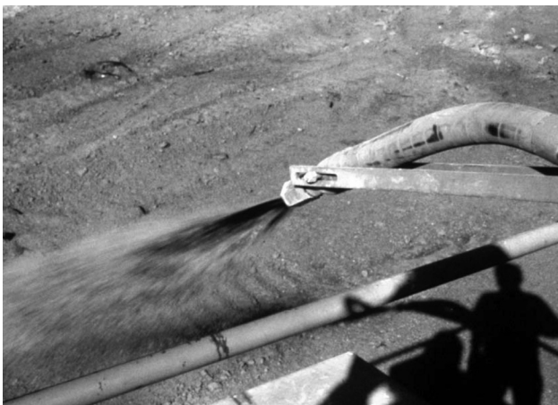
Spray mulch blown to protect exposed soil.
