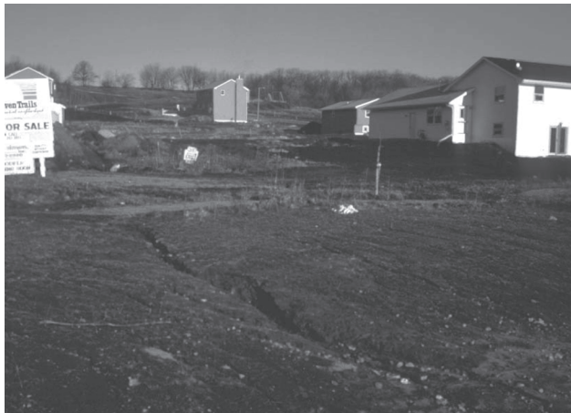
Large-scale sheet and rill erosion and isolated gully erosion beginning to start at an inadequately protected construction site.
