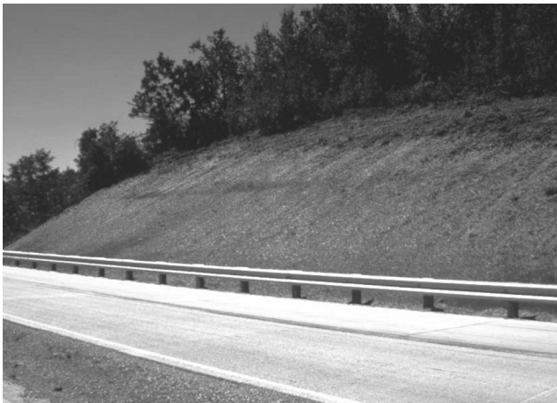
Newly installed erosion control mats on steep highway embankment.
