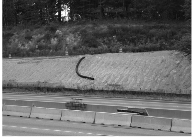
Temporary slope diversion at highway construction site.
