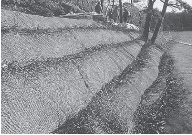
Bioengineered channel slopes (IECA photo).
