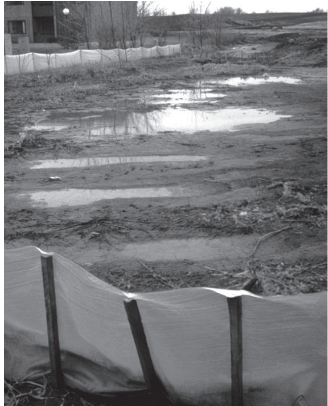
Temporary construction site pond filled with sediment
