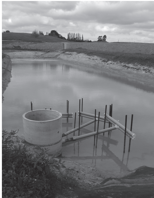
Multi-level, perforated, floating discharges (decants) to better retain floc.
