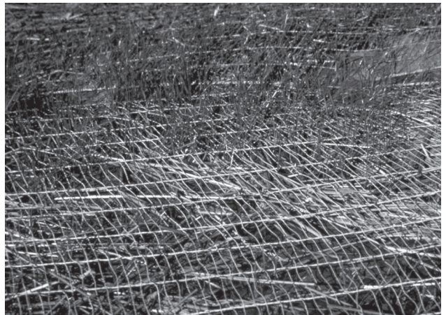
Mesh placed over seed and mulch.
