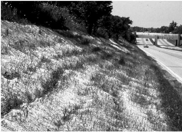
Vegetation starting to grow through erosion control netting at highway construction site.
