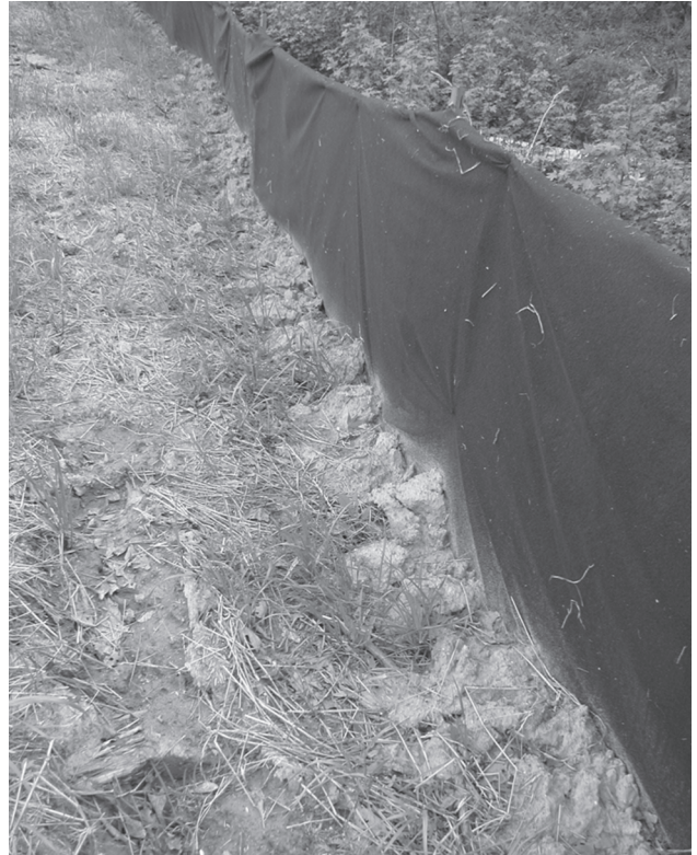
Well-installed filter fabric fence, with bottom of fabric buried and backfilled to prevent underflow of sediment.
