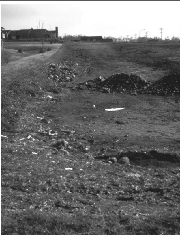
Inspections need to monitor sediment accumulations. This dry sediment pond is almost full of accumulated material.
