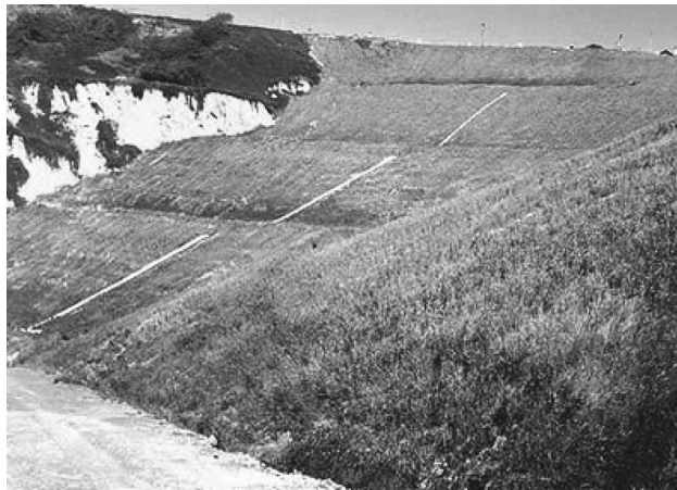
Large slope diversions carrying water from upslope benches (IECA photo).
