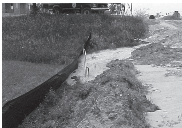
Large sediment load captured by filter fence, maximum load before needed maintenance (J. Voorhees photo).
