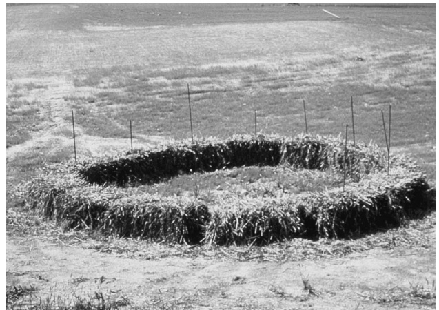
Straw bale barrier showing large gaps between bales and decomposing bales, needing replacement (SCS photo).
