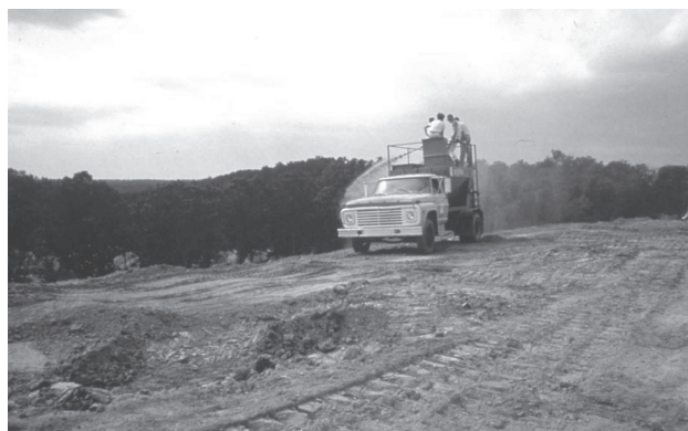
Temporary hydroseeding for erosion control (SCS photo).
