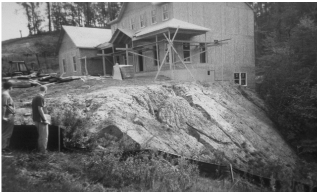
Erosion Threatening Homes (This home is actually being constructed on 12 feet of fill soil. The foundation footers are 14 feet below the groundline. Note the rills draining down to the drainage swale) (Photographs by D. Lake).
