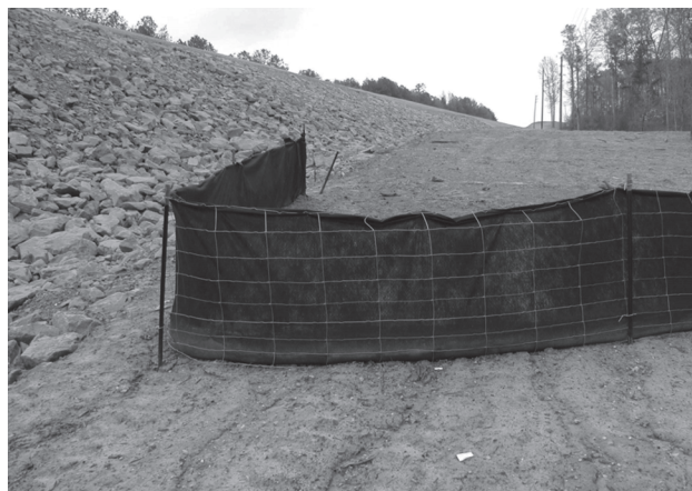
Evidence of underflow erosion beneath improperly installed filter fabric fence.
