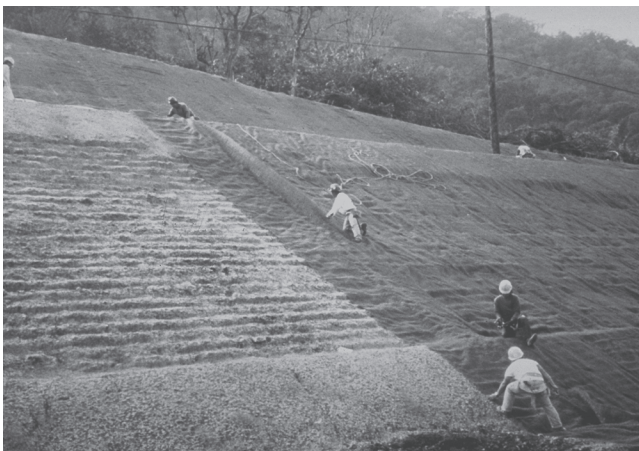
Installation of Netting over Mulch (Photograph by Synthetic Industries).
