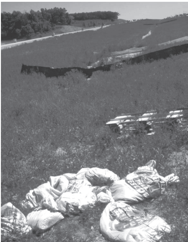
Seeding along median strip swale of highway project.
