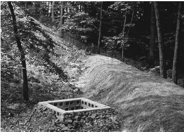
Cinder block and gravel barrier to protect inlet (SCS photo).
