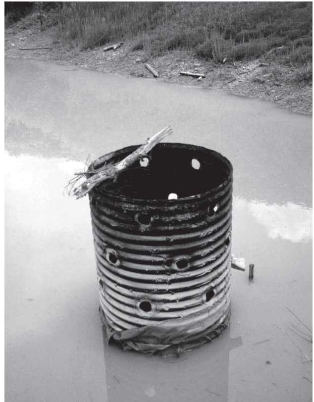
Vertical riser having multiple outlets and wrapped with geotextile fabric (Poor design, as no cap is provided).
