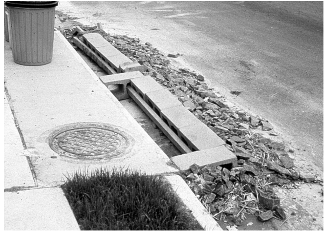
Older concrete block, lumber, and stone inlet barrier (historical SCS photo).
