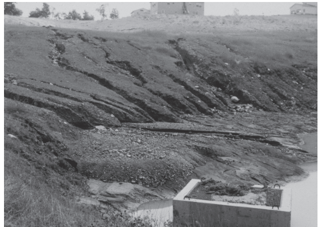
Extensive gully erosion on unprotected steeper slopes of detention pond.
