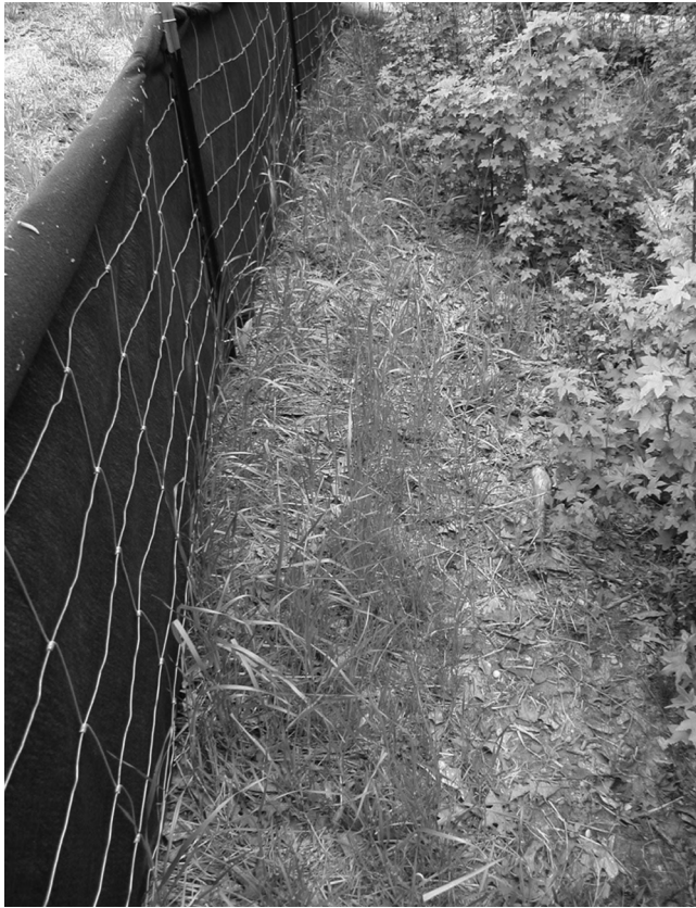
Downslope side of perimeter filter fence intercepting sheetflows.
