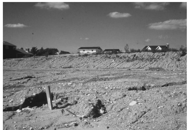
Unattended severely eroded land causes great amounts of sediment loss and requires site regrading.
