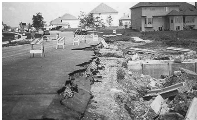
Damaged from erosion requiring repairs (IECA photo).
