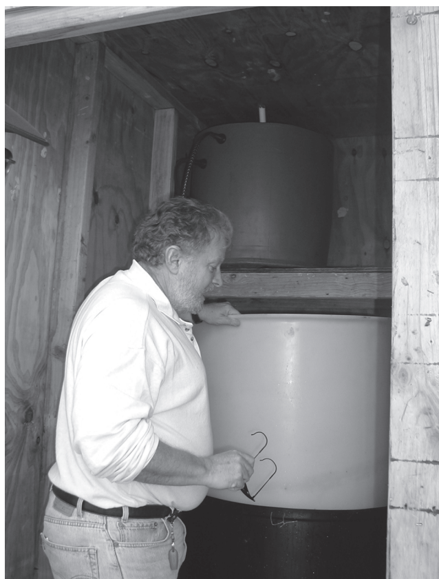
Earl Shaver of the Auckland Regional Council showing the main components of the rainfall-driven chemical dosing system.
