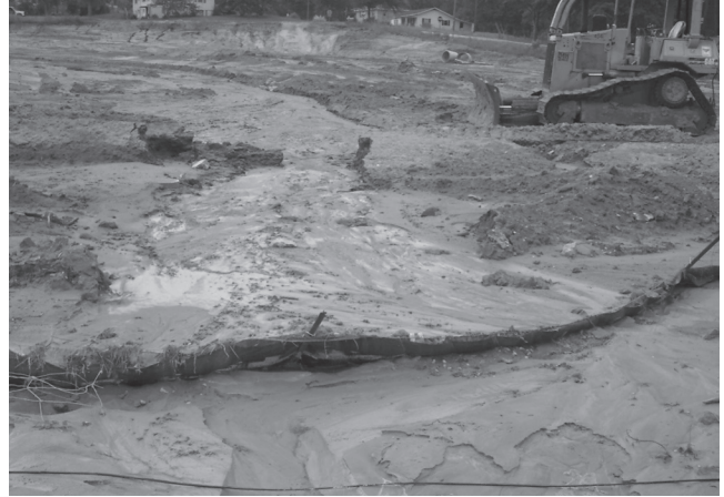
Caroline Sandel, UA student: silt fence overloaded.
