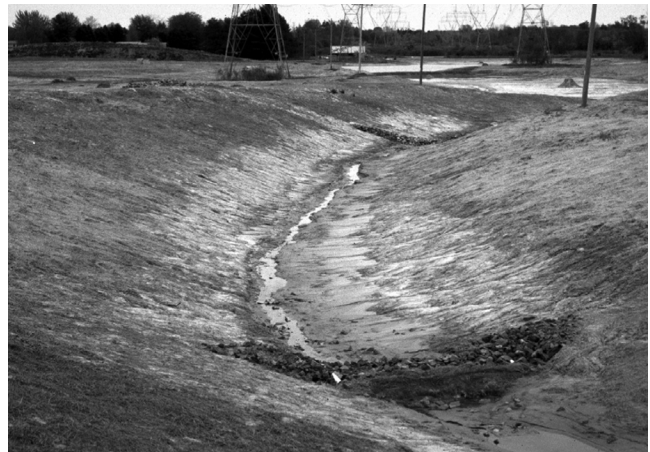
This exposed site is under a state shutdown order for destroying 2 acres of walleye spawning area in a nearby lake. 65 acres of the 70 acre site was stripped exposing soil containing 75–98 percent fines that could not settle out on site.
