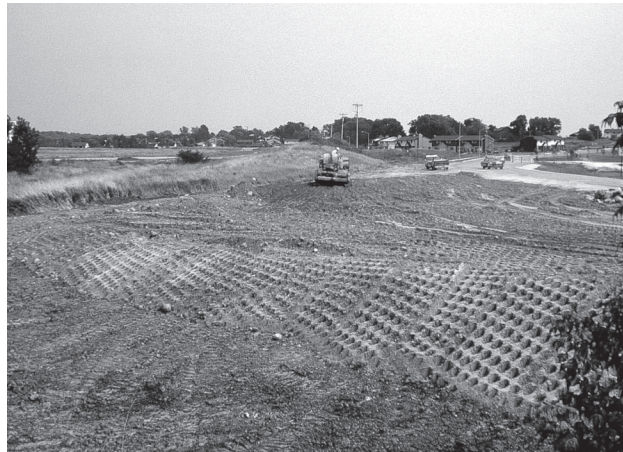
Roughened and compacted slope.
