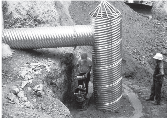
Vertical riser with inlet grate (MD photo) (normally the culvert discharge for the riser would be closer to the pond bottom to facilitate de-watering).
