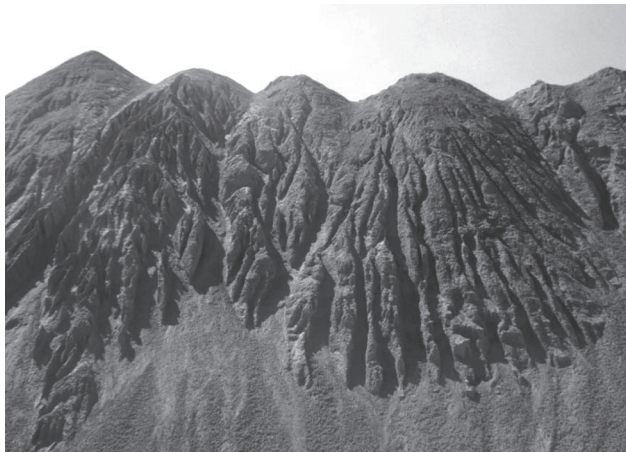
Small-scale sheet erosion on tops, rill erosion forms further downslope, and finally deposition zones, on a material stockpile at a construction site.
