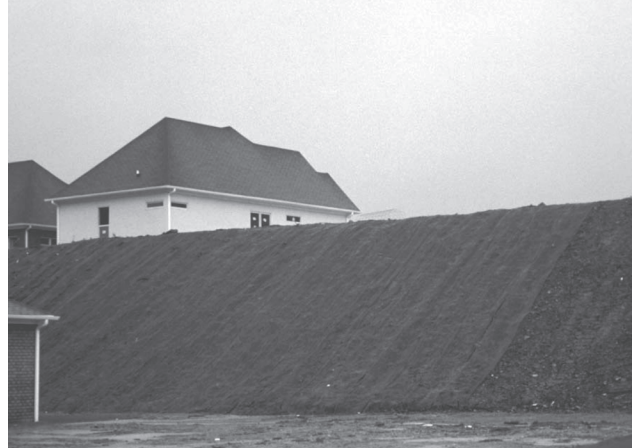
Slope being protected with netting after failure.
