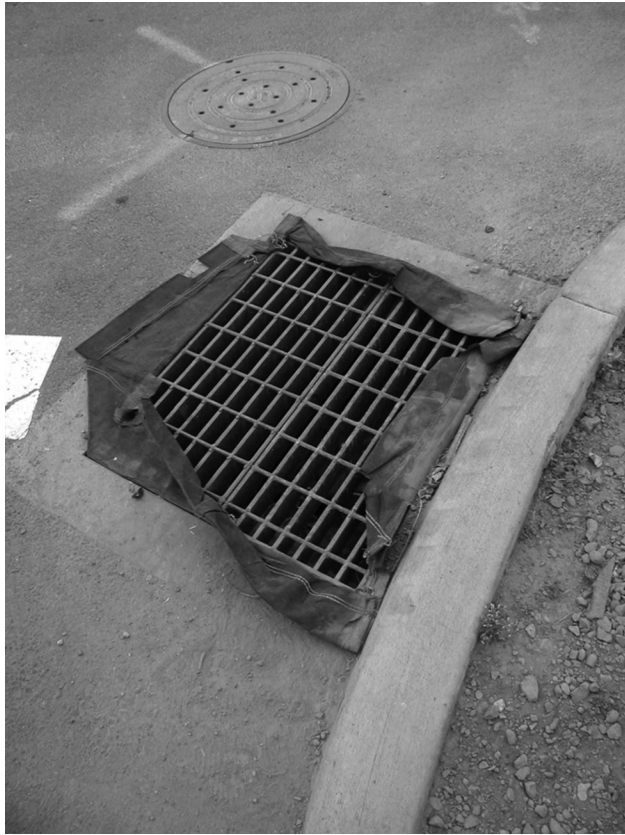
Temporary inlet filter fabric bag placed under inlet at redevelopment construction site.
