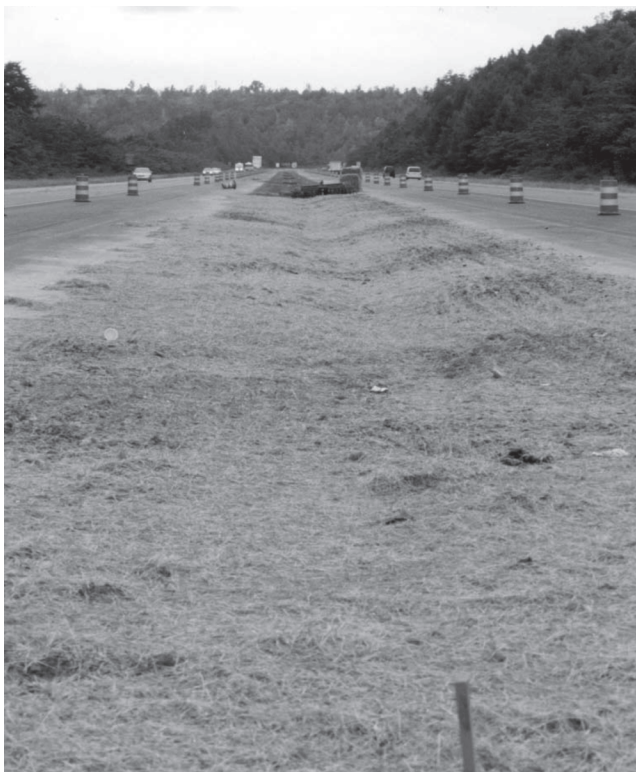
Heavy mulch at a median grass swale area.
