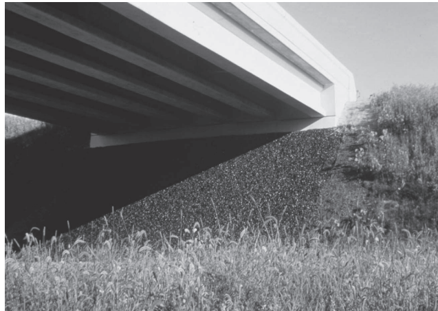
Asphaltic Slope Protection in Heavy Shade.
