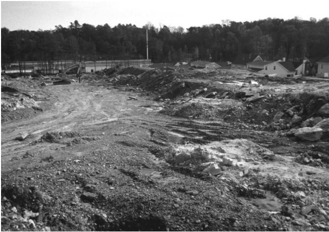
Large expanses of unprotected soils left exposed for long periods cause most of the sediment losses from construction sites.
