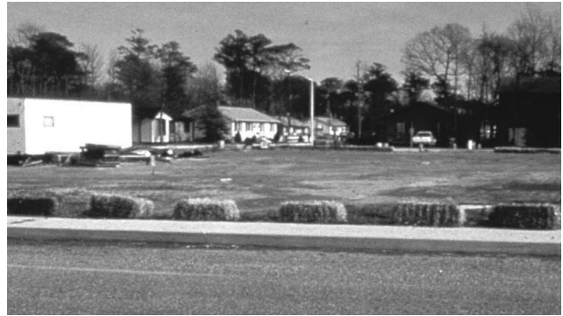
Education of erosion control contractors is mandatory (Maryland DNR, Earl Shaver, photo). These straw bales are located on the dashes on the site erosion control plan map designating the site boundary controls.
