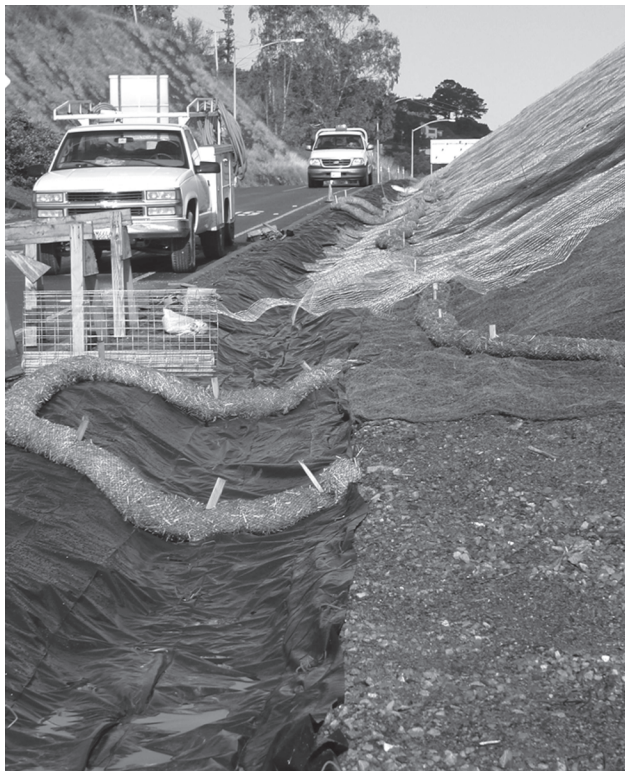
Plastic tarp, with coir logs, for a temporary liner.
