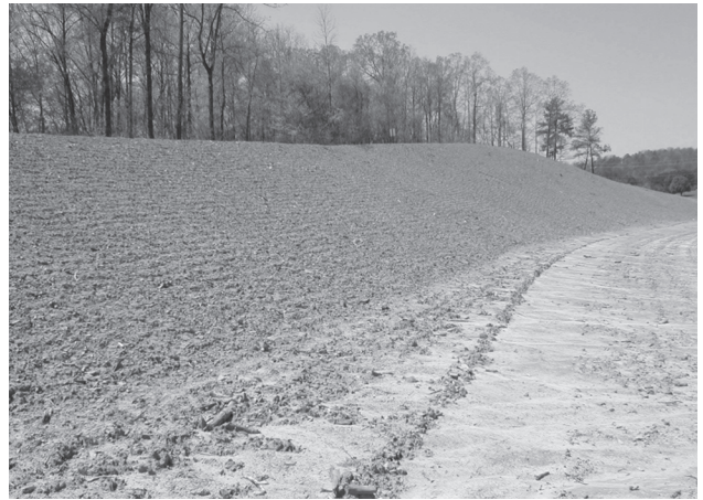
Roughened slope after compaction by Sheep's foot compactor.
