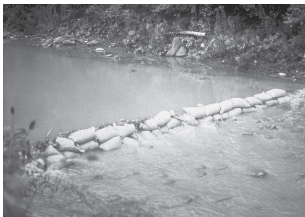
Check dam constructed of sand bags (Photograph by New York State Department of Transportation).
