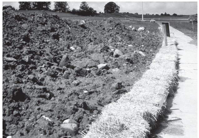
Hay bale barrier along edge of pavement.
