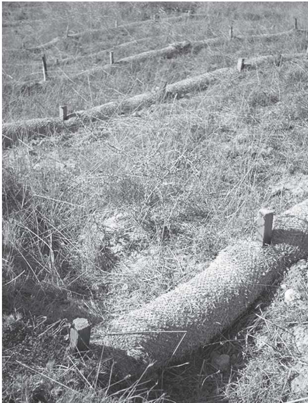
Coir (cocoanut fiber) rolls/logs and soil adhesives for slope stabilization project at Newport Beach, CA, wildlife refuge.
