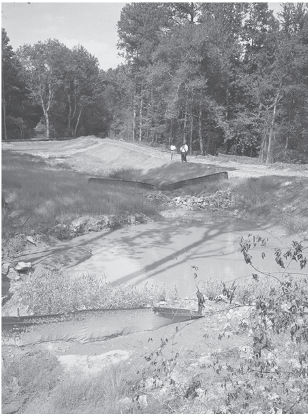
Series of small sediment ponds at a complex construction site (Atlanta, GA).
