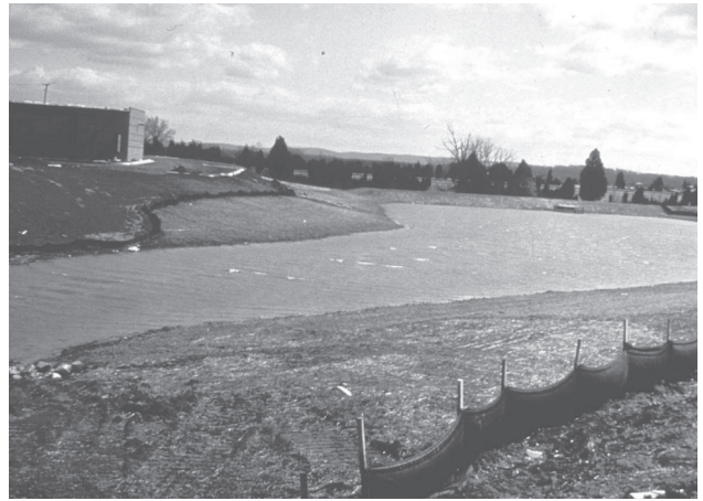
Permanent pond acting as sediment trap during final construction.
