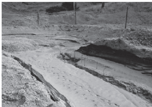
Pond inlet channel full of sediment and buried floc blocks (Source: Beca Carter Hollings & Ferner Ltd, undated).
