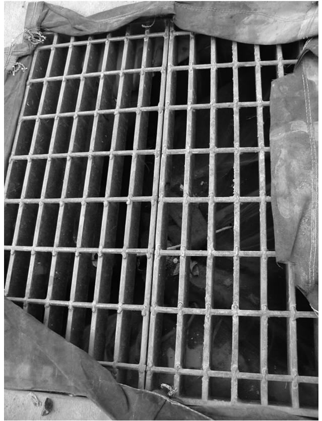
Temporary inlet filter fabric bag placed under inlet at redevelopment construction site.
