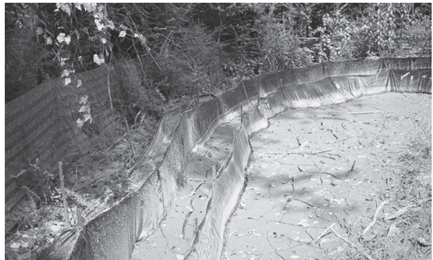
Bulk of sediment captured behind filter fence in ponded area.
