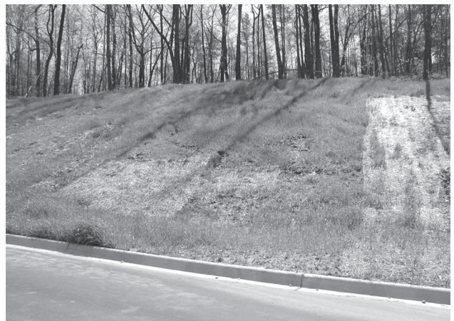
Netting used in areas to repair bank failure.
