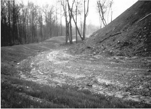
Large diversion berm and swale to divert water from downslope area at an abandoned mine site (SCS photo).
