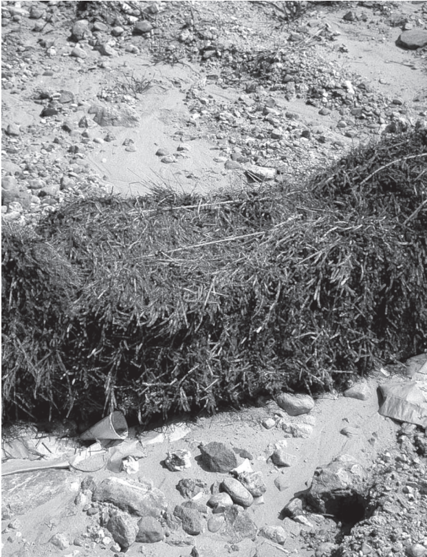
Sediment flowing under hay bale barrier.
