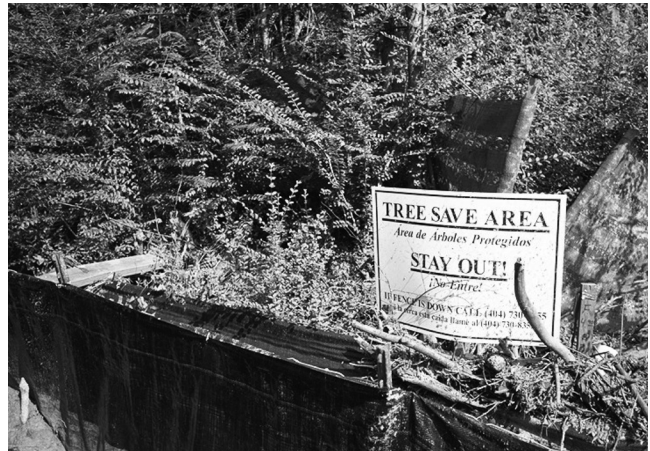
Barrier fencing setting outer limits of disturbance at construction site.
