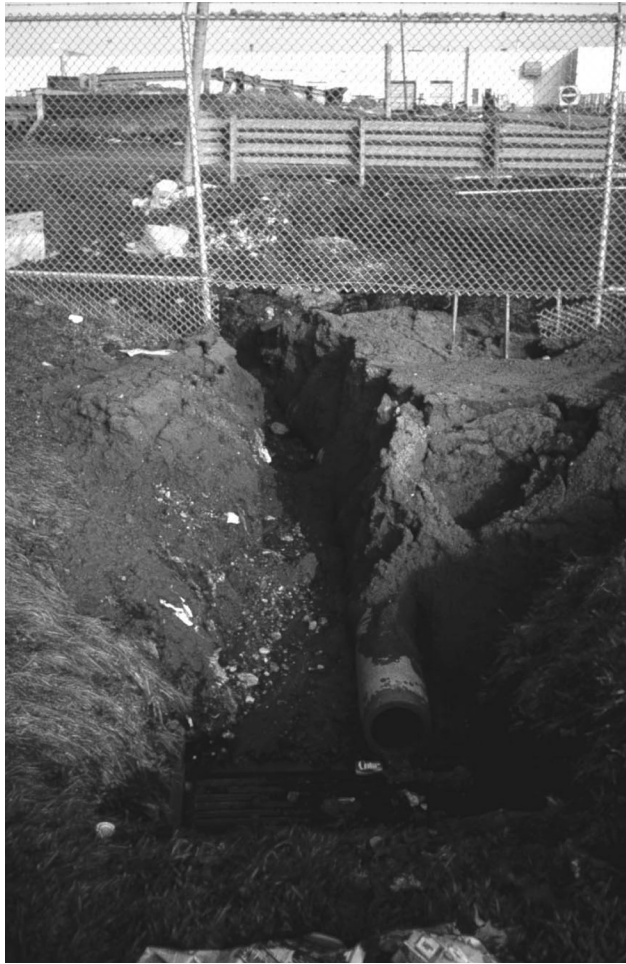
Poor grading directed runoff away from drain inlet and to the unprotected slope. Expensive repairs are now needed.
