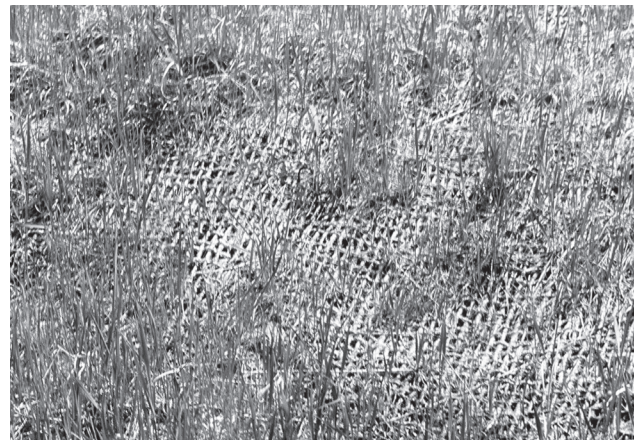
Netting over Mulch allowing Grass to Grow (Bill Morton photo).
