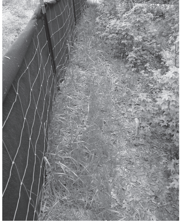
Filter fence along edge of property line (back side).
