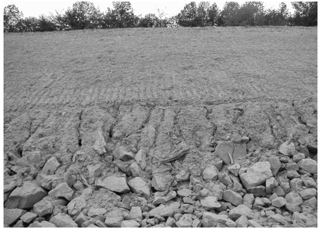
Inspections should require replacement of damaged mulch, or preferably the use of appropriate materials that are suitable for the site conditions.
