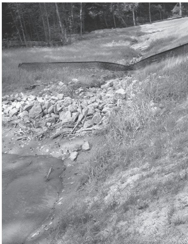
Check dams of rock and filter fabric.
