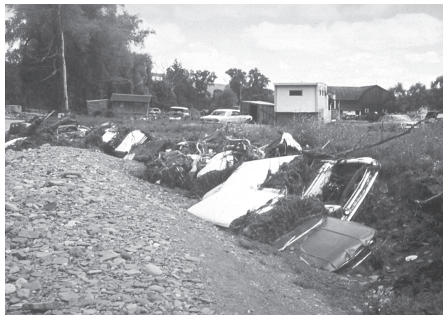
Scrap Metal Stream Stabilization.
