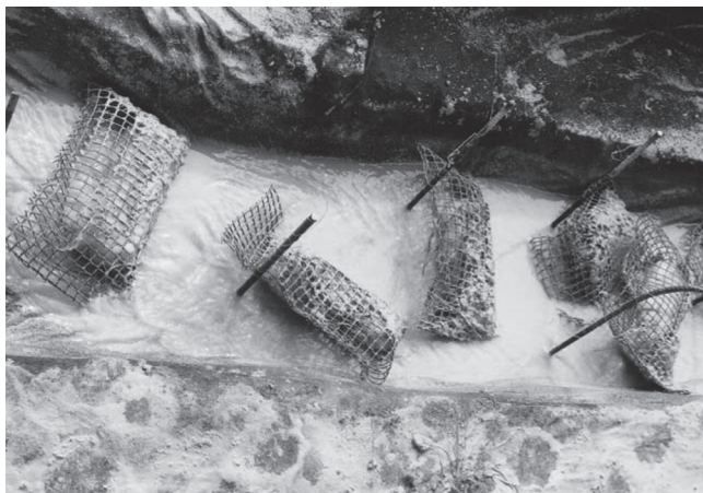
Floc blocks within channel between forebay and pond (Source: Beca Carter Hollings & Ferner Ltd, undated).
