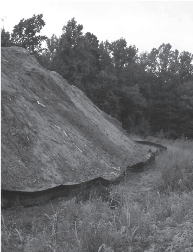
Caroline Sandel, UA student: silt fences around storage pile.
