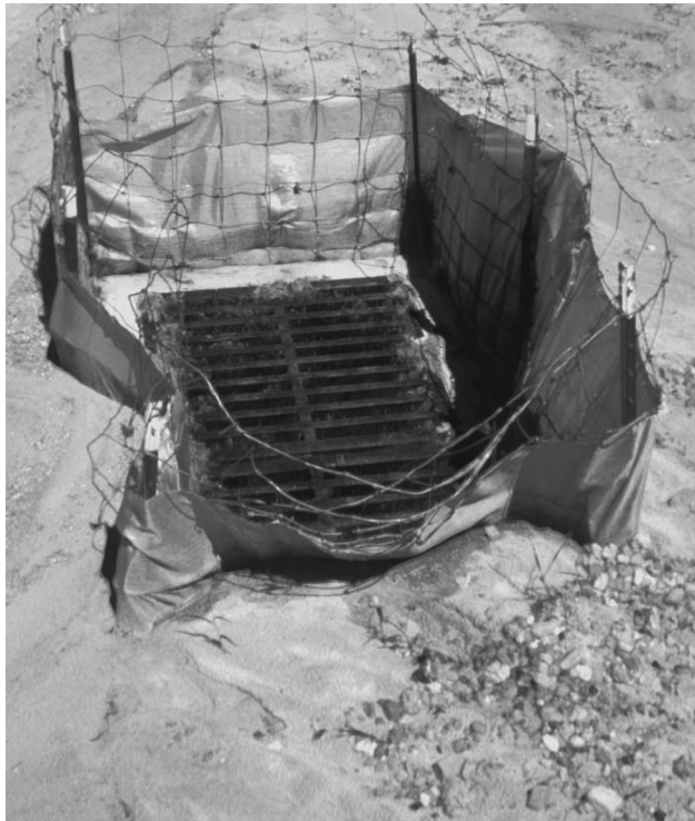
Large accumulation of debris surrounding filter fabric inlet barrier, requiring maintenance.
