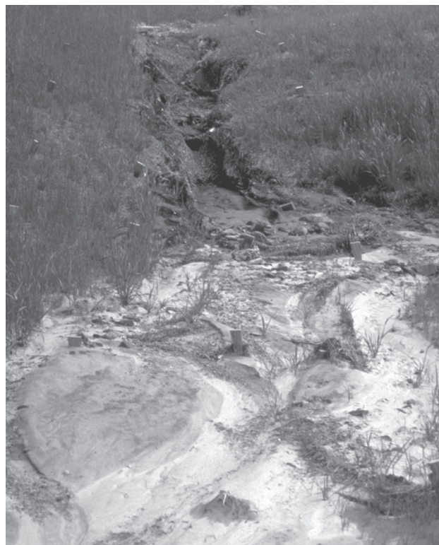
Gully erosion where concentrated flows formed, and down gradient deposition area in seeded construction area.
