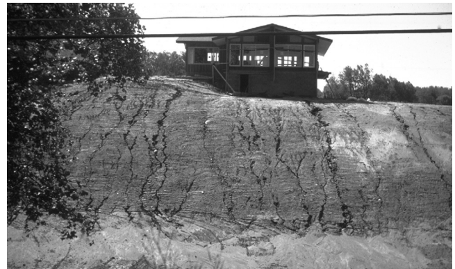
Erosion Threatening Homes (This home is actually being constructed on 12 feet of fill soil. The foundation footers are 14 feet below the groundline. Note the rills draining down to the drainage swale) (Photographs by D. Lake).
