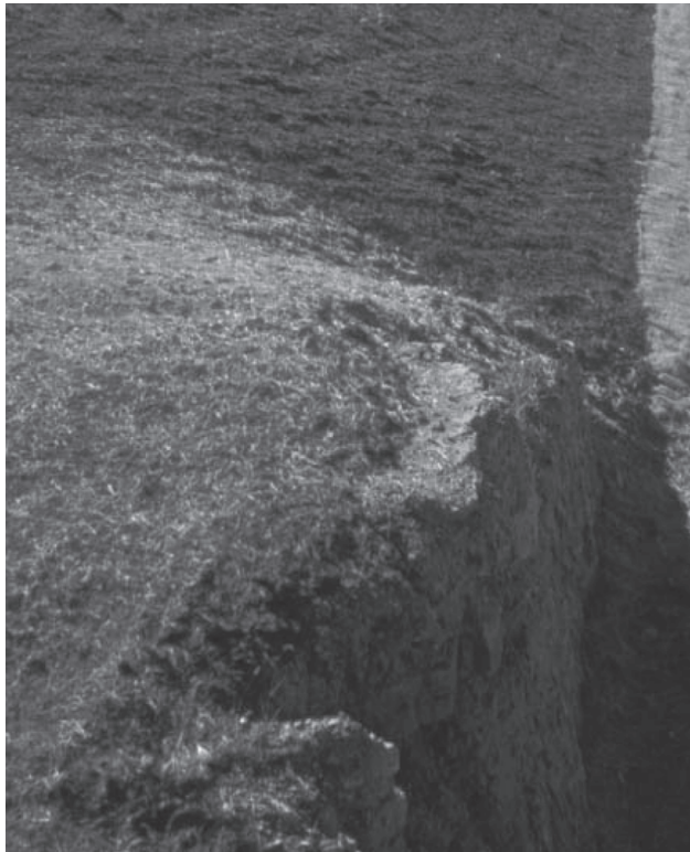
Reinforced liner along channel thalweg.
