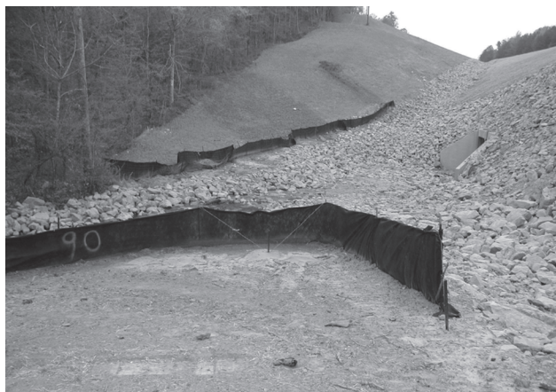
Evidence of underflow erosion beneath improperly installed filter fabric fence.
