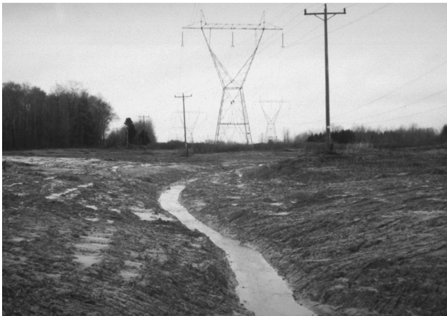
This exposed site is under a state shutdown order for destroying 2 acres of walleye spawning area in a nearby lake. 65 acres of the 70 acre site was stripped exposing soil containing 75–98 percent fines that could not settle out on site.
