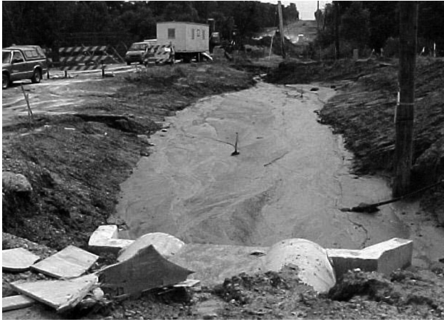
Drainage Ditch Filled with Construction Sediment (J. Voorhees) (Decreased drainage capacity causes increased flooding).
