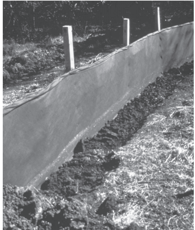
Layer of silt captured against bottom edge of newly installed filter fabric fence.
