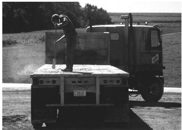
Vehicle being cleaned as it leaves a construction site to prevent debris from affecting public roads.
