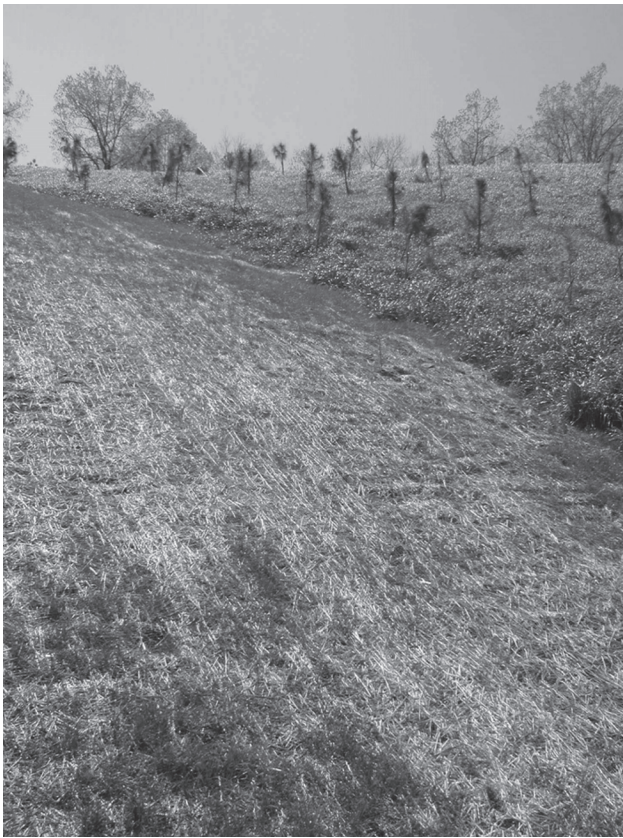
Netting used in areas to repair bank failure.
