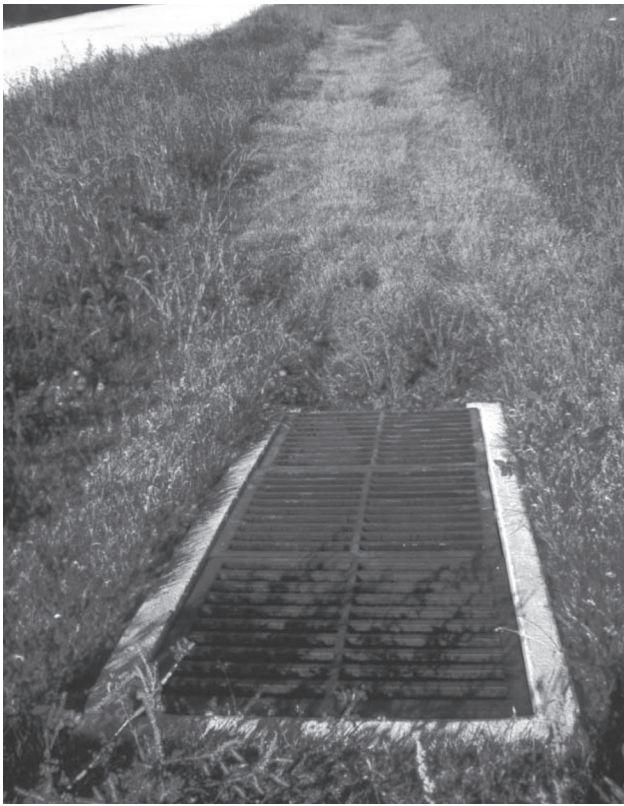
Sod placed along a channel bottom, with grass seed along the edges.
