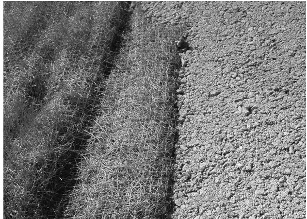
Netting and mulch along with cemented soil for roadside stabilization.
