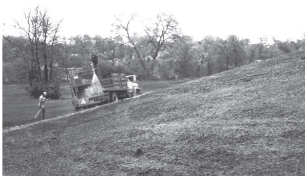
Hydroseeding, with mulch (SCS photo.)
