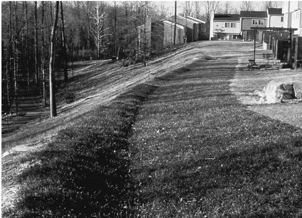
A small berm and sodded swale divert flows from newly graded and mulched hillside.
