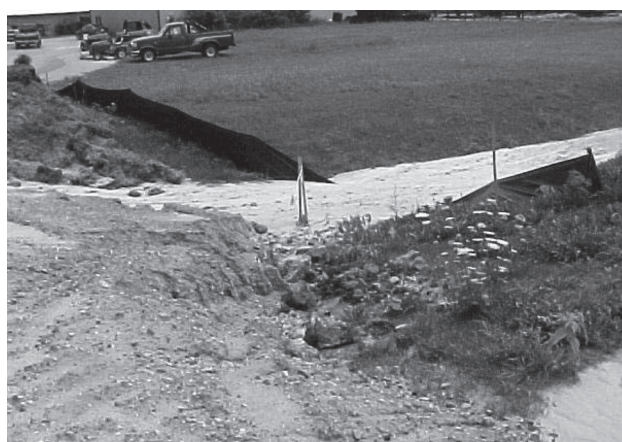
Same site as photo to left showing sediment load overtopping filter fabric fence due to lack of maintenance (J. Voorhees photo).
