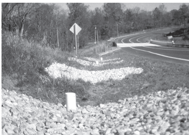
Series of riprap check dams spaced to cause ponding between dams (SCS photo).
