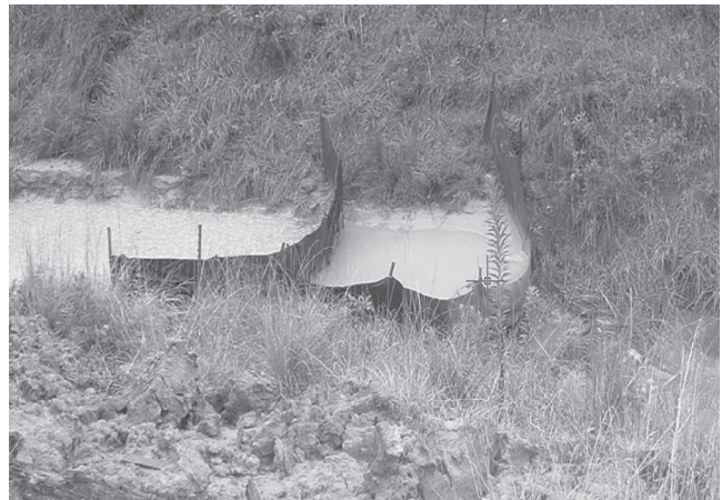
Jamie Lyles; UA student, filter fence check dams on a construction site.
