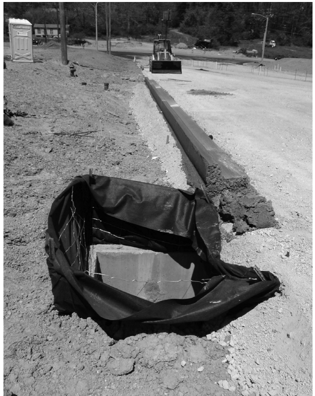
Damaged erosion controls need to be repaired or replaced as soon as possible.
