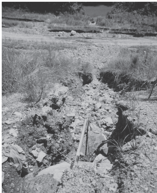
Large gully from concentrated flow (Bill Morton photo).
