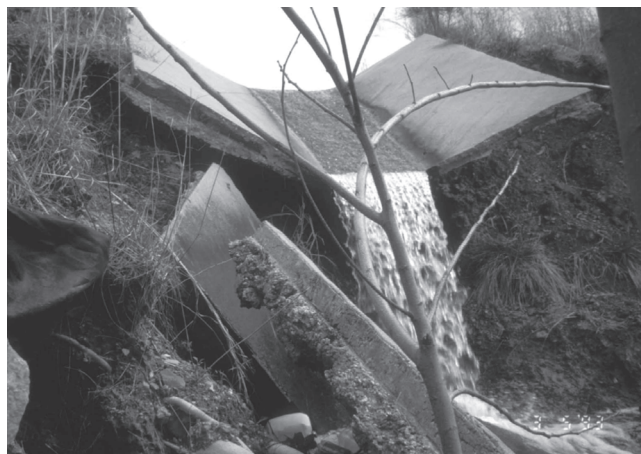
Failed concrete channel liner due to undercutting (photo by Mark Burford).
