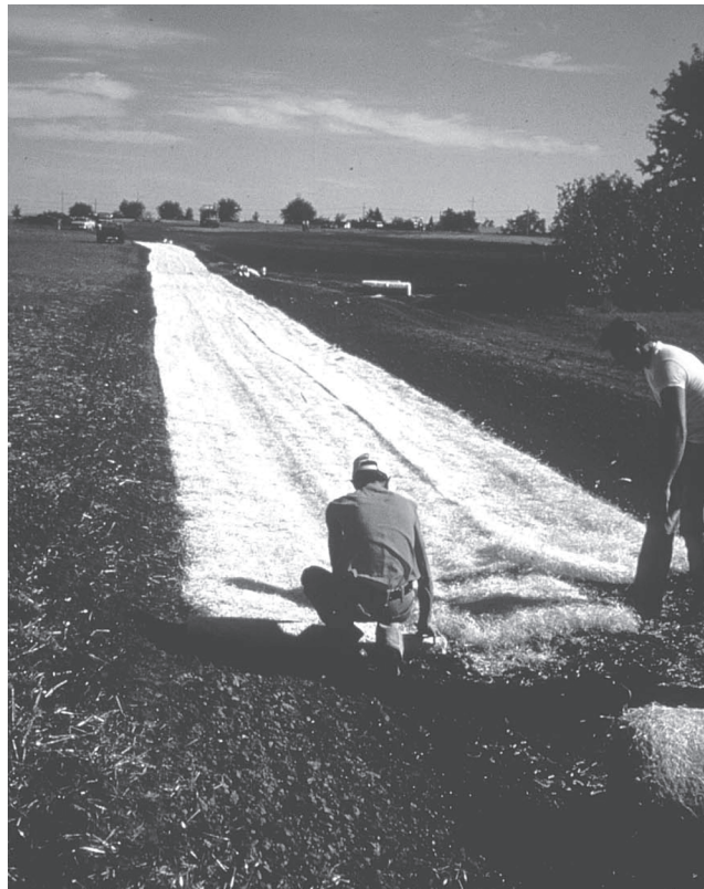
Installation of Erosion Control Matting (SCS photo).
