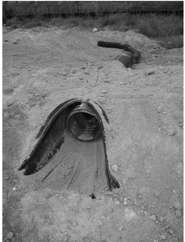
A diversion downslope pipe at a highway construction site (during installation) to prevent erosive flows from damaging an unprotected slope.
