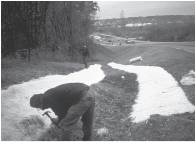
Installation of reinforced liner along thalweg of channel, with other material along sides (VA photo).
