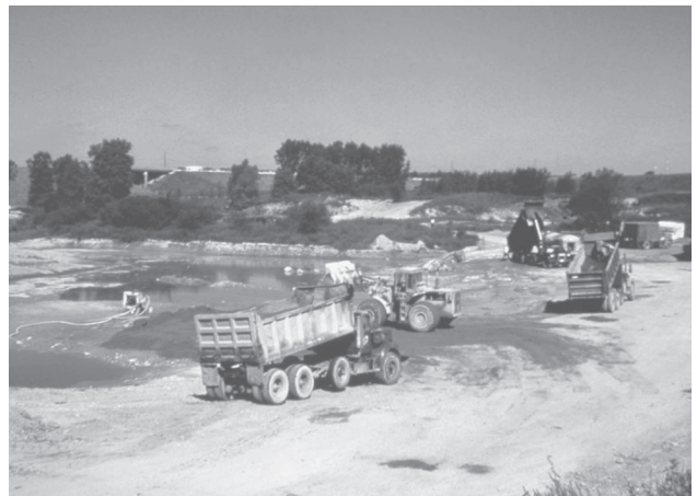
Temporary pond at highway construction site in area where hauling trucks are washed prior to re-entering roads (WI).
