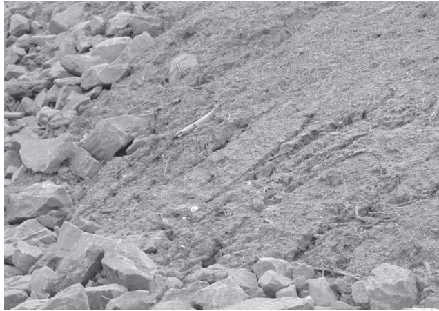
Failing Mulch on Slope above Rip Rap.
