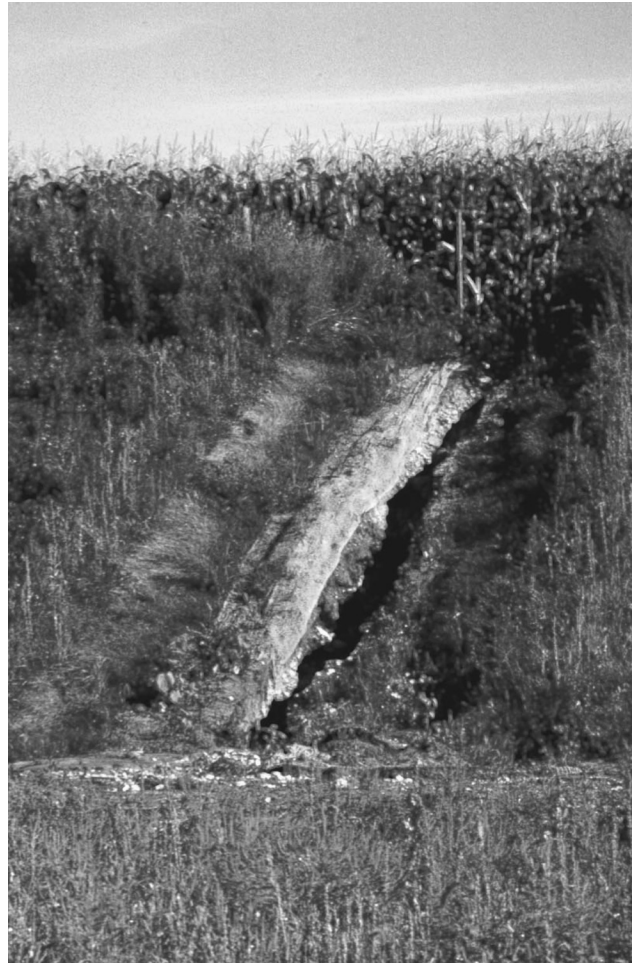
Another unfortunate example of poor grading allowing runoff to miss protected downslope channel.
