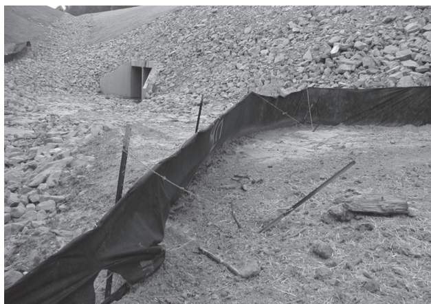
Holes in filter fabric fencing.
