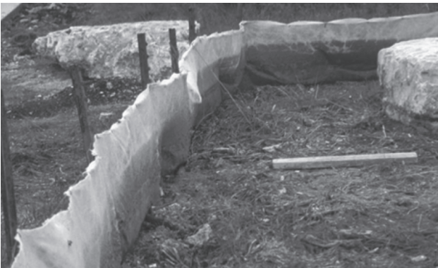
Ponded area sediment accumulation and smear of silt on fence.
