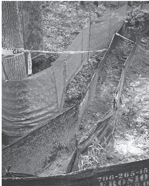
Multiple rows of filter fabric fences and tree barriers to mark edge of disturbed zone.
