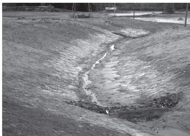
Typical check dams made of riprap.
