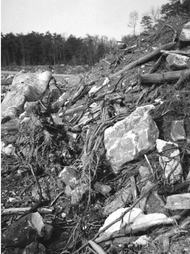
Buried debris and other material adversely affects soil structure and future drainage.
