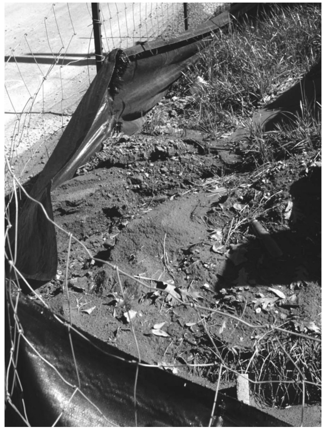
Inspections must enforce needed maintenance before failure. This silt fence is retaining massive amounts of sediment and is near its limit and needs to be maintained soon.
