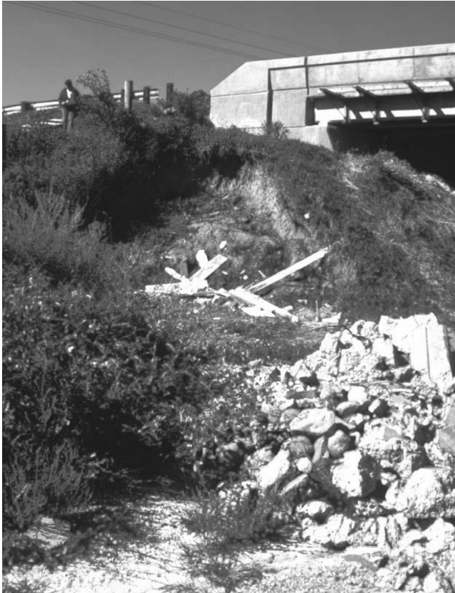
The lack of an appropriate diversion structure to safely drain water down sensitive slopes can cause much damage and sediment loss.
