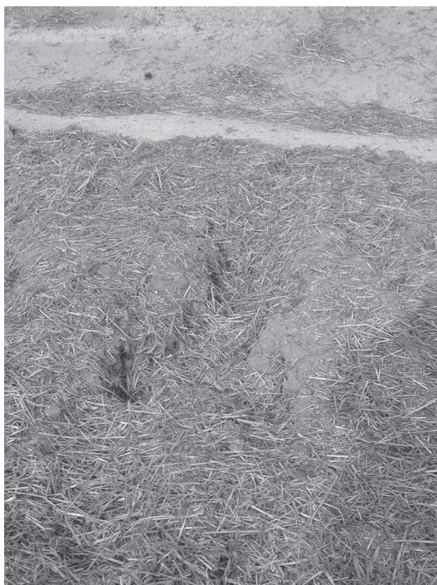
Straw mulch applied over previously eroded ground.
