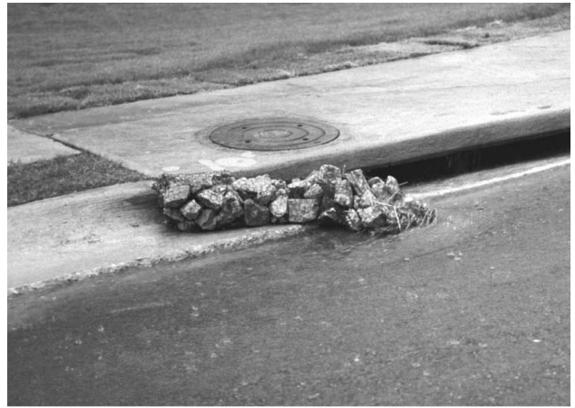
Netted stone barrier to attempt to divert bypassing gutter flows into inlet.
