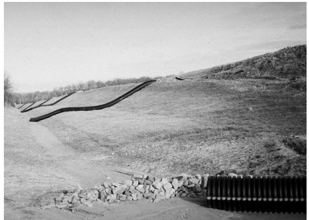
This photo of U.S. Route 1 being relocated around Dover, Delaware shows pipe slope drains that carry sediment laden runoff downslope to a collector swale. Note that the side slopes are graded and seeded as the work progresses to keep soil from washing down (Photograph by D. Lake).
