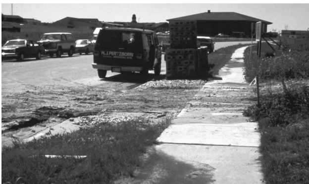
Excessive tracking due to insufficient or non-maintained graveled access needs to be corrected.
