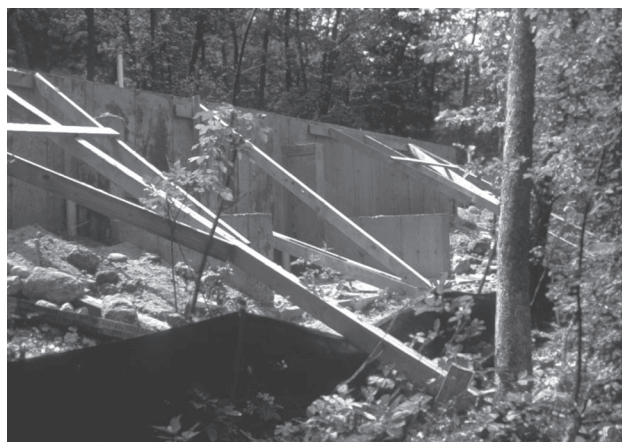
Filter fabric fence installed close to construction area.
