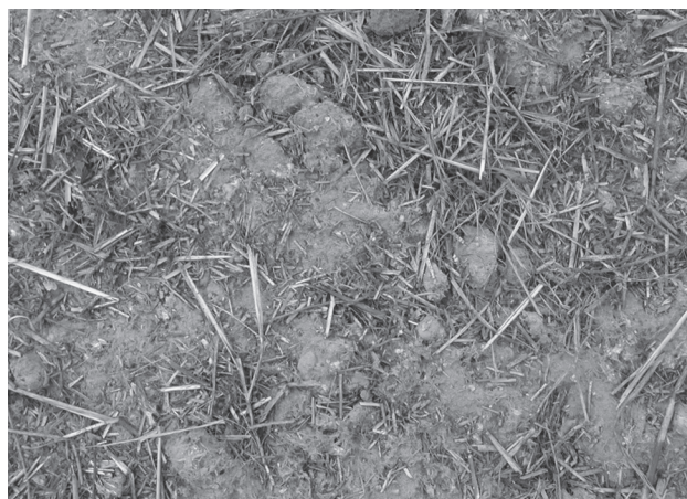
Thin straw mulch application showing poor coverage.
