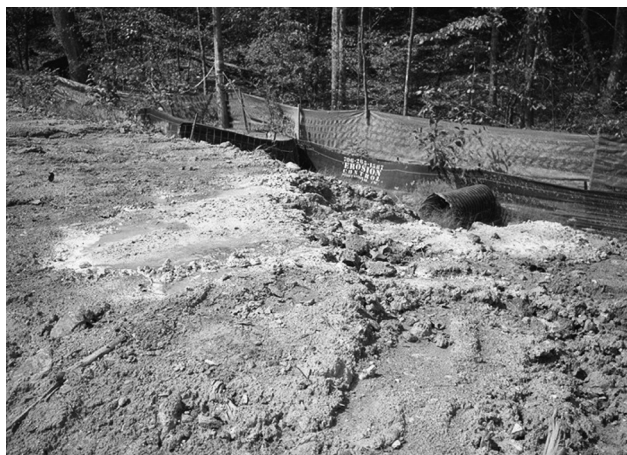
Improper waste concrete disposal.
