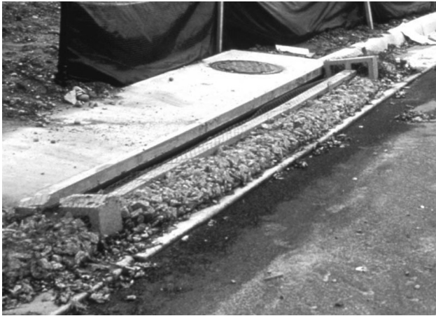
Older concrete block, lumber, and stone inlet barrier (historical SCS photo).
