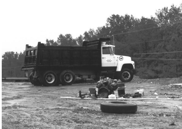
Engine repairs and other heavy equipment maintenance should not be allowed on construction sites, unless suitably protected from the elements.
