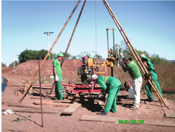
Fig. 12. Execution of the rotary drilling on the river Itacarambi possible to bridge the implementation outline of São Joao Mission.
