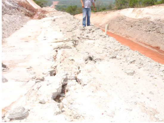
Fig. 8. Traction cracks in the berm slope of cut 25.
