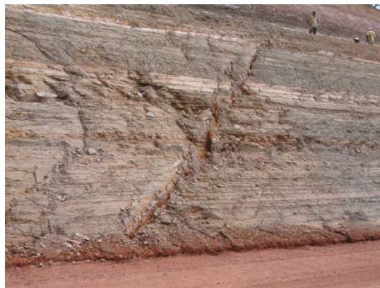
Fig. 4. View of the slope of cut 23.
