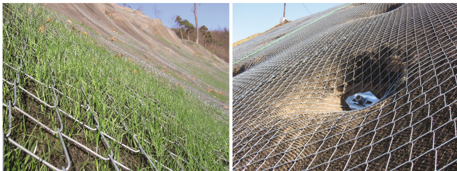
Fig. 1. TECCO® mesh and system spike plates
