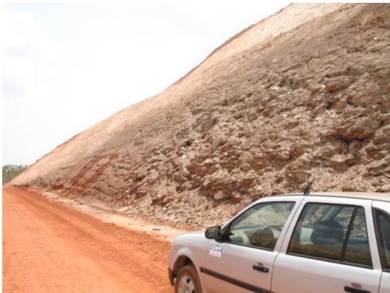
Fig. 6. Slope of cut 25 starting degradation process of slope.
