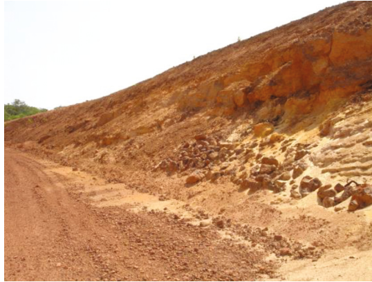
Fig. 2. General view of part of cut 16 with superficial erosion.
