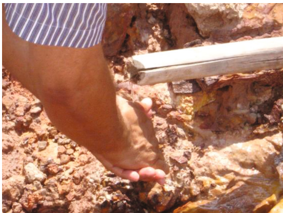
Fig. 11. Upwelling water in cut 25 slope.
