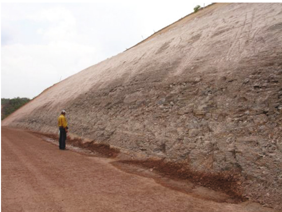
Fig. 13. Cut 31 (slope basis saturation).
