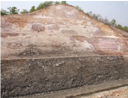
Fig. 5. Cut 25, still intact (September 2007).
