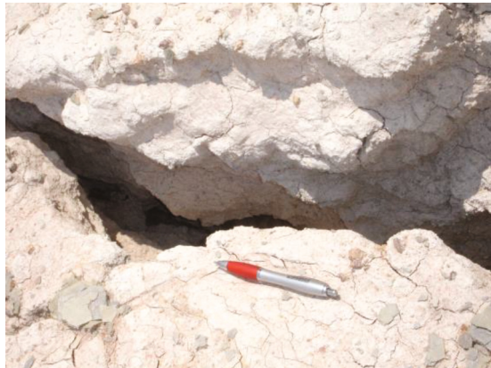
Fig. 9. Traction cracks on berm slope of cut 25.
