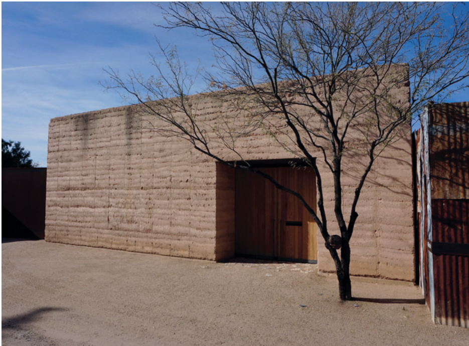
Figure 7.11 Architect Rick Joy, in Tucson, AZ, has helped to promote the use of rammed earth as a modern alternative as shown here in the façade of his firm's offices
