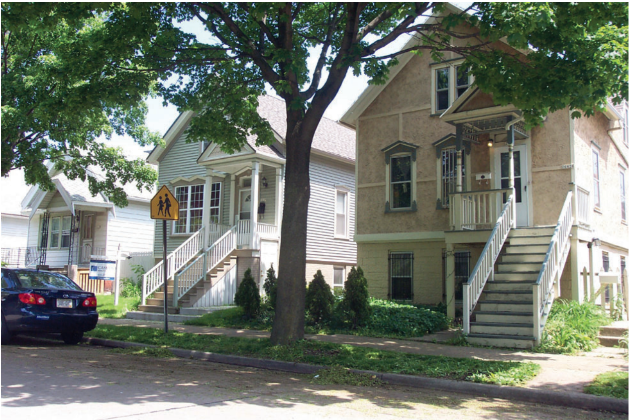
Figure 4.7 A Typical Street Of Polish Flats Elevated On High Basement Walls, Which Are Found In And Around Milwaukee, WI
