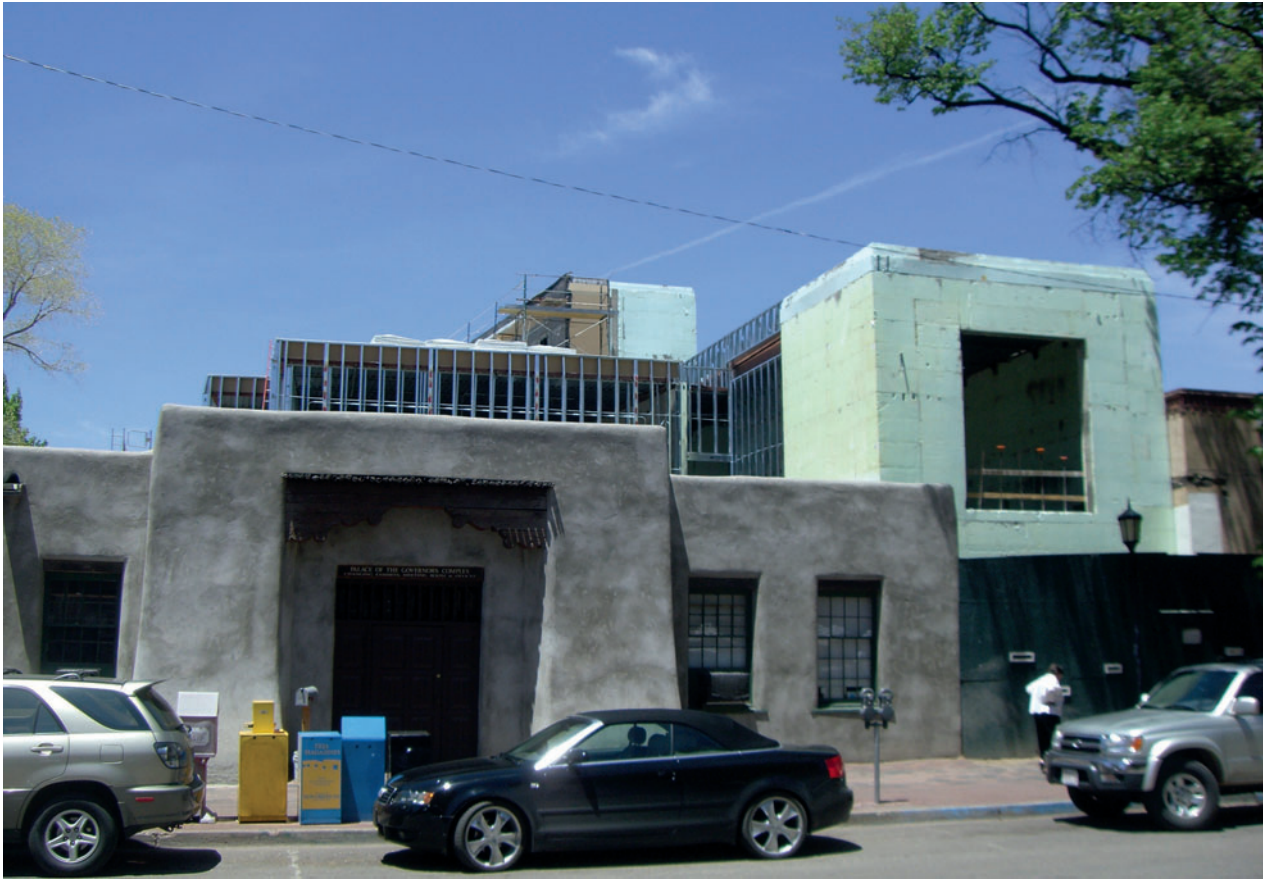
Figure 7.14 This Project In Santa Fe, NM, Shows How Current Construction Practices Of Steel Studs Covered By Rigid Insulation Form The Basis For Pseudo-Adobe Buildings In The Southwest
