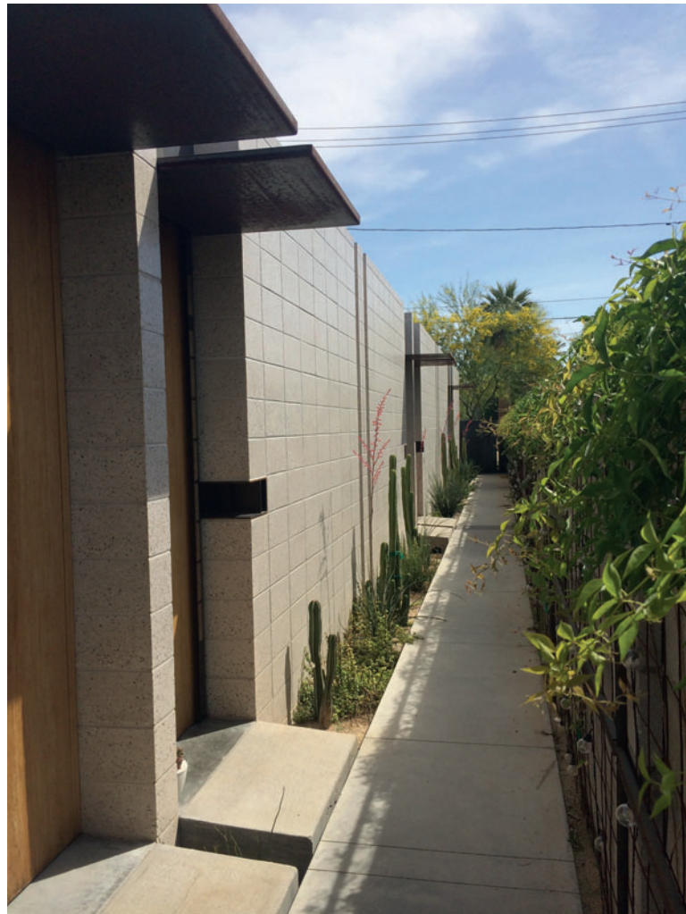
Figure 7.12 The Use Of Refined Concrete Block In The Walls Of These Modern Apartments Demonstrate How They Can Create An Elegant Exterior Surface
