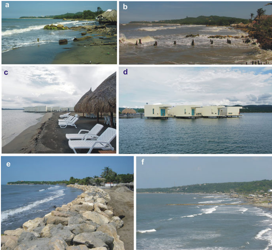
Fig. 1.5 Increasing beach erosion at Puerto Colombia, October 2012 (a) and 2013 (b) Flat beach of fine sediments with umbrellas and chairs (c) and human constructions (d) at Puerto Velero. Long seawall (e) and groins constructed (f) south of Punta Sabanilla
