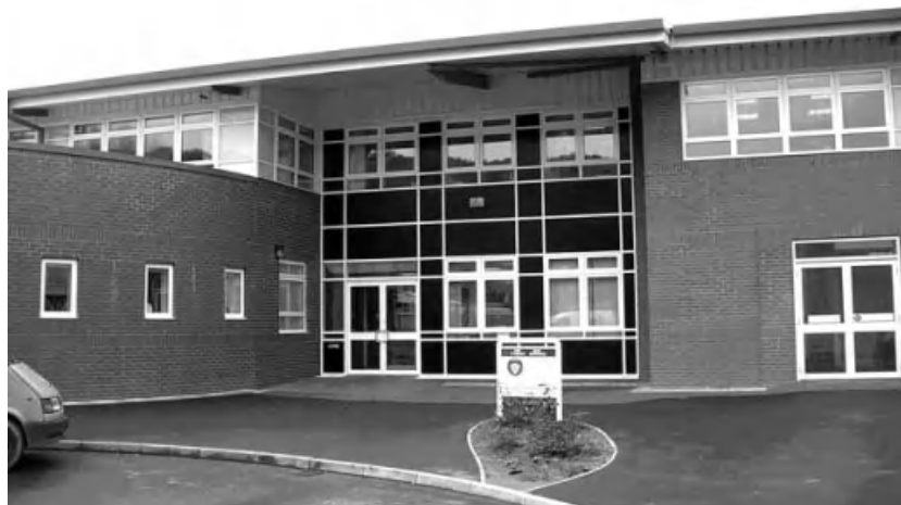
Figure 3.7 Unclear entrance to a PFI secondary school.
