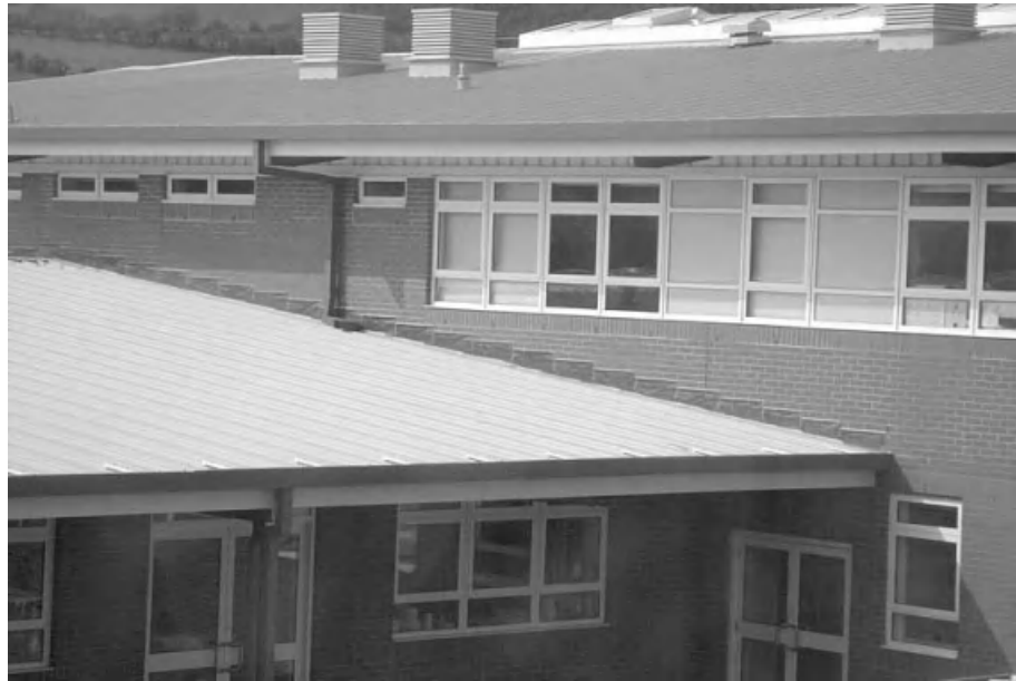
Figure 3.21 Typical metal roof covering of a PFI school.
