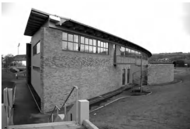
Figure 3.29 Traditionally procured school, which houses a flexible atrium space.
