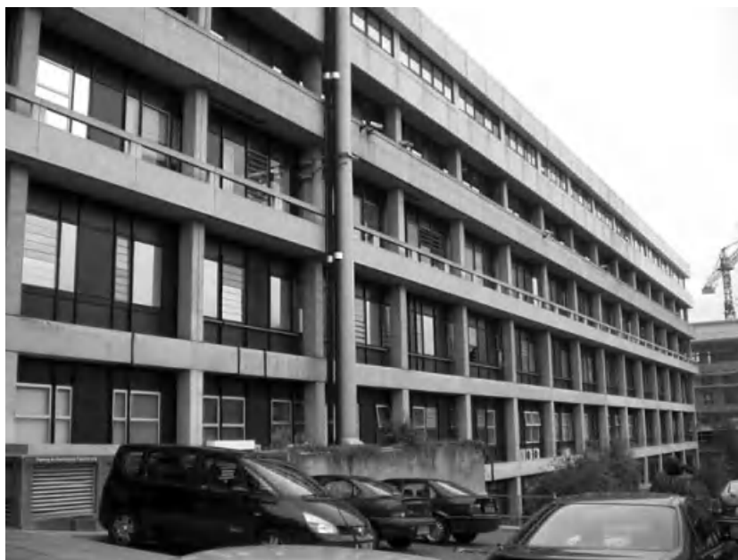
Figure 4.10 Traditionally procured hospital (circa 1970) with recent lightweight roof extension.
