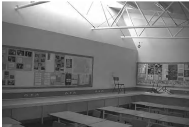
Figure 3.39 Clerestory windows provide daylighting to the back of a traditionally procured secondary classroom.
