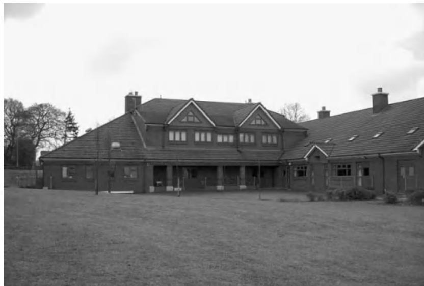
Figure 3.15 Boiler flues integrated into chimneys in a traditionally procured primary school.
