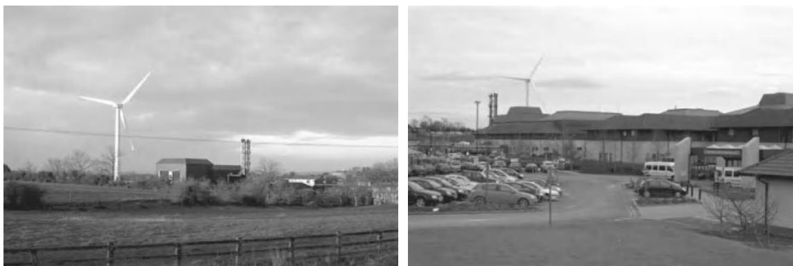
Figure 4.13 Antrim Hospital, Northern Ireland – retrofitted wind turbine.
