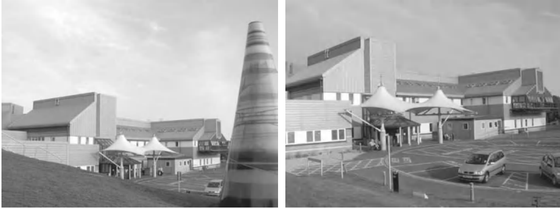
Figure 4.7 St Mary's Hospital, Isle of Wight (1990) – a low energy hospital. This figure is also reproduced in colour in the colour plate section.
