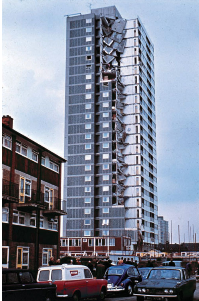
Figure 5.6 Ronan Point, London: after building collapse in May 1968. Reproduced with permission from RIBA Library Photographs Collection.
