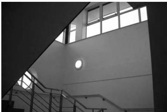
Figure 3.41 High-level opening lights to a stairwell with no easy means of opening.
