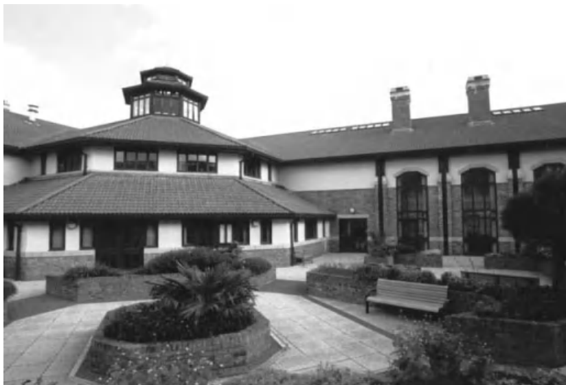
Figure 3.25 Traditional materials and detailing of a traditionally procured school. This figure is also reproduced in colour in the colour plate section.
