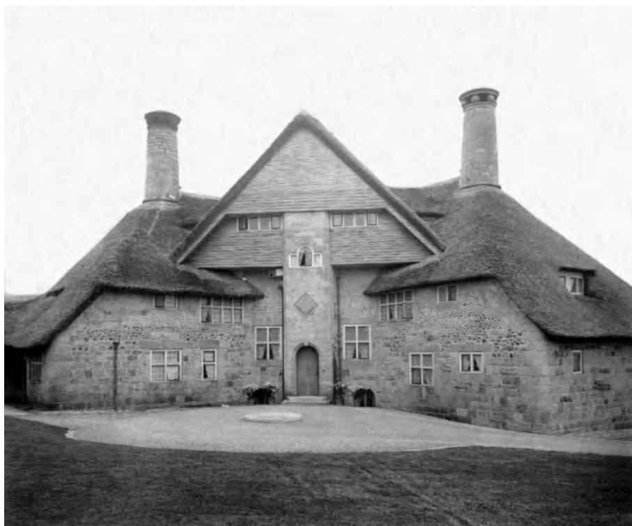
Figure 5.2 'The Barn', Exmouth – designed in 1896 by Edward Prior with local stone, pebbles from the beach and reed thatch. Reproduced with permission from RIBA Library Photographs Collection.
