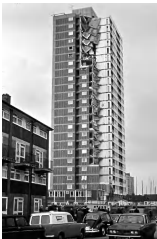
Figure 5.6 Ronan Point, London: after building collapse in May 1968. Reproduced with permission from RIBA Library Photographs Collection. This figure is also reproduced in colour in the colour plate section.
