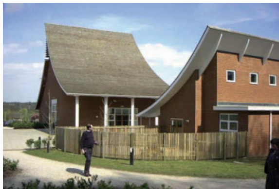
Figure 1.3 Imaginative buildings for young children – ‘ducks’. The boat and waves are primary schools. Copyright Joe Low/Architectural Association.
