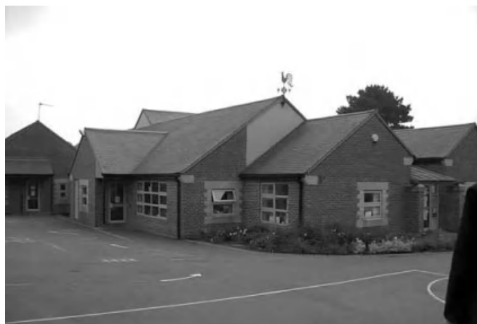
Figure 3.23 Typical concrete tile roof of a traditionally procured school.
