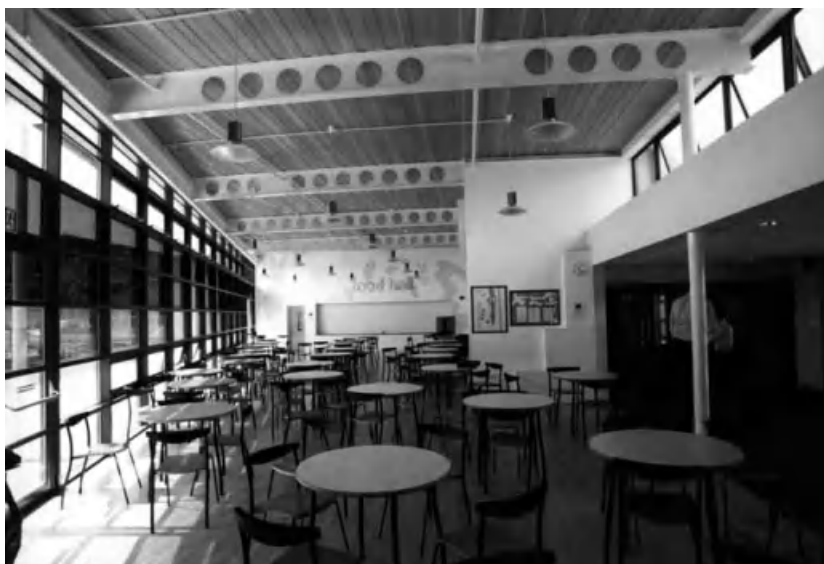
Figure 3.27 Lightweight materials and acoustically 'hard' surfaces in the restaurant of a PFI school.
