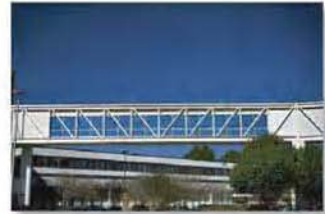
The forces in selected members of this Pratt truss can readily be determined using the method of sections.
