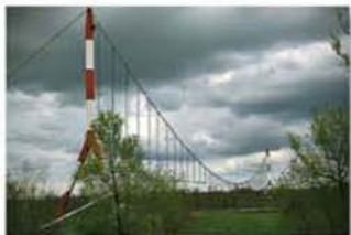
The cable and suspenders are used to support the uniform load of a gas pipe which crosses the river.
