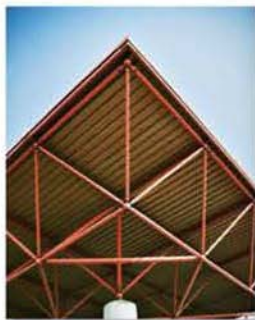
Typical roof-supporting space truss. Notice the use of ball-and-socket joints for the connections
