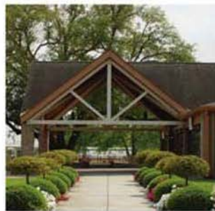
The forces in the members of this simple roof truss can be determined using the method of joints.
