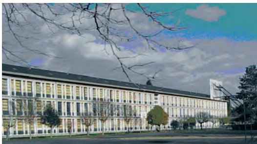
Figure 1.11 REVIVAL building Lycée Chevrolier, Angers, France: Built in 1958 of pre-cast concrete construction with dry lining and poorly fitting metal windows, it had very high infiltration rates before refurbishment
