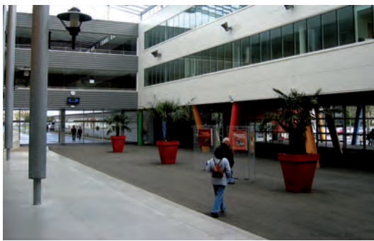
Figure 1.20 The new wing and atrium built as part of the Lycée Chevrollier (Angers, France) refurbishment. The old wing is on the right behind the retrofit shading
