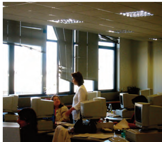
Figure 5.14 Office in Athens where internal louvres interfere with the opening windows and ventilation. A REVIVAL project before refurbishment
