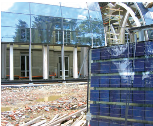
Figure 13.7 Exterior view of greenhouse during construction
