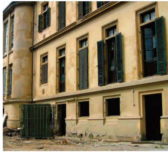
Figure 5.11 The traditional louvred shutters on the south facade retained as shading devices for the Meyer Hospital refurbishment, a REVIVAL project
