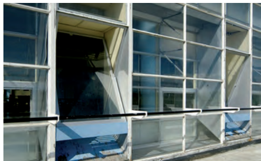
Figure 6.1 Wallesey School by Morgan in 1967, set out to be self sufficient in energy, combining a double skin south facade with highly insulated thermal mass
