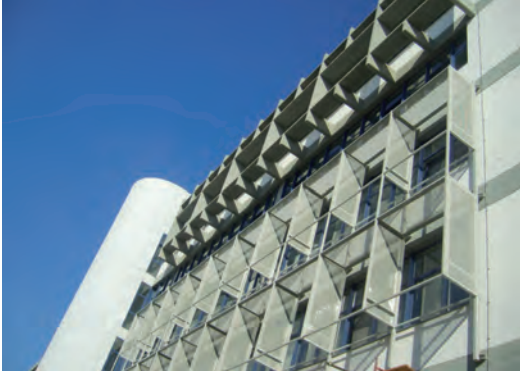
Figure 12.2 Newly fitted vertical and horizontal shading devices on WSW elevation on floors 2 and 3 with original concrete brise soleil on upper floors. Material is grey painted perforated steel to give the best combination of diffuse daylight and shading. Original internal louvre blinds shown on the right
