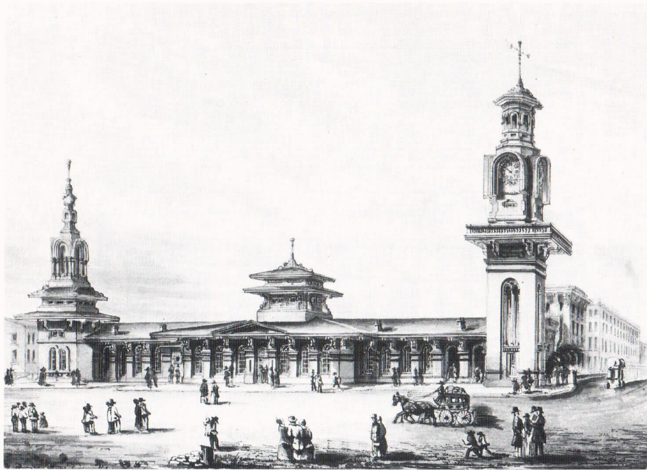
65 Henry Austin: New Haven Railroad Station, Connecticut, 1848-49.
