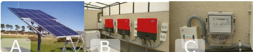
**Fig. 12** a Photovoltaic array on a rooftop, b balance of system (BoS) including an inverter, and c energy meter, junction boxes, wiring, etc., mounted on a wall [29]
