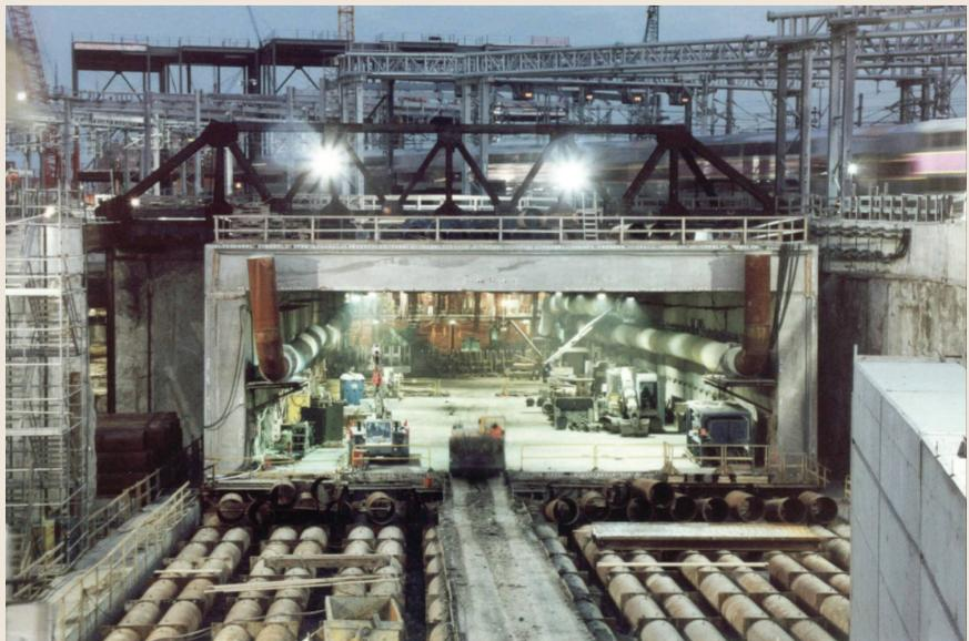
**FIGURE:** A view of the rear end of the tunnel box being jacked into place for the eastbound lanes of I-90 below the railroad tracks in Boston. A train is visible, passing over top of the tunnel. This jacked tunnel box was 36 feet high, 79 feet wide, and 379 feet long, and weighed approximately 32,000 tons. Used with the permission of the Massachusetts Turnpike Authority.
