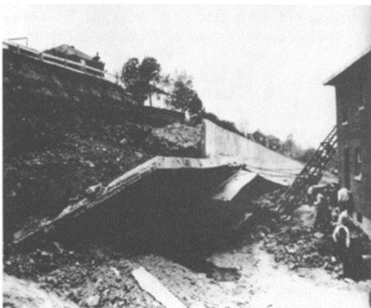
FIG. 1. Reinforced concrete cantilever retaining wall sections that failed during placement and compaction of backfill.
