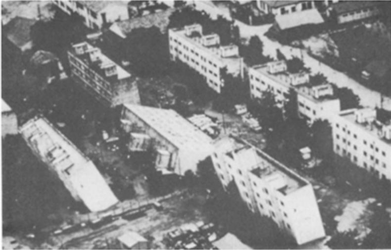
FIG. 1. Liquefaction of soil and collapse of buildings at Niigata, Japan, 1964.
