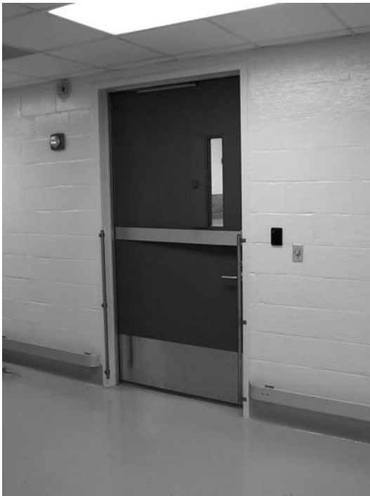
Fig. 9-4 Picture of an animal facility corridor illustrating guard rails installed approximately 6" off the floor. Note also the crash rail on the door and the vertical door-frame guards.
