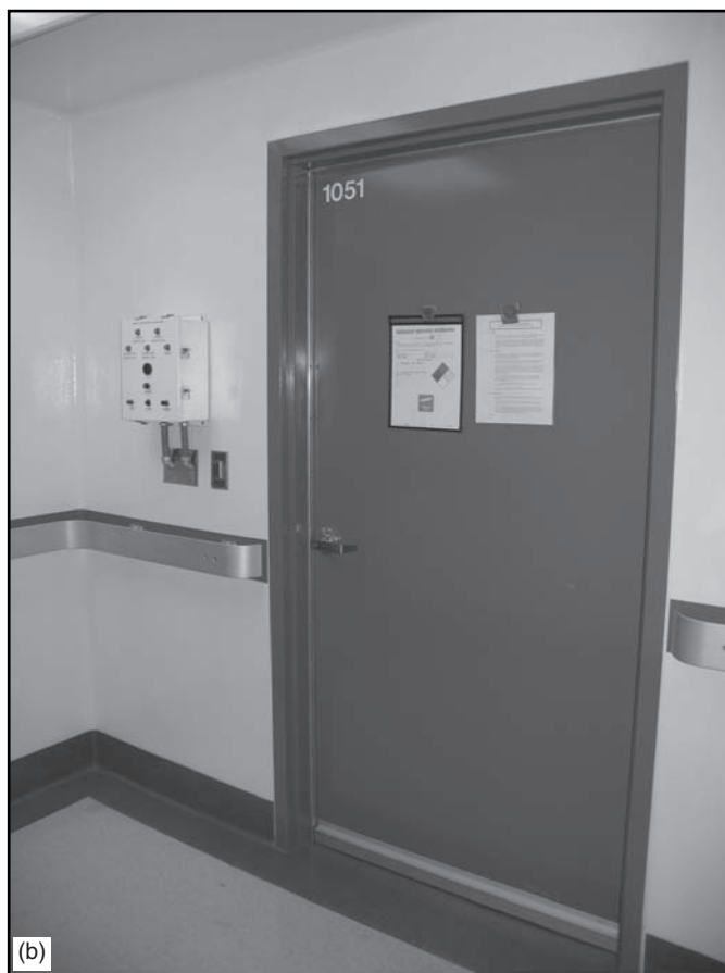
Fig. 19-4 (b) Entrance to gas cylinder storage room. This room is conveniently located outside of the surgery suite and easily accessible by delivery personnel. The alarm adjacent to the door is located in an area of high traffic and visibility, to alert personnel when a gas supply cylinder has been depleted and the manifold needs to be switched to obtain gas from a full cylinder or cylinder replacement is necessary.
