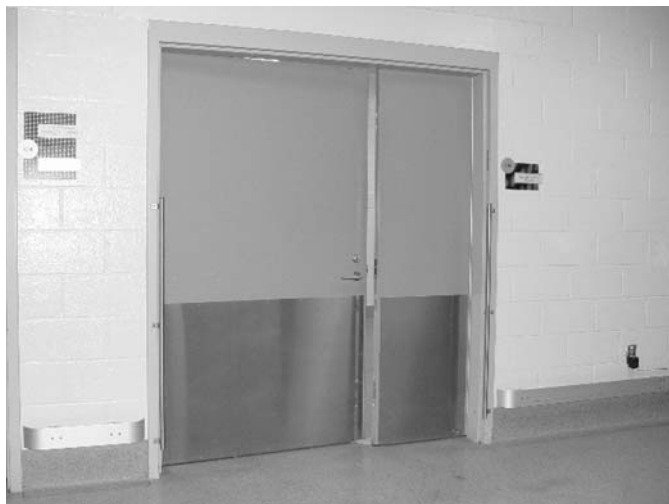
Fig. 12-1 Dual door entry for a bulk feed and bedding storage area used to facilitate the passage of materials on pallets. The paired doors open inward and are each 84 inches high with one measuring 48 inches and the other 24 inches in width.
