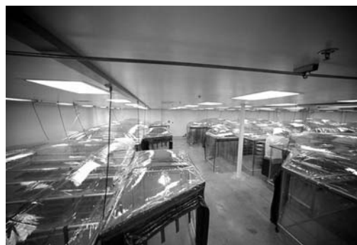
Fig. 34-2 Multiple HEPA-filtered mass air displacement flexible film “rooms” inside a large room. Figure courtesy of bioBubble, Inc.
