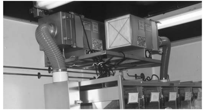
Fig. 34-6 Supply and exhaust filter/fan modules for a ventilated rack sitting on a wall-mounted shelf.
