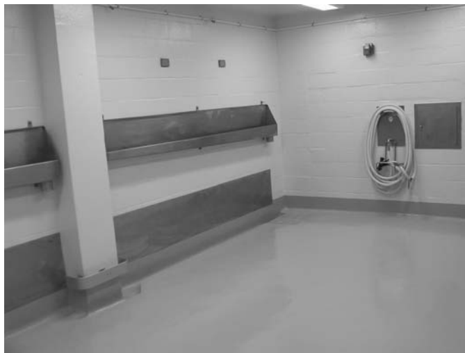
Fig. 21-2 Interior of a NHP housing room.
