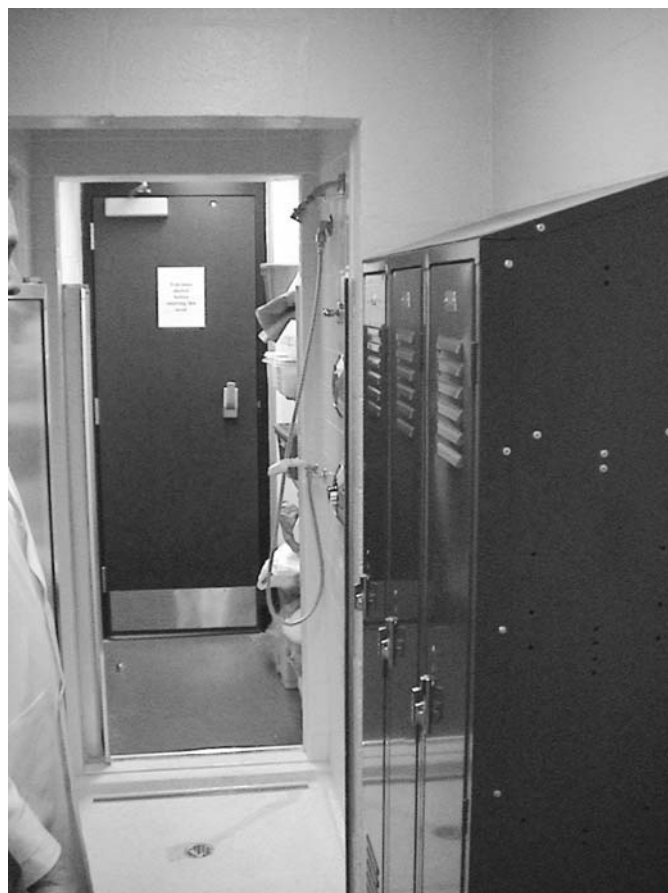
Fig. 24-3 (Continued) (b) Photograph of such a dressing/shower room looking into the entry portion with lockers. Note the closed shower door. (c) The same view as (b) with the shower doors open, looking through to the door leading into the containment area.
