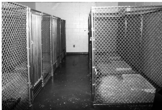
Fig. 22-1 Chain-link runs within an animal housing room with a single, capped floor drain. The runs are 4' × 6' in dimension, with the 6'-long back panel oriented along the side wall of the room to provide a larger aisle between runs. The runs are equipped with fiberglass resting boards and direct bedding consisting of wood shavings.
