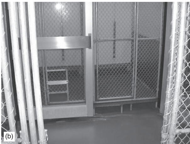
Fig. 15-16 Cubicles with fixed raised floors: (a) two adjacent large animal cubicle pens with different types of raised floors, fiberglass T-bar slats and vinyl-coated expanded metal; (b) raised vinyl-coated expanded metal floor showing a stainless-steel leg of the stainless-steel frame that supports the raised floor.
