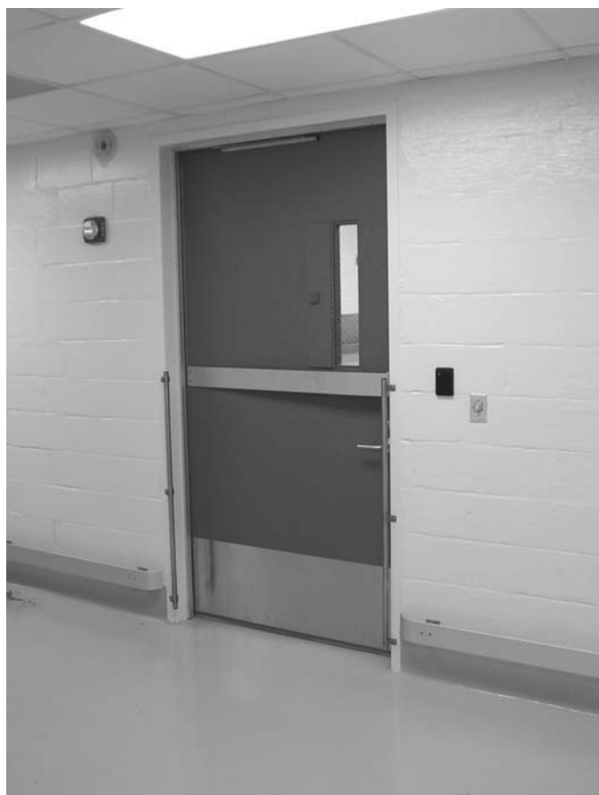
Fig. 21-1 Exterior view of animal room doorway.
