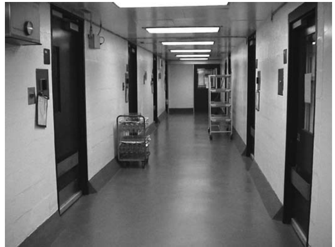
Fig. 9-5 Picture of an animal facility corridor illustrating 6" x 6" sloped bases designed to protect the walls. The bottle cart and cage rack show how the base serves to protect the wall. They also show how the low-mounted crash rail in Figure 9-3 would effectively protect the wall from being hit by either short or tall carts.
