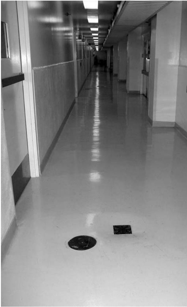
Fig. 23-4 Corridor drain and corresponding cleanout. Both the drain grate (right) and cleanout access cover (left) should be level with the floor surface.
