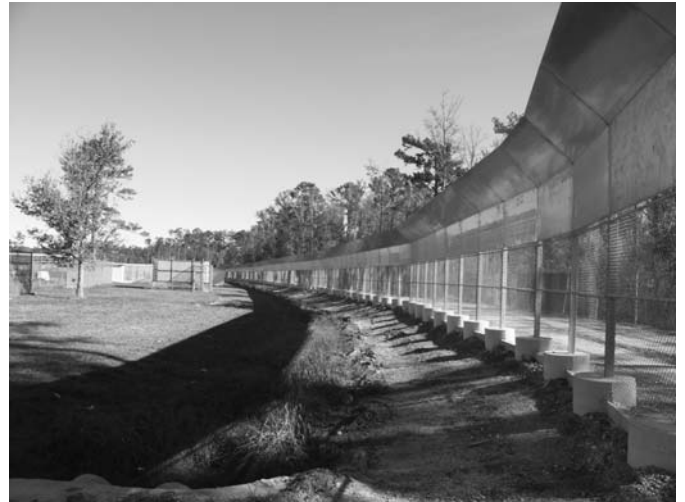
Fig. 21-11 Unscalable perimeter fence.
