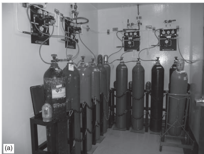
Fig. 19-4 (a) Gas cylinder storage. This automatic gas cylinder storage room is utilized for the bulk storage and source for building wide distribution of gasses (oxygen, nitrous oxide and carbon dioxide). These automatic switching gas manifolds allow serial connection of multiple gas cylinders to ensure that gas distribution is not interrupted.
