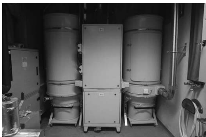
Fig. 31-18 Vacuum system for removing soiled bedding.
