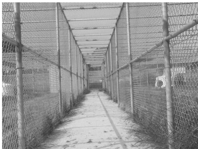
Fig. 21-24 Berm for separation of enclosures in divided field cages. Berms are used to separate enclosures that are in close proximity by directing wastewater runoff away from adjoining enclosures and preventing contact between animals. The photograph shows a concrete berm that is within a divided field cage and is 5 feet wide.
