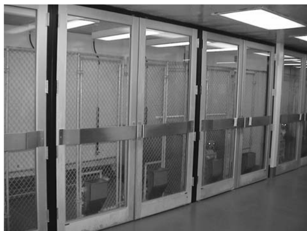
Fig. 15-18 A row of large animal cubicles with hinged doors. Dogs are housed in the end cubicles.
