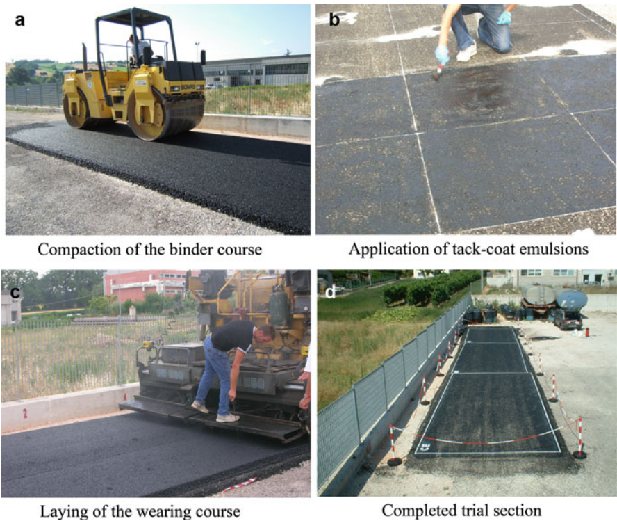
Fig. 6.9 Phases of trial section construction
