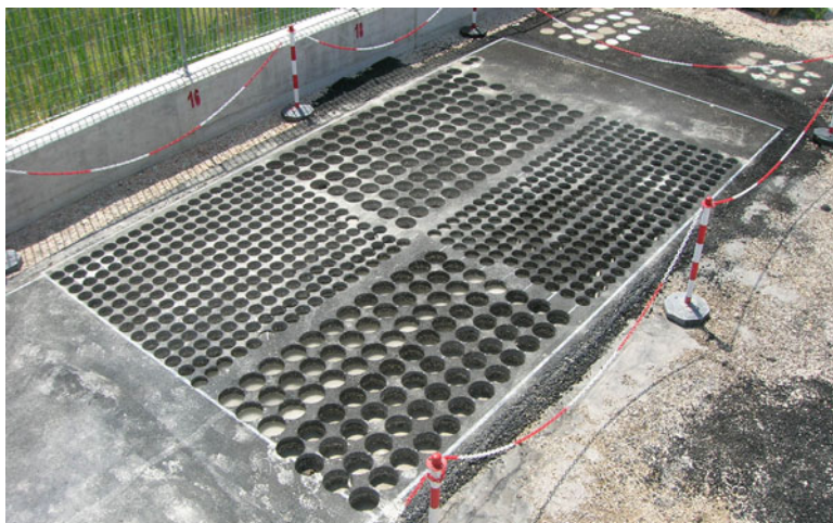
Fig. 6.10 Trial section after taking 100 and 150 mm cores from Pavement 1
