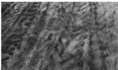
(a) Compacted soil used as sub-grade
