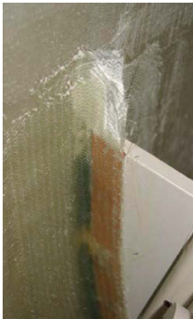
Figure 5 : A junction made by manual layered VTR reinforcement.
