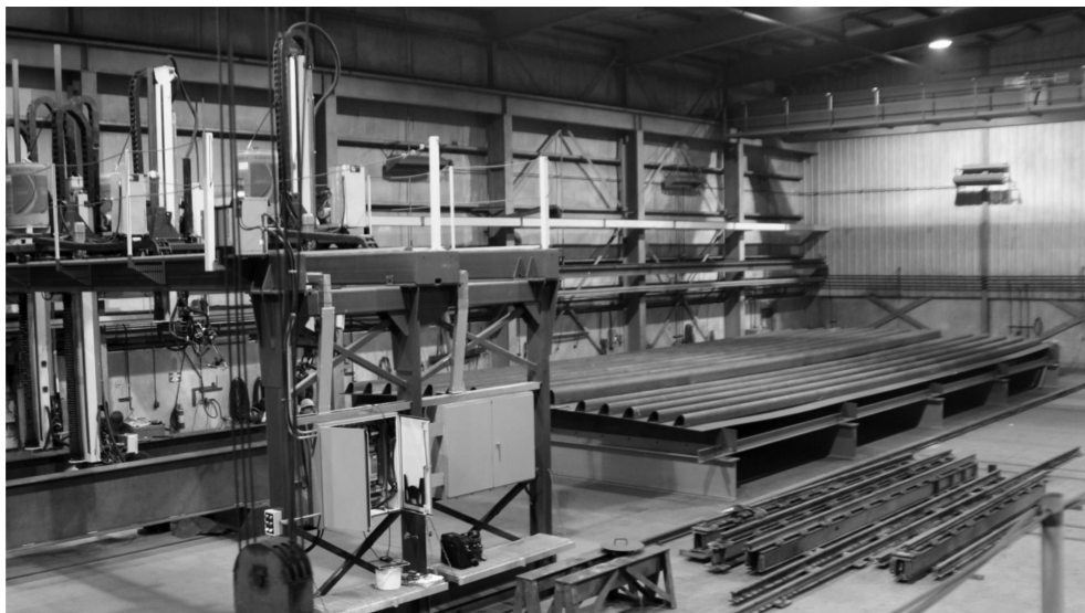
Figure 6. Partially fabricated deck section.
