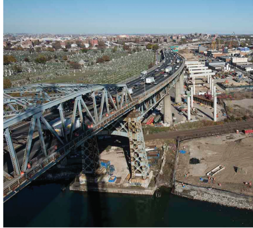
Figure 1. Existing Kosciuszko Bridge looking east into Queens with new Queens Approach substructure.
