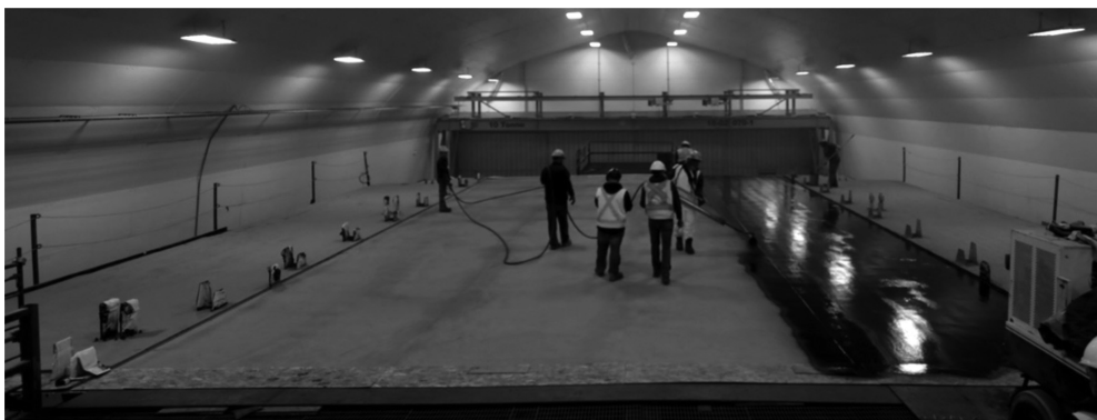
Figure 10. Segment in the painting tent.
