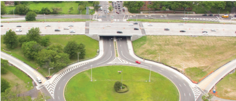
Figure 6. Replacement Belt Parkway Bridge over Rockaway Parkway (2013).
