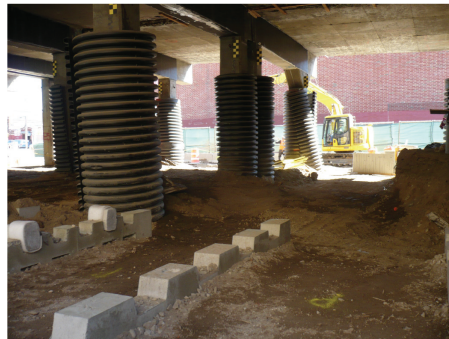
Figure 9. Fill placement under Meeker Avenue Viaduct with isolation sleeves around columns.
