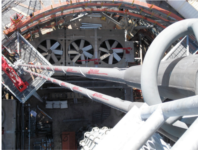
Figure 6. Fiber assemblies installed on roof structure.
