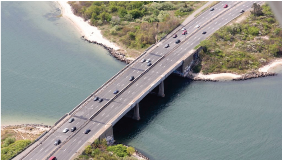
Figure 11. Original Belt Parkway Bridge over Gerritsen Inlet (2010).
