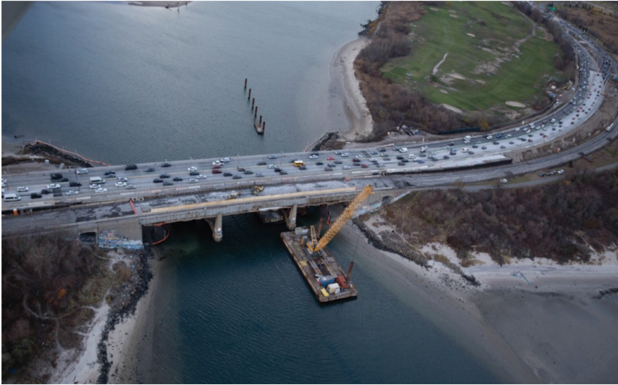
Figure 12. Replacement of Belt Parkway Bridge over Gerritsen Inlet—Stage 3 (January 2017).
