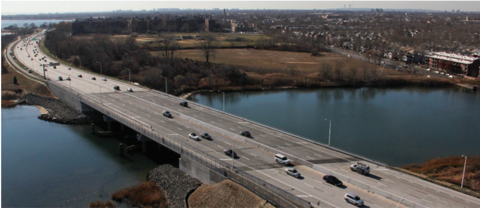
Figure 8. Replacement Belt Parkway Bridge over Fresh Creek Basin (2013).
