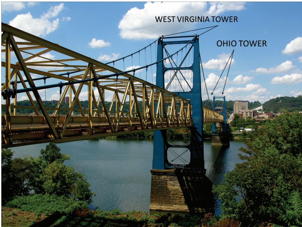
Figure 1. Elevation view of Market Street Bridge—looking west.
