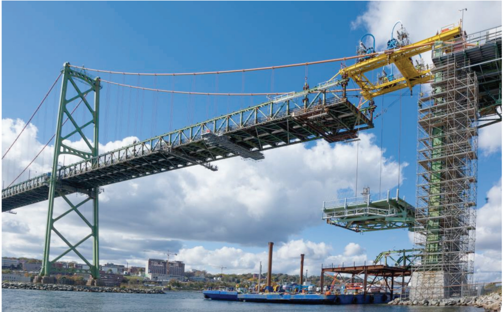
Figure 12. Raising of a new deck segment.
