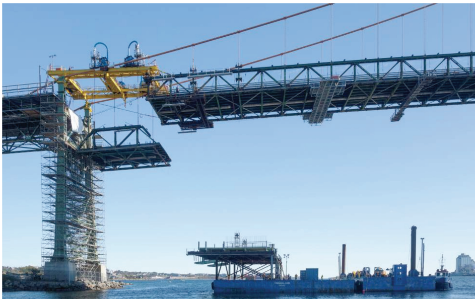
Figure 9. Lowering of the first existing deck segment in the Dartmouth side span.
