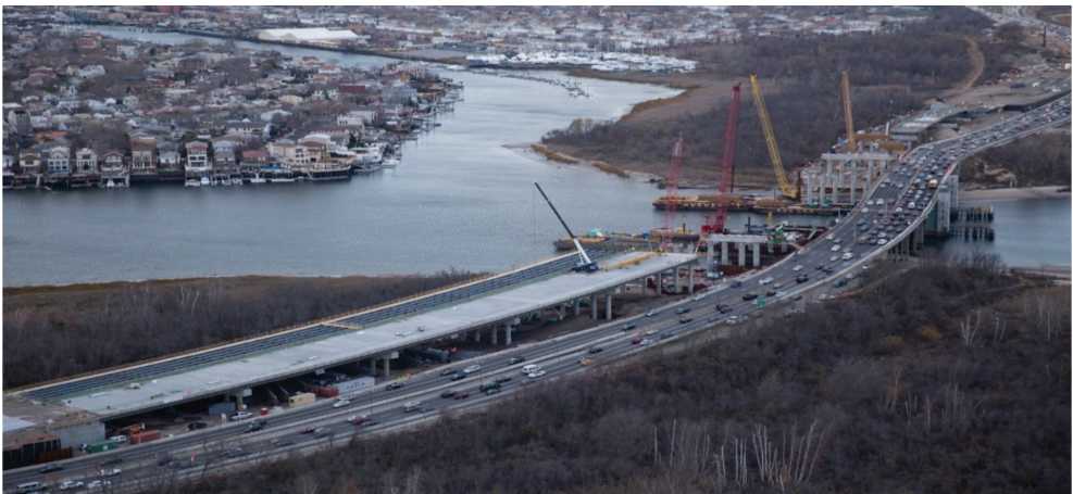
Figure 14. Replacement of Belt Parkway Bridge over Mill Basin—Stage 2 (December 2016).
