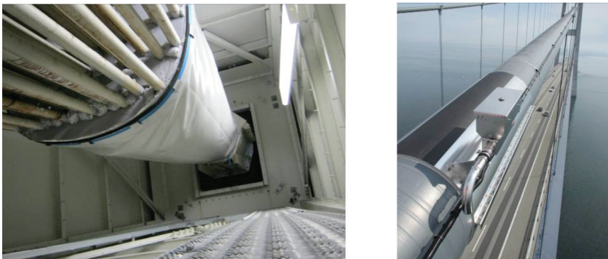
Figure 18. Enclosure of strands, Älvsborg Bridge and monitoring sleeve, Storebælt Bridge.
