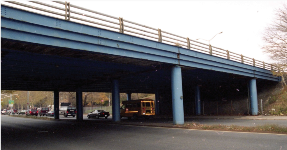
Figure 5. Original Belt Parkway Bridge over Rockaway Parkway (2005).
