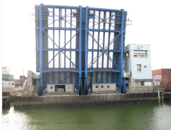
Figure 2. Metropolitan Avenue Bridge over English Kills, Brooklyn—typical view of low-lying bridge. Note proximity of machinery to water level.
