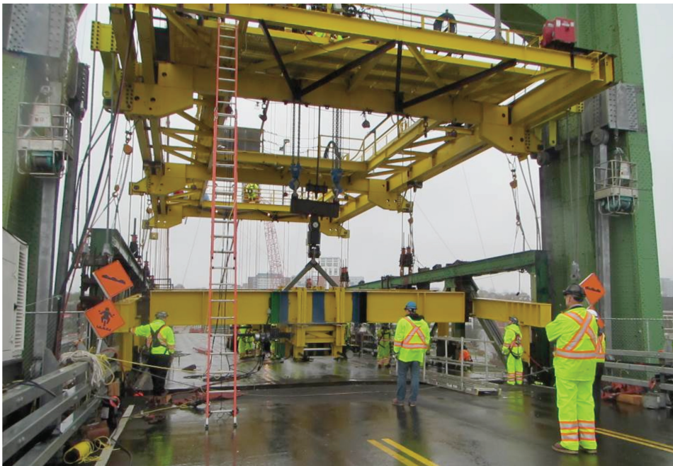
Figure 16. Halifax side span erection gantry equipped with a swivel and lifting frame.
