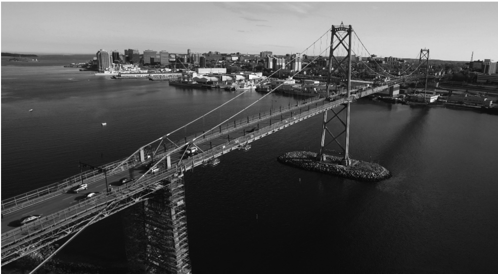
Figure 2. Aerial view of the Macdonald Bridge; part way through redecking.
