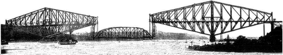
Figure 10. The span linked to the chains and raised clear of the scows, attempting the last hazardous operation in the construction of the bridge.
