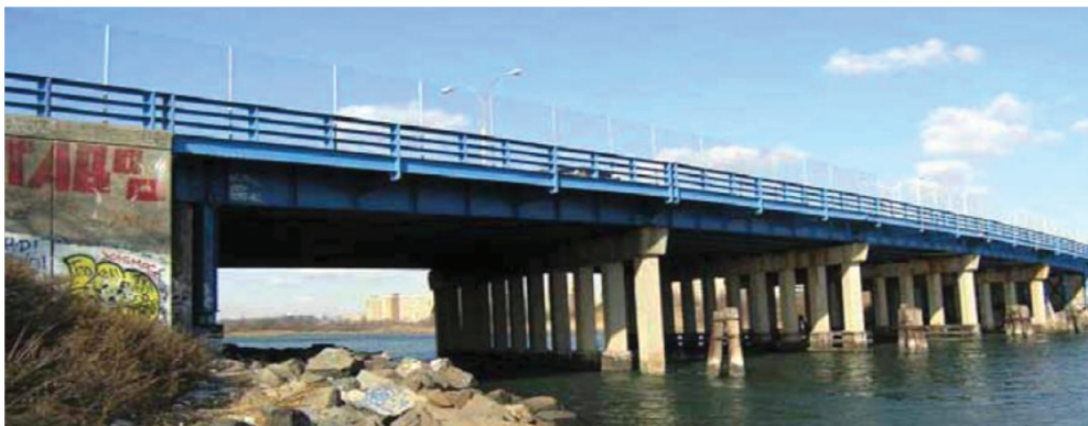
Figure 7. Original Belt Parkway Bridge over Fresh Creek Basin (2005).
