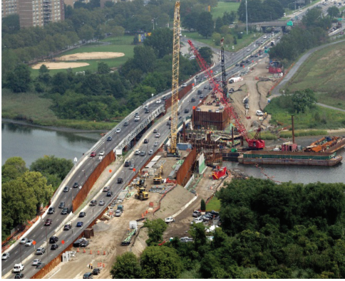
Figure 9. Belt Parkway Bridge over Fresh Creek Basin temporary bridge (2012).
