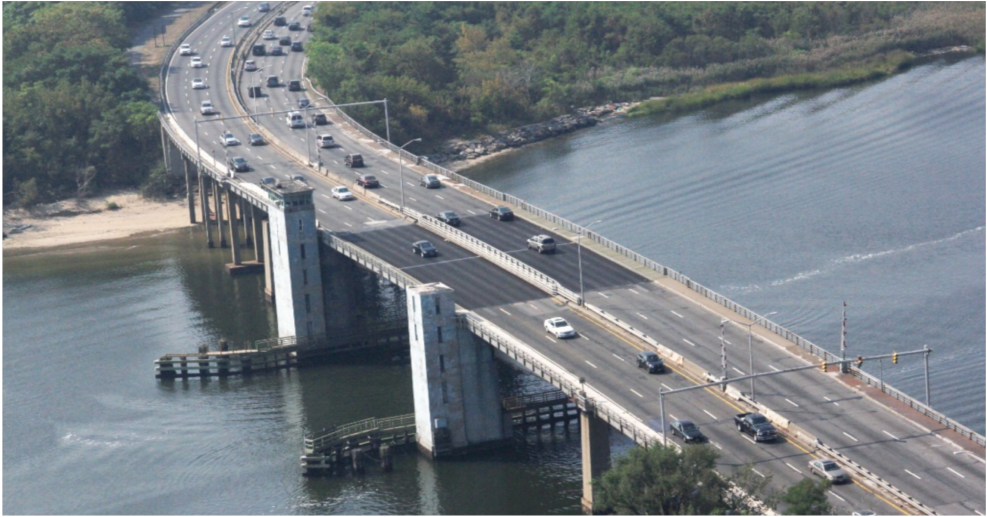
Figure 13. Original/existing Belt Parkway Bridge over Mill Basin (2012).
