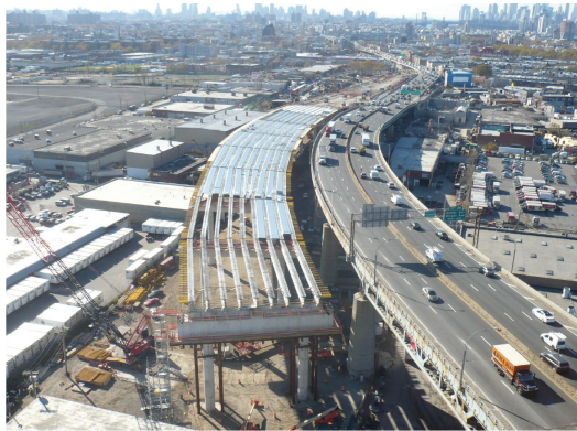
Figure 11. Aerial view of new Brooklyn Approaches with stay-in-place formwork being laid out over the prestressed girder superstructure.
