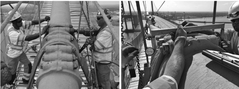
Figure 7. Cable band bolt tightening (left); Measuring bolt extension (right).
