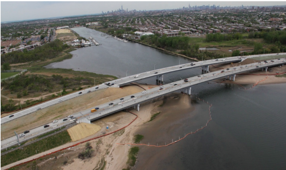
Figure 4. Replacement Belt Parkway Bridges over Paerdegat Basin (2013).
