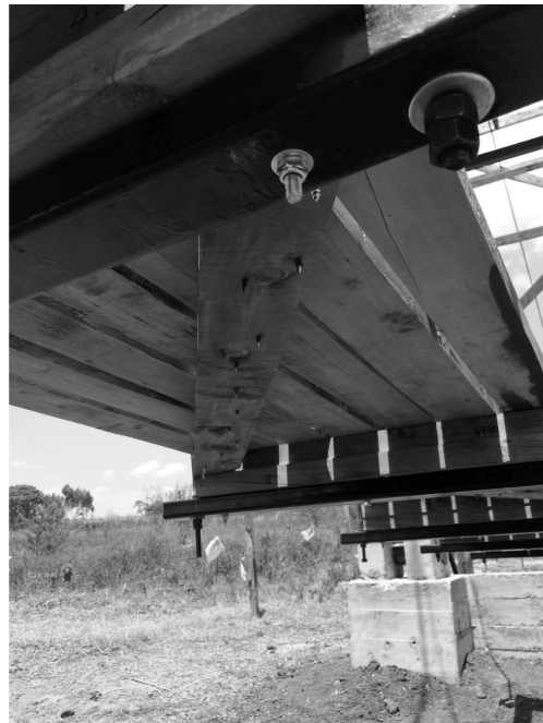
Figure 3. View of underside of deck showing crossbeams.
