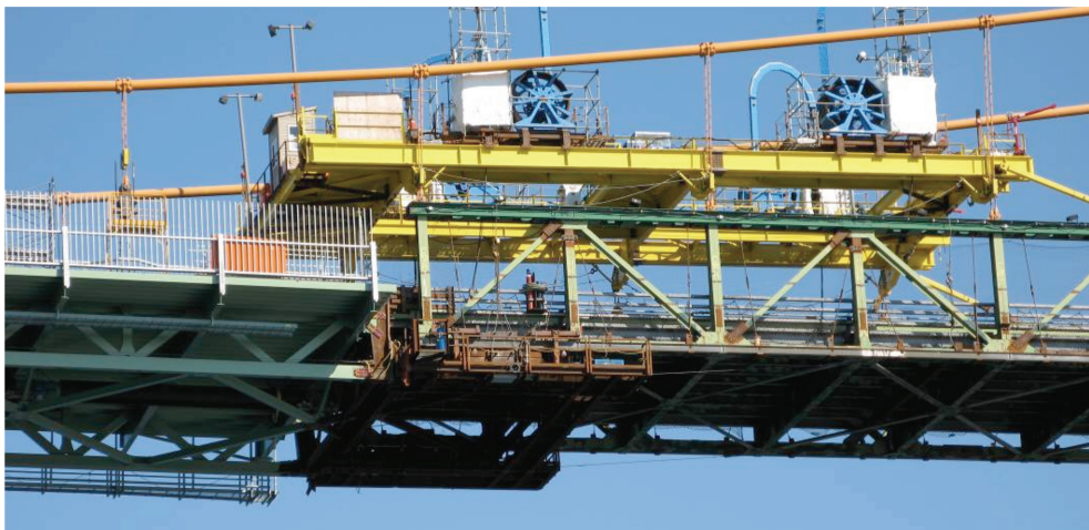
Figure 13. TDC in place between the new and existing segments (brown colored steel under the deck).
