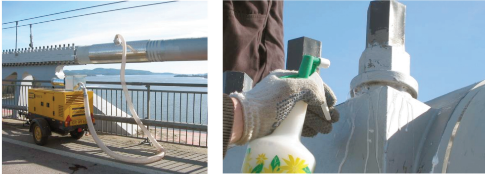
Figure 6. Flow test on Högakusten Bridge, air injection and soapy water test.
