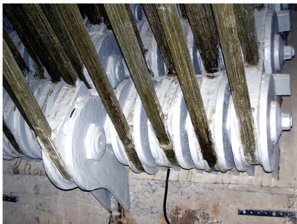
Figure 2. Anchorage of suspension cable built by the air-spinning method.
