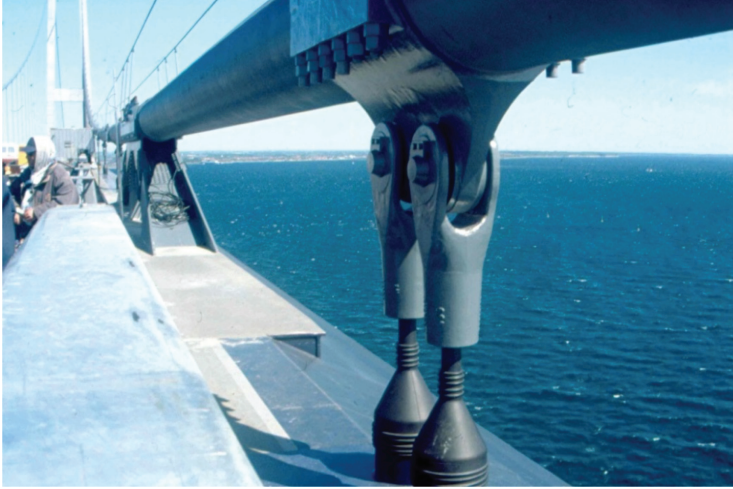
Figure 5. Cable, bands, suspenders and mid-span clamp at the Great Belt Bridge.
