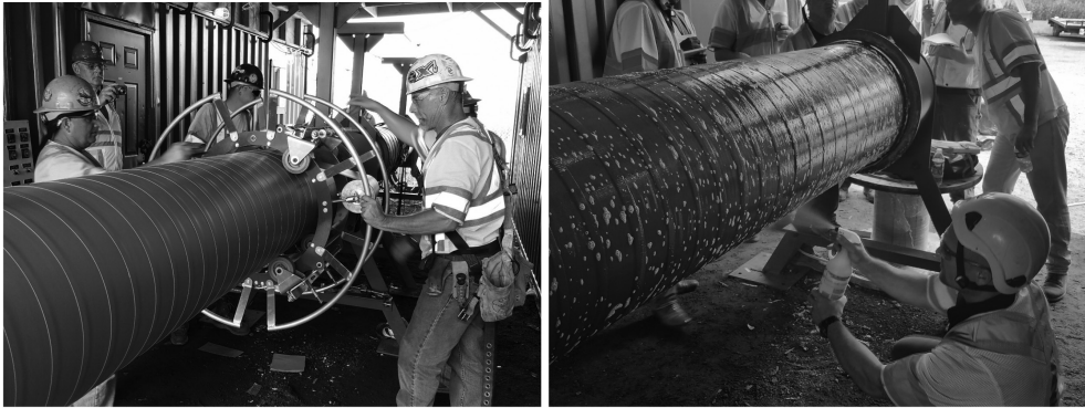
Figure 4. Trial wrapping on test rig (left); soapy water test on trial wrapping (right).
