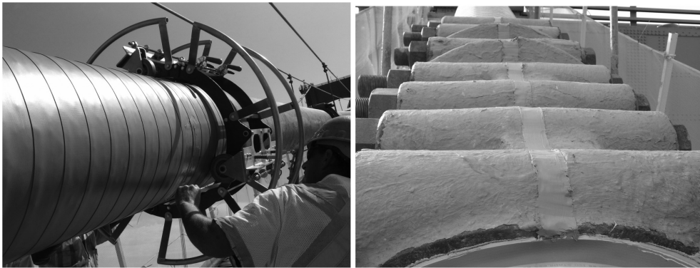
Figure 5. Skewmaster used to wrap cableguard on main cable (left); caulking on cable bands (right).
