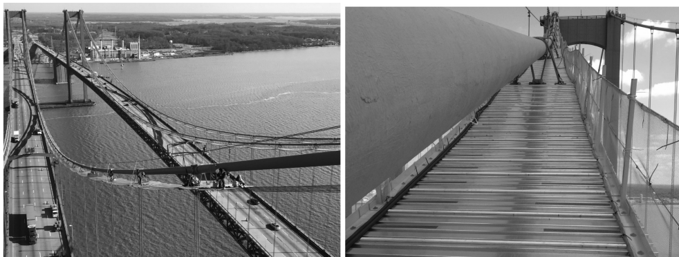
Figure 3. Cable access being erected (left); completed cable access platform (right).
