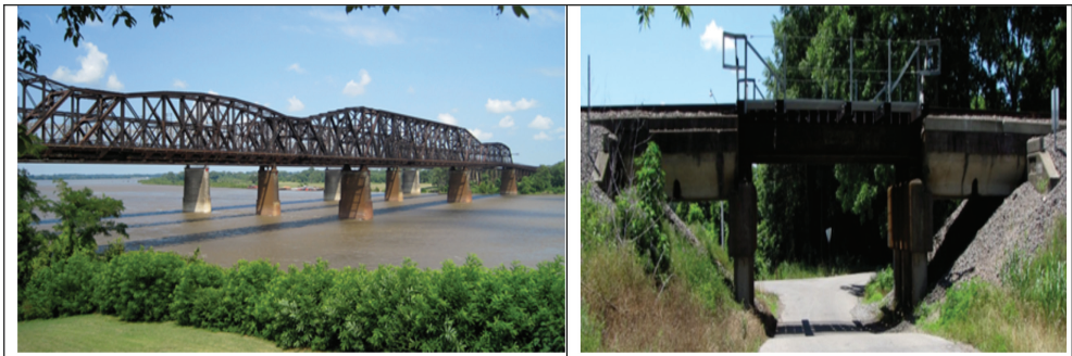
Figure 2. Harahan Bridge and Parkin Bridge.
