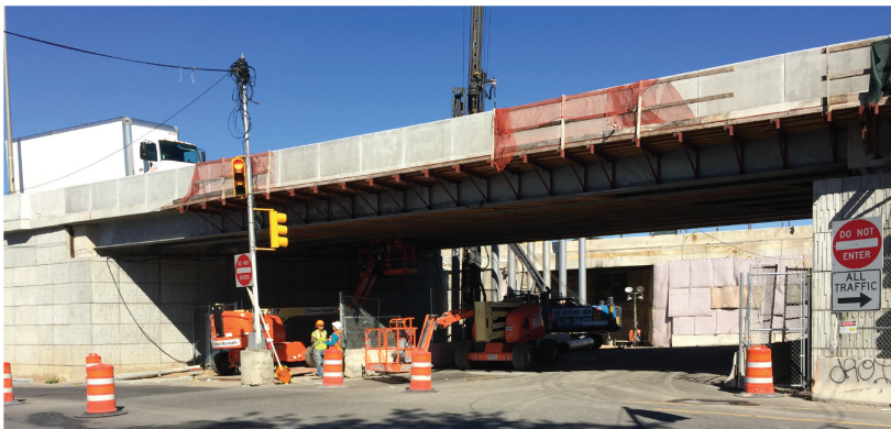
Figure 7. Vandervoort first stage completed and pile installation for the second stage in the back.
