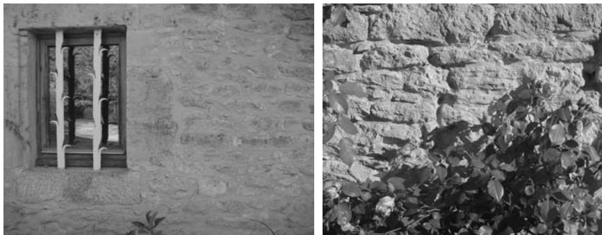
Figure 1.11 Improving the durability of the joints of a stone house with mortar joints (courtesy of Philippe Pattyn).
