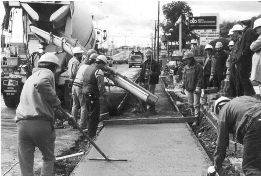
Figure 10.31a Placing the entrained-air concrete.
