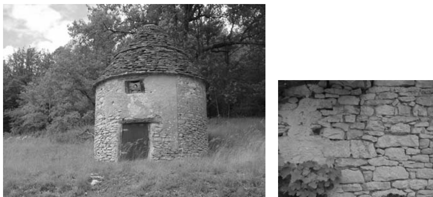
Figure 1.8 Improving the tightness of a borie with clay joints (courtesy of Philippe Pattyn).
