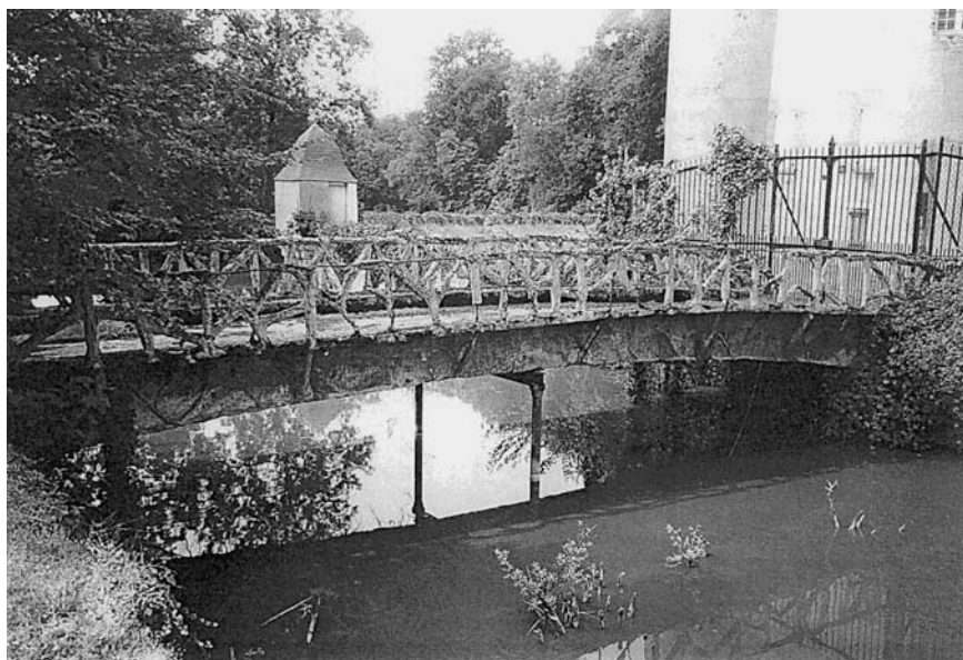
Figure 2.18 The first bridge in reinforced concrete: the Chazelet bridge by Monier (courtesy of J.-L. Bosc).
