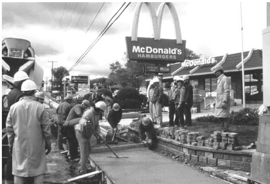
Figure 10.31b Placing the non-air entrained concrete.
