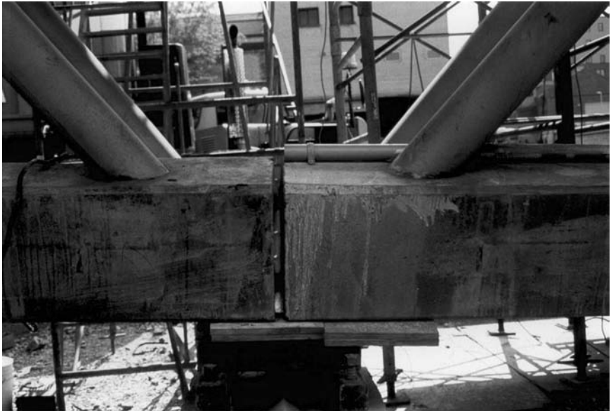
Figure 10.46 Assembling two prefabricated elements (dry joint).
