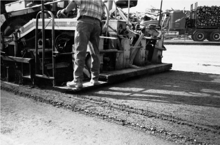
Figure 10.34 Mixing and placing a roller compacted high-performance concrete at the Domtar pulp and paper plant in Windsor Mills near Sherbrooke.
