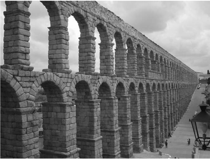
Figure 2.3 Segovia aqueduct in Spain.
