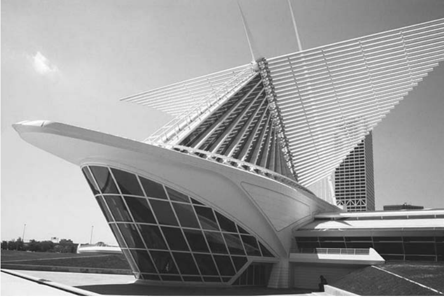
Figure 1.15 Milwaukee Art Museum by Calatrava (courtesy of the Milwaukee Art Museum).
