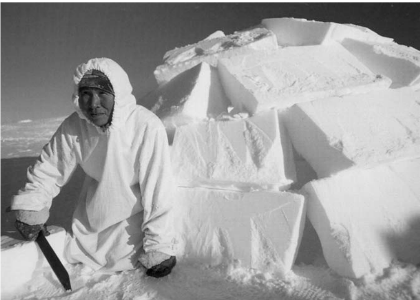
Figure 1.7 An igloo is built with blocks of compacted snow, not with ice blocks. Photo by Heiko Wittenborn.
