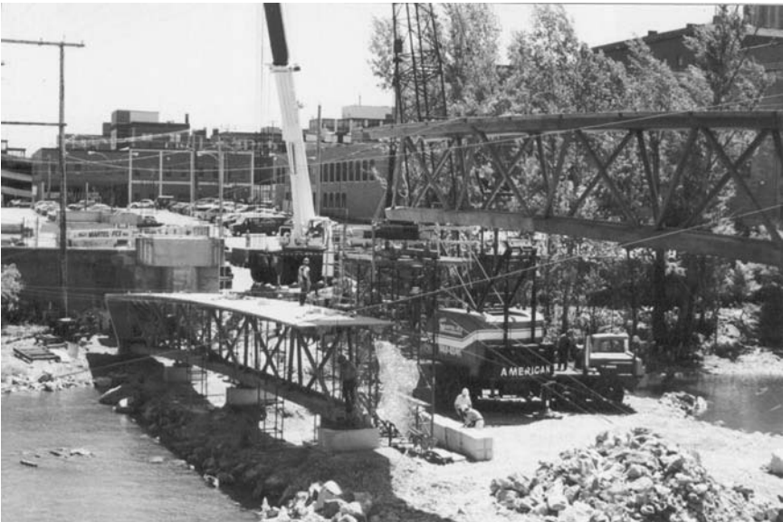
Figure 10.47 Assembling the two halves of the bridge.
