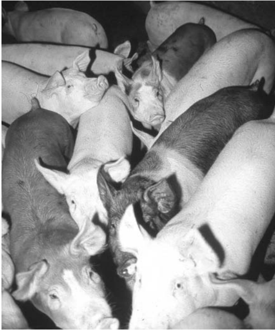
Figure 10.32 Use of high-performance concrete floor in a piglet farm.
