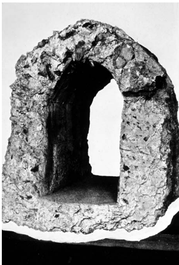
Figure 2.5 Section of a Roman aqueduct from Köln (Germany) (courtesy of the Portland Cement Association).
