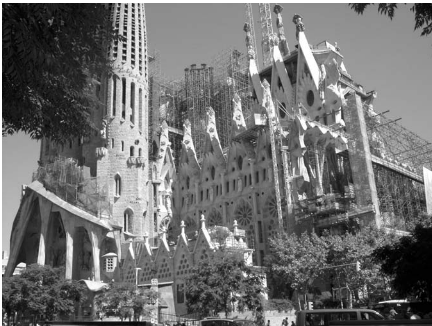
Figure 1.14 The use of high-performance concrete in the Sagrada Familia (photo by Isabelle Aitcin).
