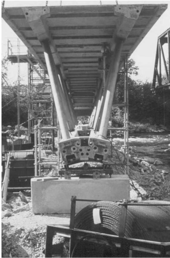
Figure 10.45 Assembling the northern part of the bridge.
