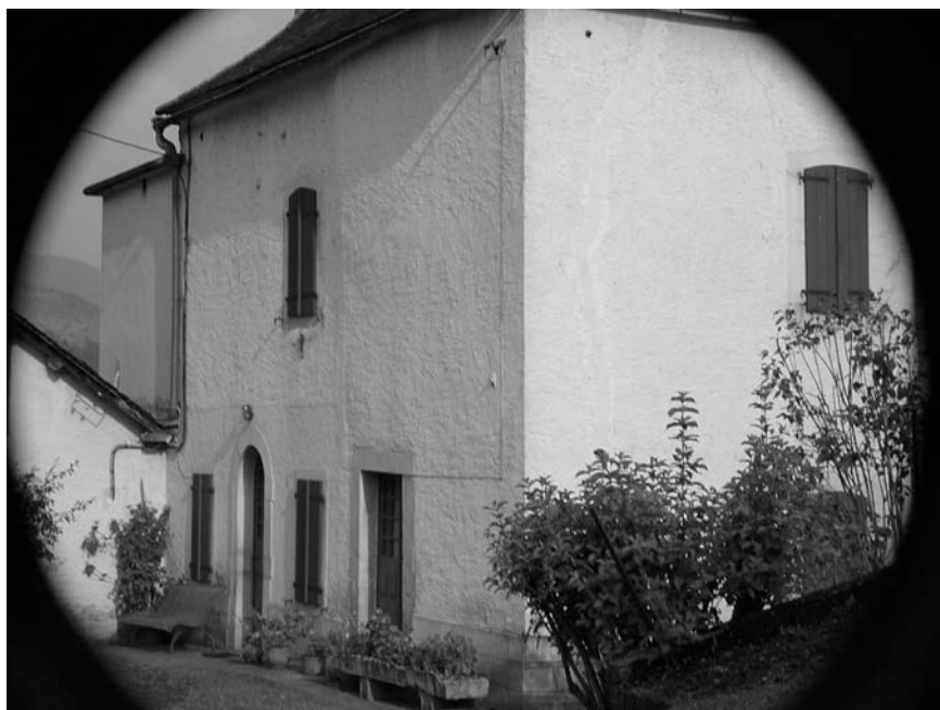
Figure 1.9 The Jauregi farmhouse built by one of my ancestors before 1365 in the Basque province of Xuberoa in France. Initially the house was built with pebbles of a nearby mountain stream jointed with a lime mortar. The lime-Portland cement roughcast was added more recently. The house resisted a nearby strong earthquake in the Pyrenees, three patched cracks are still visible.
