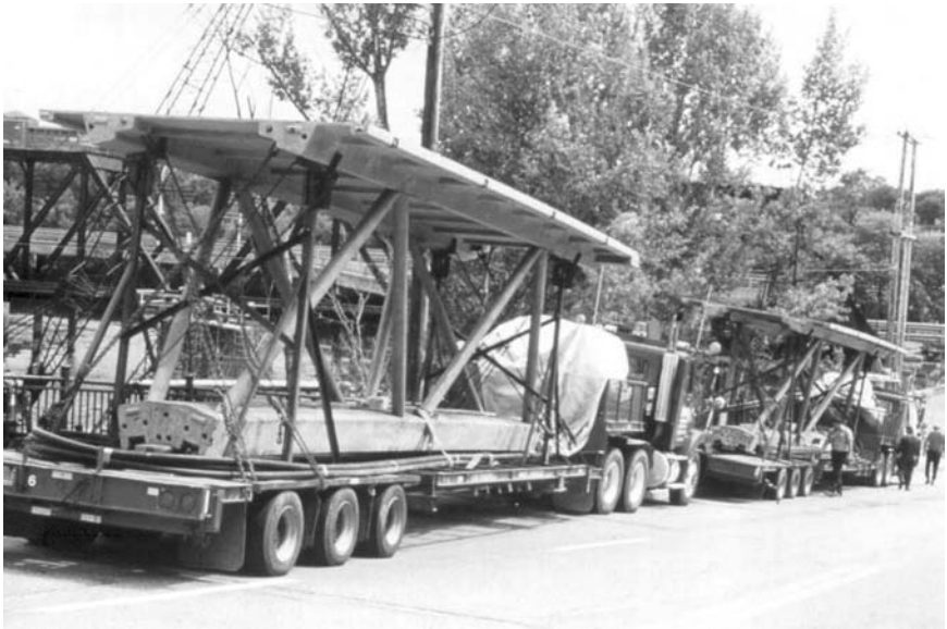
Figure 10.44 Transportation of the prefabricated elements.
