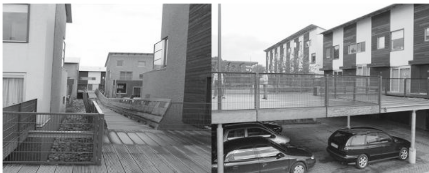
Fig. 2 Example of adapted building use
