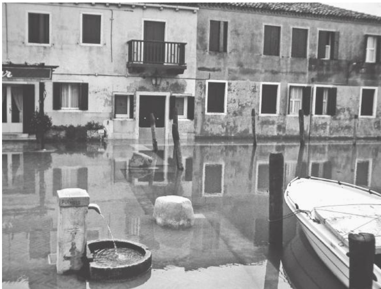
FIGURE 4.23. Water damage. The frequent flooding of Venice, known as acqua alta , has become a serious environmental problem as rising waters are taking their toll on the foundations of buildings and monuments. In this photo, water damage is quite visible on the faces of these buildings.
