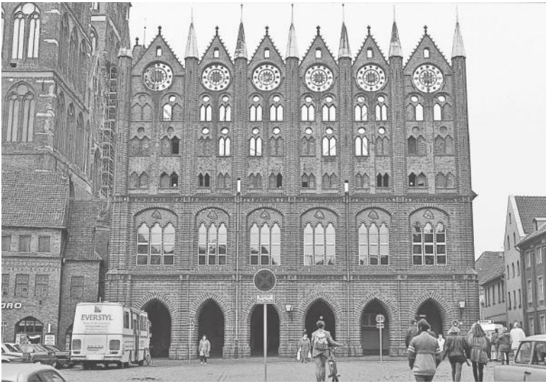
FIGURE 8.13. Rathaus. Straslund's mid-13th-century town hall is a solid example of the characteristic medieval decorated brickwork of northern Germany. The high façade features spire-tipped turrets and huge holes to lessen wind resistance. Coats of arms are embedded in the brickwork.
