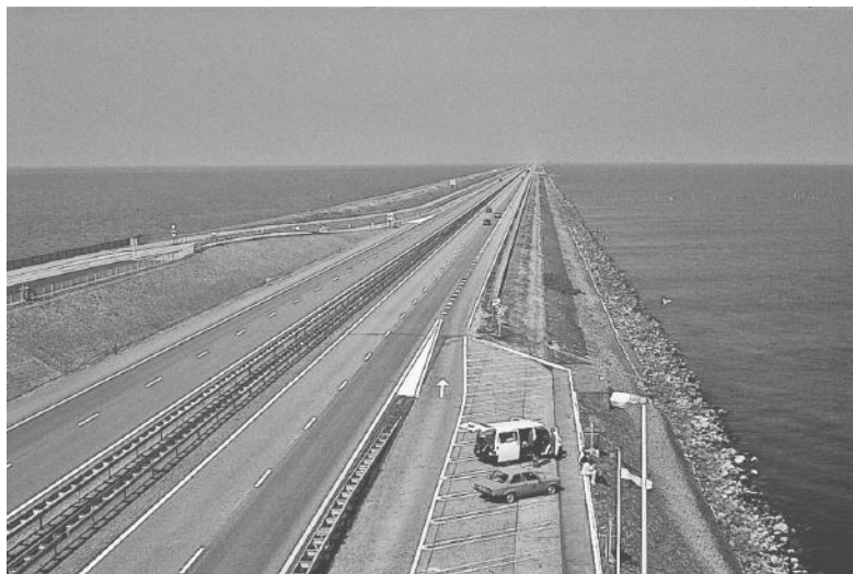
FIGURE 4.4. Afsluitdijk. In 1932 the Dutch completed this 31-kilometer-long dike to isolate the Zuiderzee, a large inland arm of seawater, from the North Sea. Freshwater soon replaced salt water in the old Zee, seen to the right of the dike in this photo. Large areas (polders) were reclaimed for agriculture in a series of projects, and the remainder was preserved as a freshwater lake, now known as the IJsselmeer.
