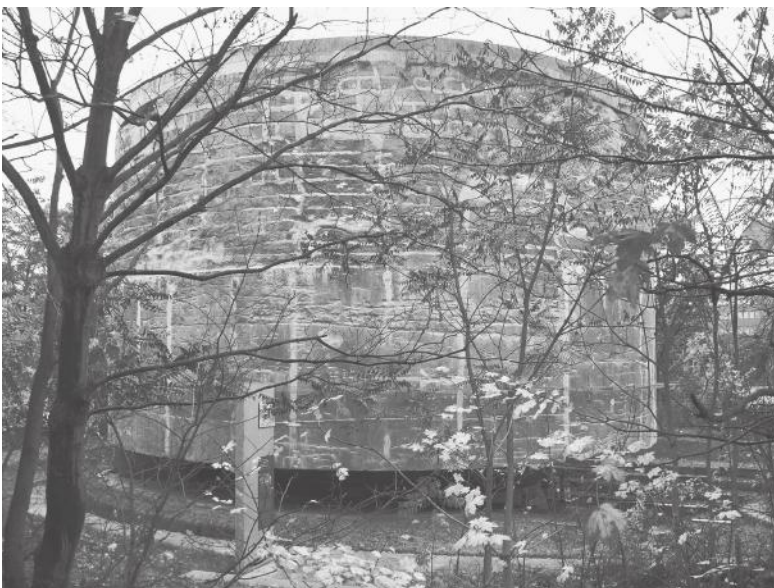
FIGURE 9.6. Footing. Almost nothing remains of Hitler's grandiose designs for postwar Berlin. One of the few pieces remaining is the giant concrete cylinder, which was poured as a test footing for a planned triumphal arch, so enormous that it would dwarf Paris's Arc de Triomphe and have sufficient surface space to carry the names of millions of German soldiers who gave their lives in sacrifice. Today it sits quietly on a vacant lot on the south side of Berlin.
