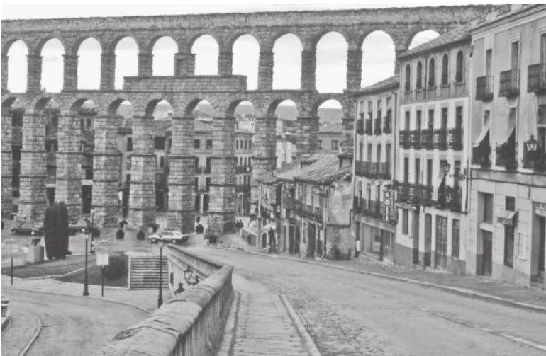
FIGURE 8.7. Public works. Built in the first century CE, the aqueduct at Segovia brought water from the River Frio to the Roman settlement and military camp at Segovia. Nearly 30 meters tall at its highest point, the double-tiered arched construction carried water until late in the 19th century.
