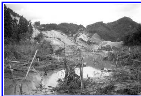
(e) Aratozawa dam landslide
