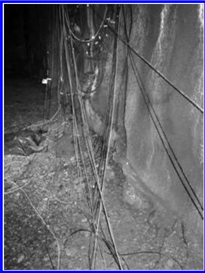
Slot tunnel showing soil movement after Test #3
