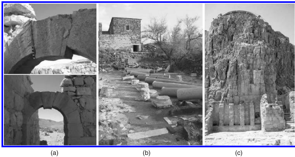
Figure 16.1 Analyzed field case studies: (a) key stone displacement in a Roman arch, (b) toppling of a series of columns in a Byzantine church. (c) The highly fractured rock slope at the North face of Masada – King Herod's palace.
