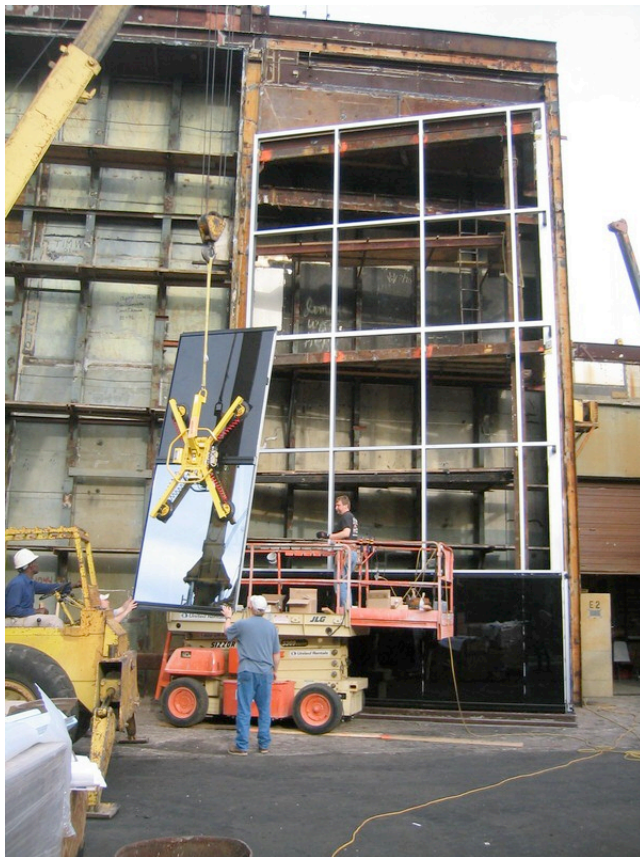
Figure 8: New curtain wall units attached to the laboratory mock-up frame.
