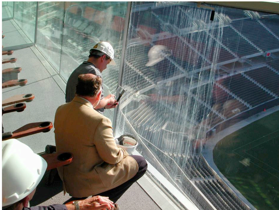
Figure 3 - View of streaking at suite vision lite.
