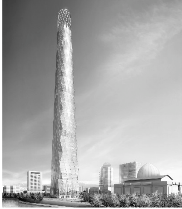
Figure 2: Lotte Super Tower (Courtesy of SOM, Chicago)
