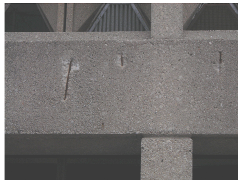
Figure 3. Concrete spalls
