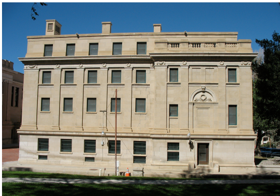
Figure 1 Building Front Elevation
