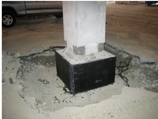
Figure 4 - CFRP Wrap around New Rectangular Concrete Pedestal.
