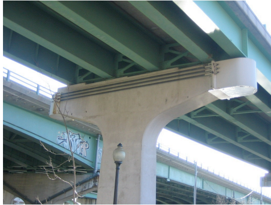
Figure 1- Strengthening of Bridge Pier Cross Beam by High Tensile Bar Post-Tensioning
