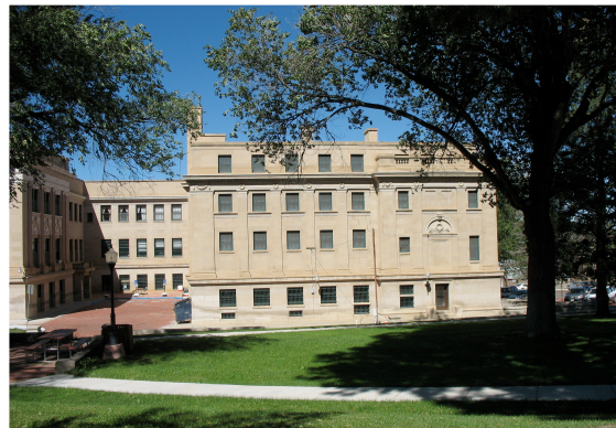
Figure 2 Building w/surround buildings
