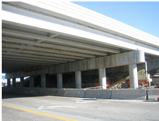
Figure 2- Reconstruction of New Concrete Pier on Existing Foundation
