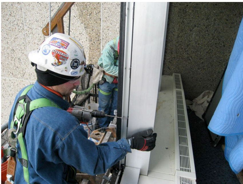
Figure 13: Fastening a new curtain wall unit into existing aluminum mullion.
