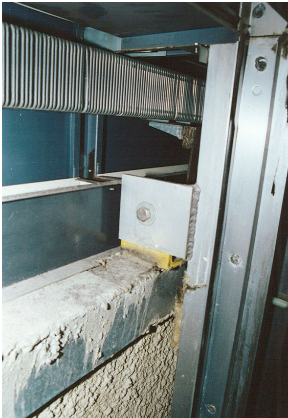
Figure 6: Existing curtain wall framing connection.
