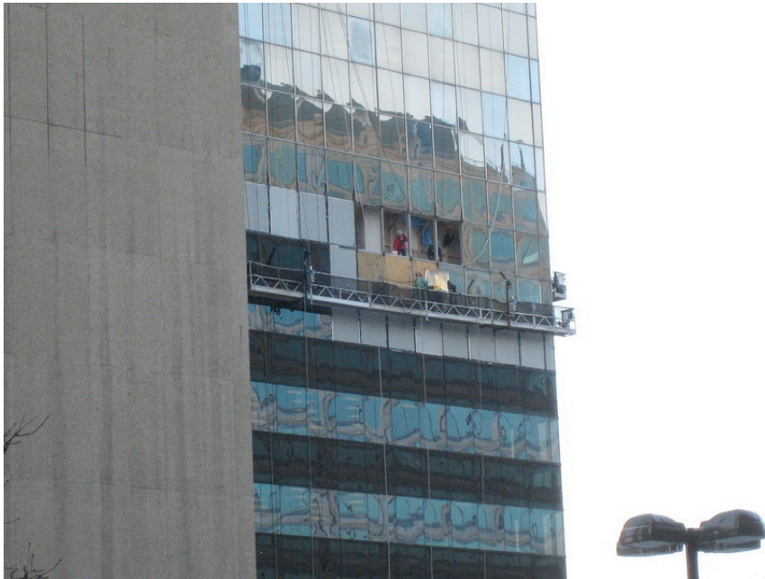
Figure 14: Installing temporary panels at the end of a work day.
