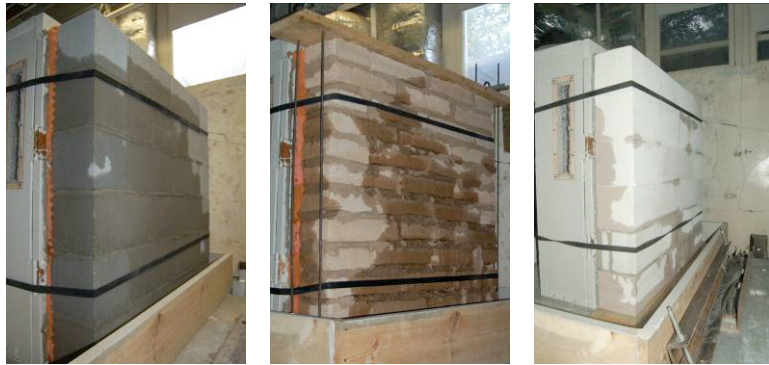
Figure 2. Photographs of the wall specimens at the end of water penetration tests
