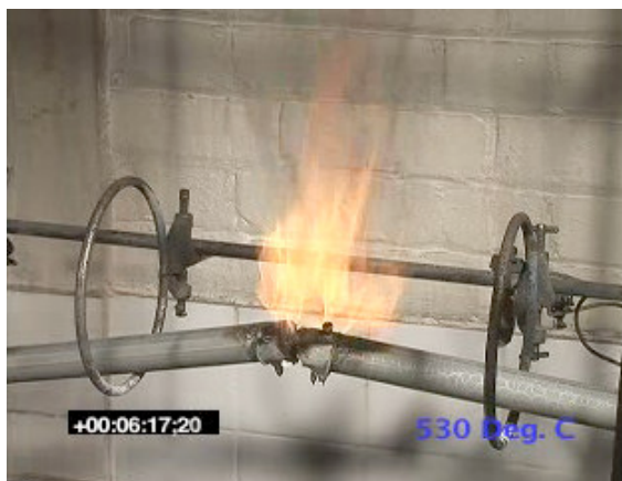
Figure 15 - Complete failure of Die-Cast Coupling at 530°C, with non-plenum cabling flaming.
