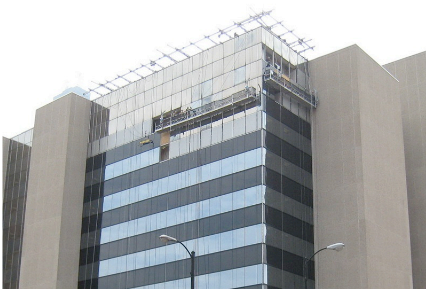
Figure 11: Using the monorail system to "trolley" curtain wall units into position.
