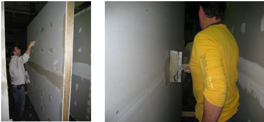
Figure 4. Application of joint compound over the horizontal drywall joint
