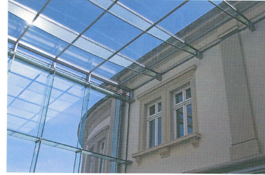
Figure 6.a Glass beams with tension rods [35]
