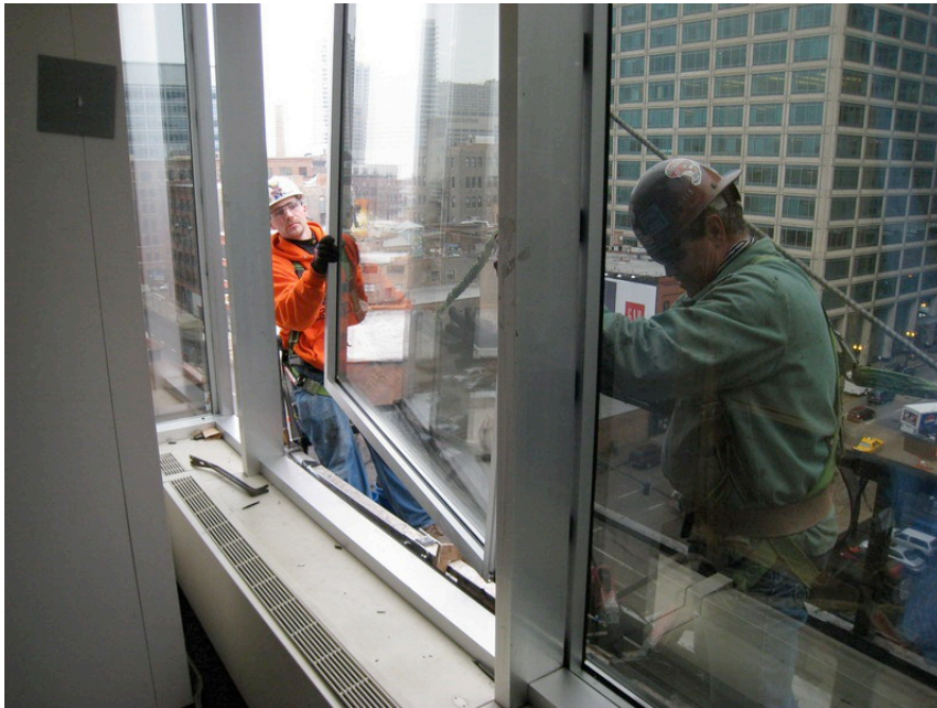
Figure 12: Moving a new curtain wall unit into position.
