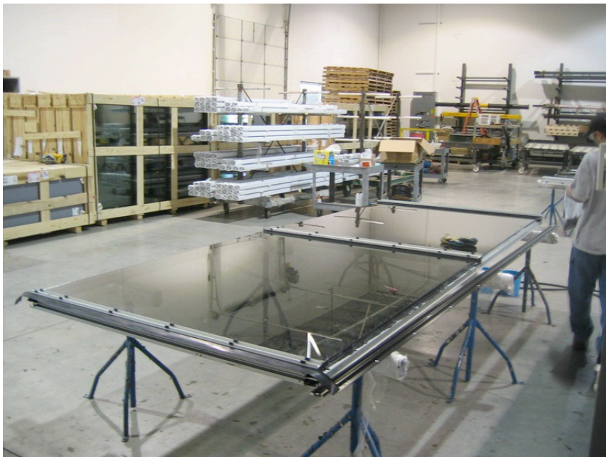
Figure 10: Curtain wall unit shop fabrication.
