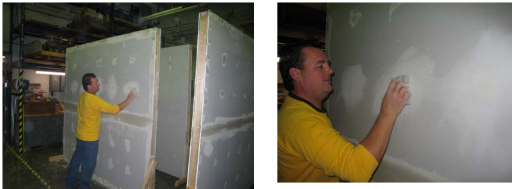
Figure 5. Sanding the finishing compound after being sufficiently dry
