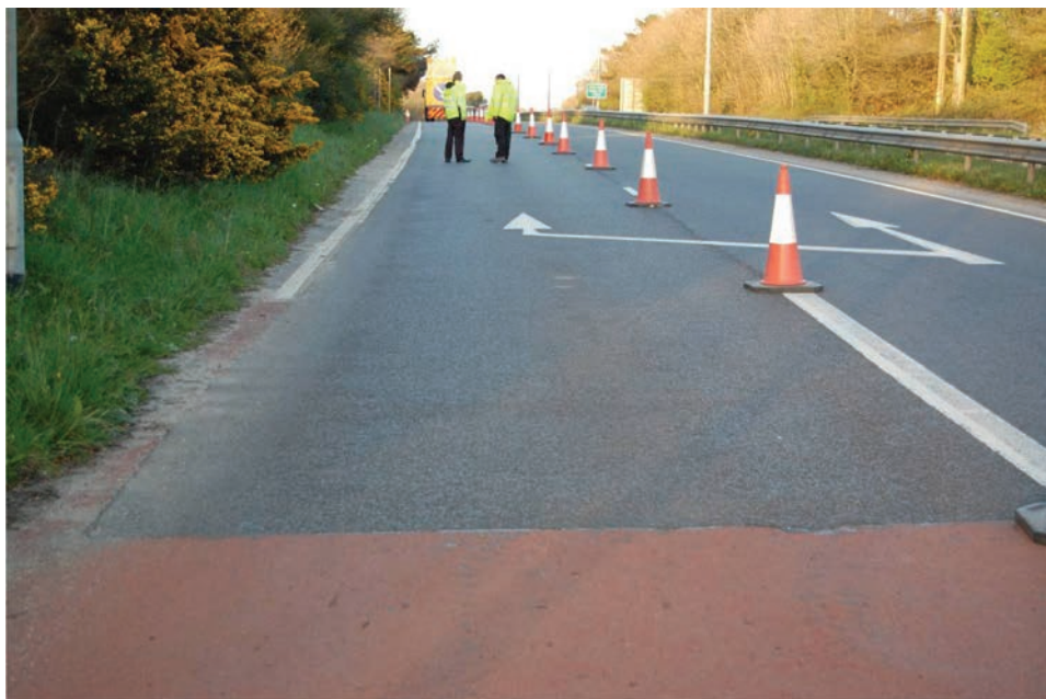
Figure 3. Epoxy asphalt trial section after 12 months trafficking (2013).
