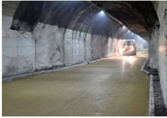
Figure 5. Clear asphalt concrete compaction in the road tunnel.
