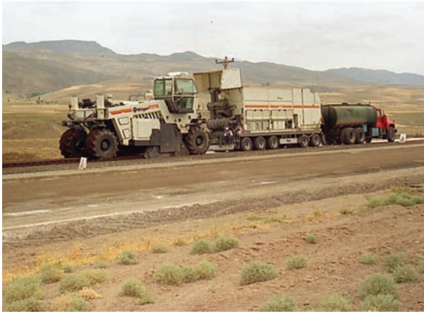
Figure 7. Train of cold-in-place recycling machineries.
