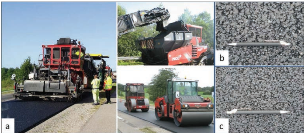
Figure 1. Field section activities (a), SMA 8 (b), SMA 6 (c).
