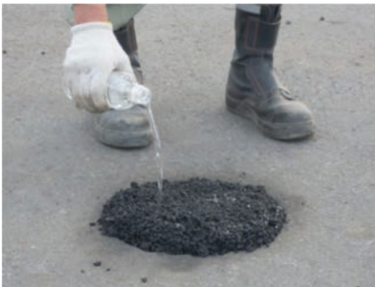
Photo 3. Water spraying.
