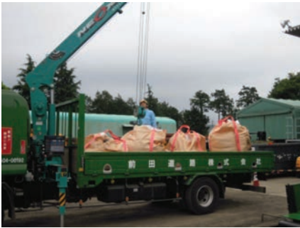
Photo 9. Stockpile materials bagged in flexible container.
