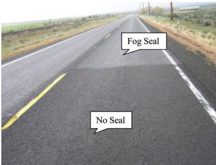
Figure 3. Visual comparison of sealed with non-sealed section at the US 395 test site.
