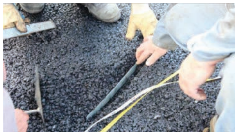
Figure 4. Implementation of a flat steel bar in the asphalt.
