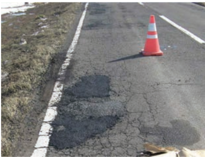
Photo 5. Restoration after earthquake.
