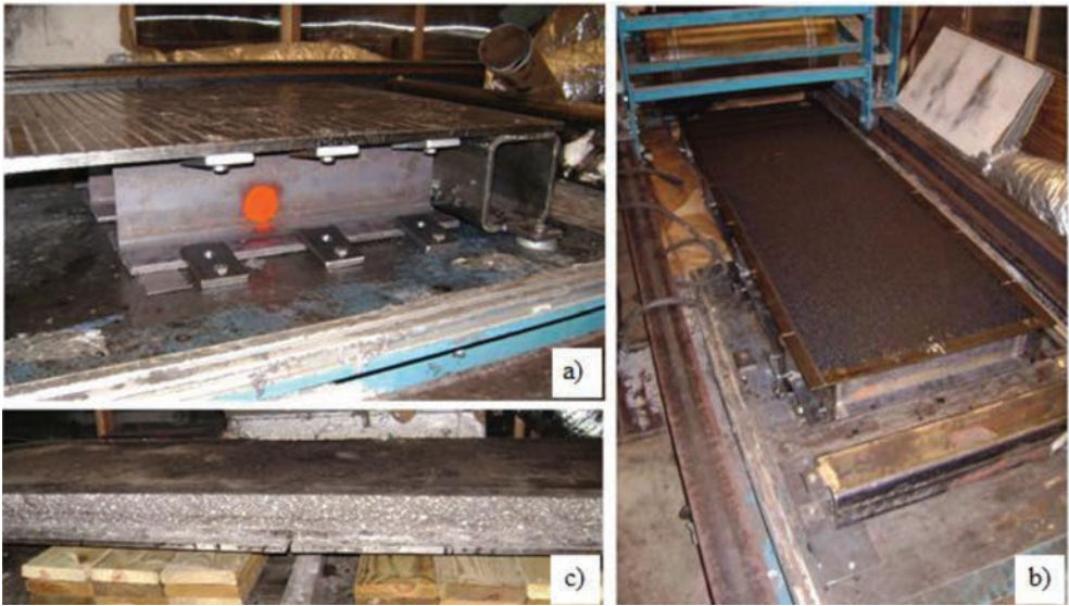
Figure 3. a) Close-up of steel plates bolted to supports, b) RCT and compaction frame during compaction, and c) Final layered system with smoothed surface.
