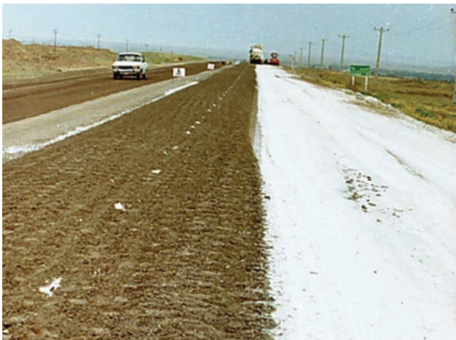
Figure 8. Base layer recycling and compaction.
