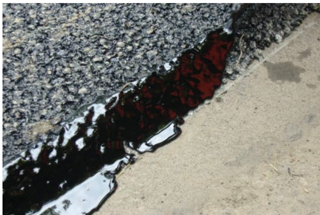
Figure 7. Chamfered joint.
