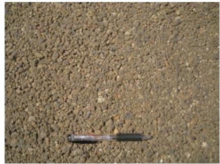
Photo 10. Application to natural stone pavement.
