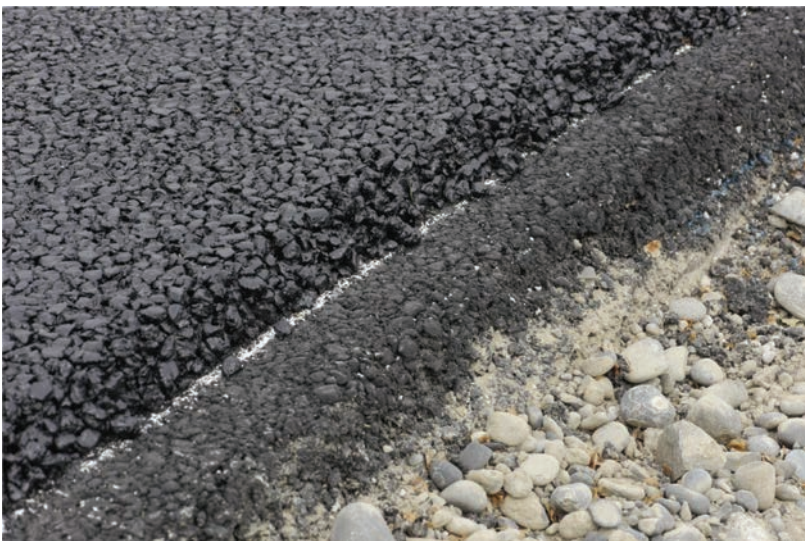
Figure 1. Trial pavement structure. Upper most layer is the final OGPA surfacing.
