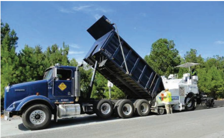
Figure 2. CCPR mixture paving.
